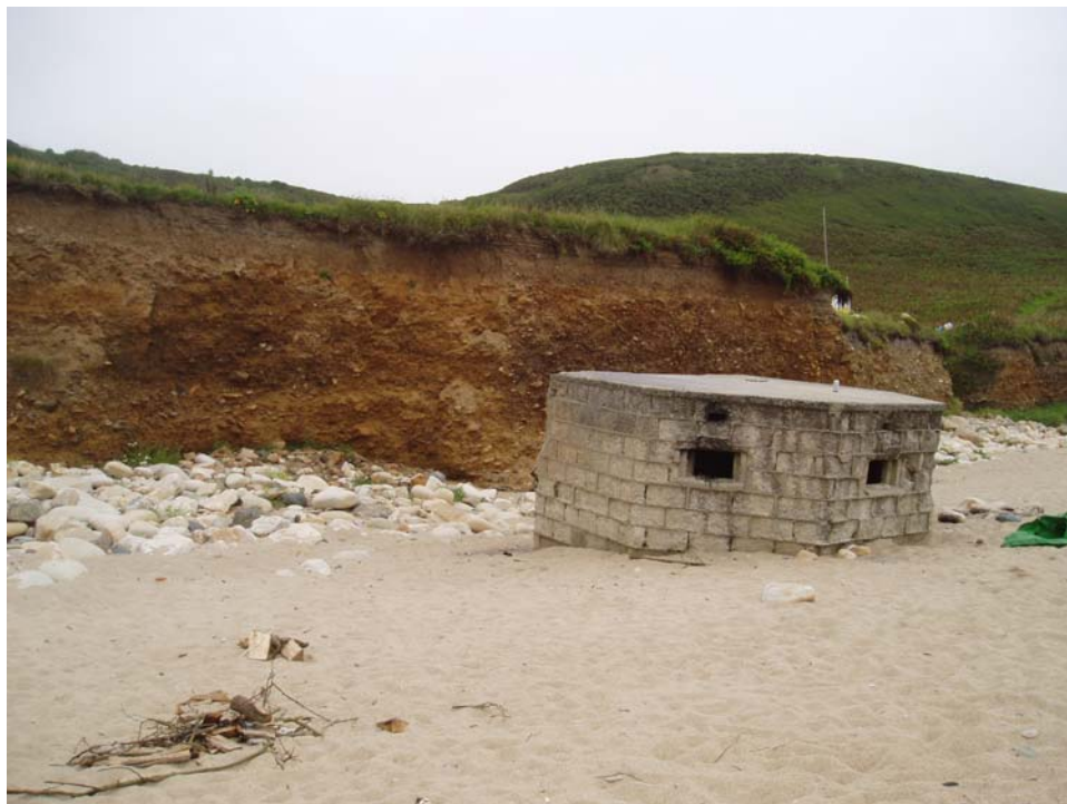
Figure 37: Prah Sands pillbox originally erected in dunes, now on the beach as the result of coastal erosion
