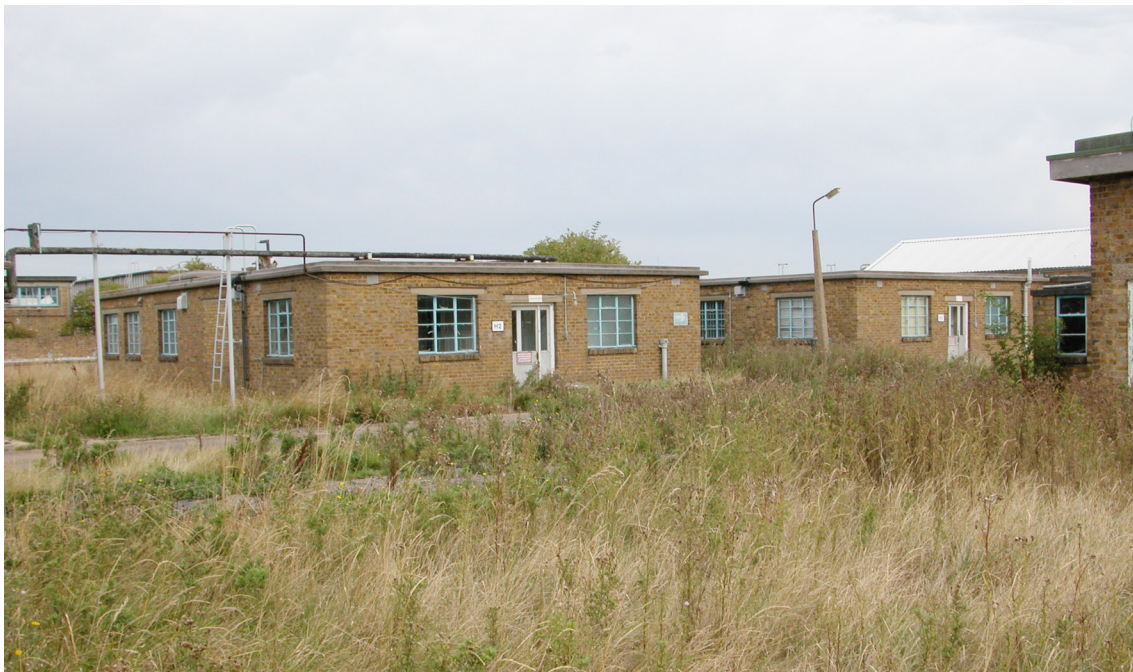
Figure 47: Late 1940s office buildings, to the left H2, was 40, and to the right H3, was 49. (c) English Heritage
