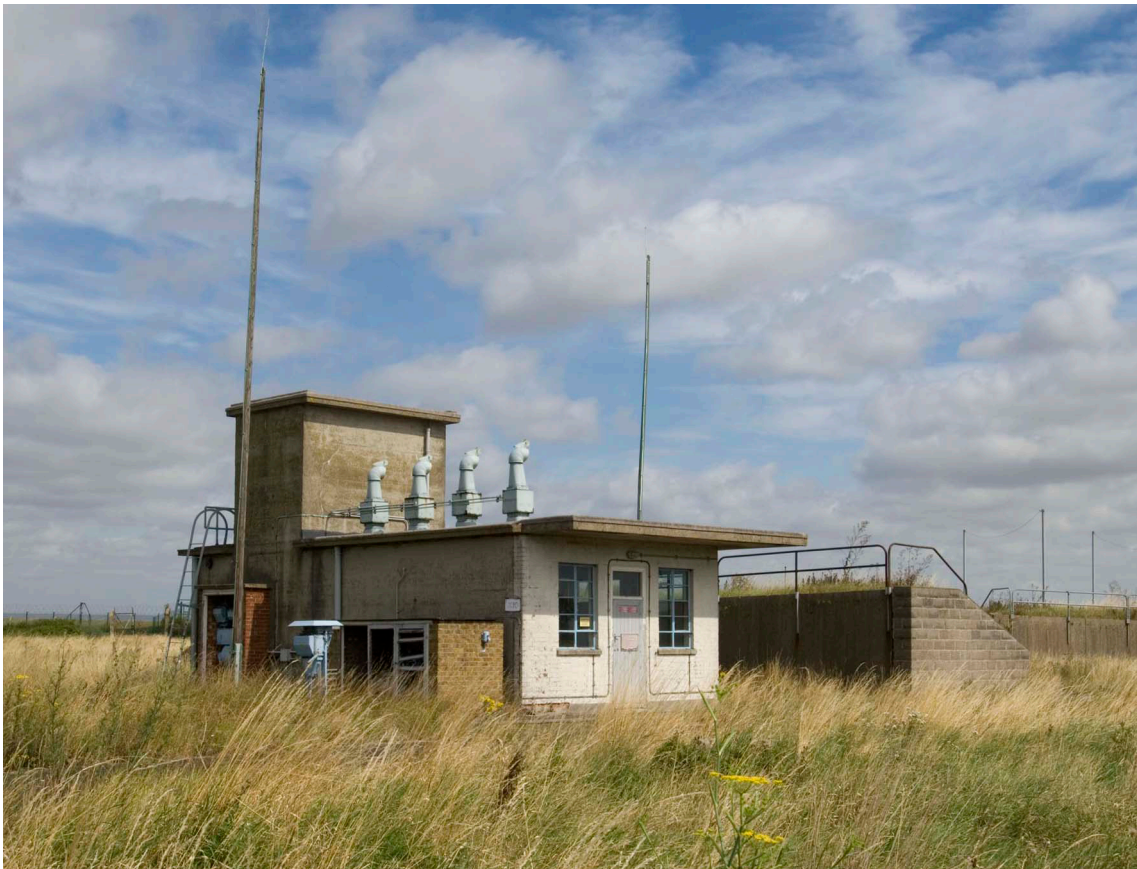
Figure 40: Casting Shop X10, was 56, built about 1953, with a rear reinforced concrete wall and to the right is later breeze block and earthwork traverse. (c) English Heritage DP035931
