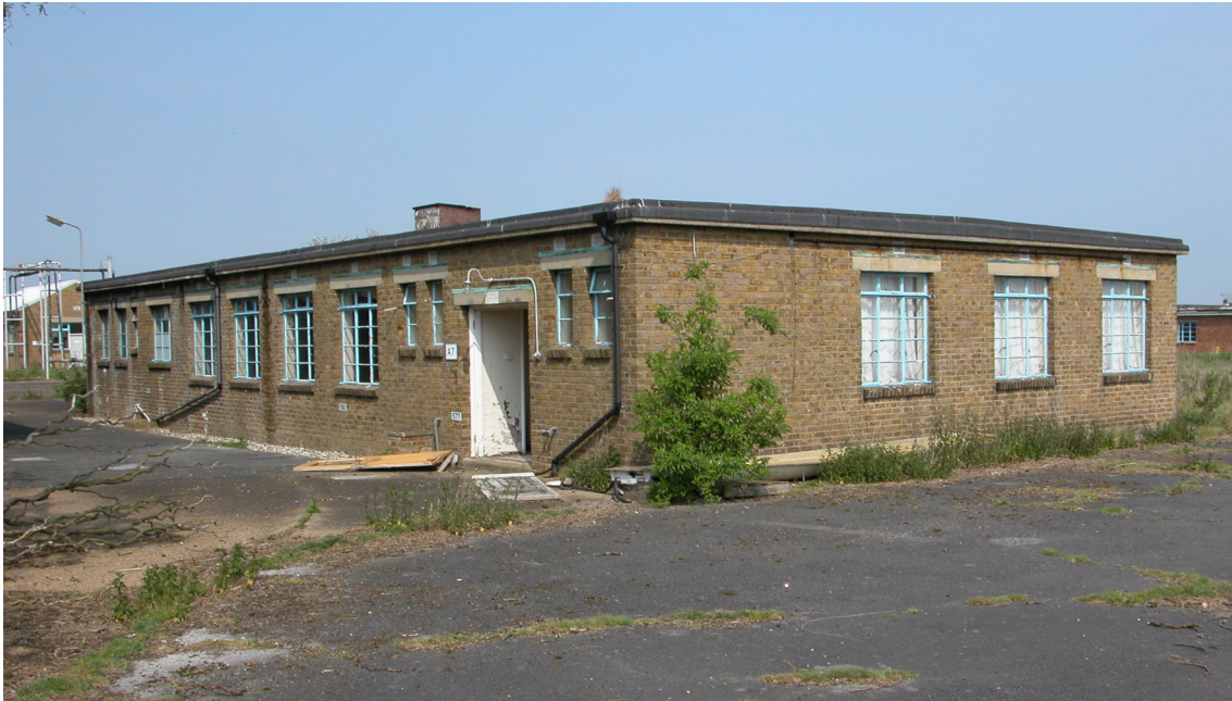
Figure 46: Canteen A7, was 24, is typical of buildings of this date with brick walls, a flat concrete roof, metal Crittall windows with concrete lintels and sloping brick sills. (c) English Heritage
