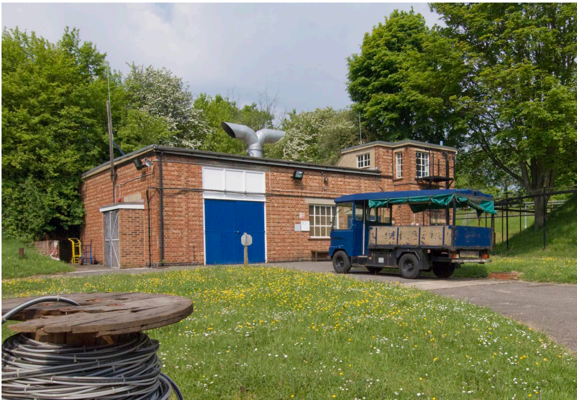
Figure 4: Fort Halstead, Kent, Detonation Chamber purpose built in 1949 for the High Explosives Research team. Smaller laboratory sized experiments were carried out here before the larger scale trials at Foulness. (c) English Heritage DP060573
