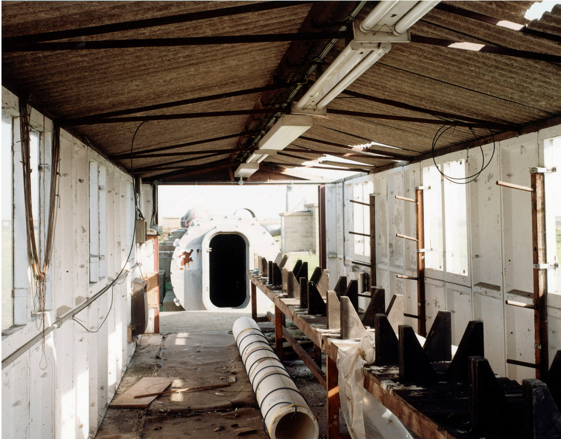
Figure 16: Charge Assembly Building I/SF46, this view shows the polystyrene former around which a length of detonating cord was wrapped. Once assembled the charge was suspended in the tunnel and the bulkhead doors sealed. (c) English Heritage BB99/16000
