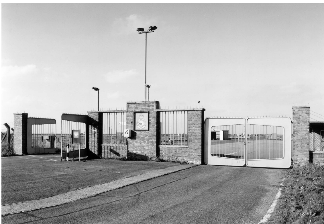
Figure 9: The main entrance to the AWRE area from Foulness Road in September 1999. (c) English Heritage BB99/15987
