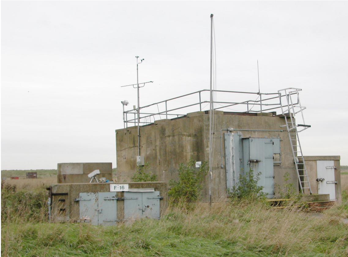
Figure 14: Fire Control and Instrumentation Building F6 and Cable Terminal Building F16. (c) English Heritage
