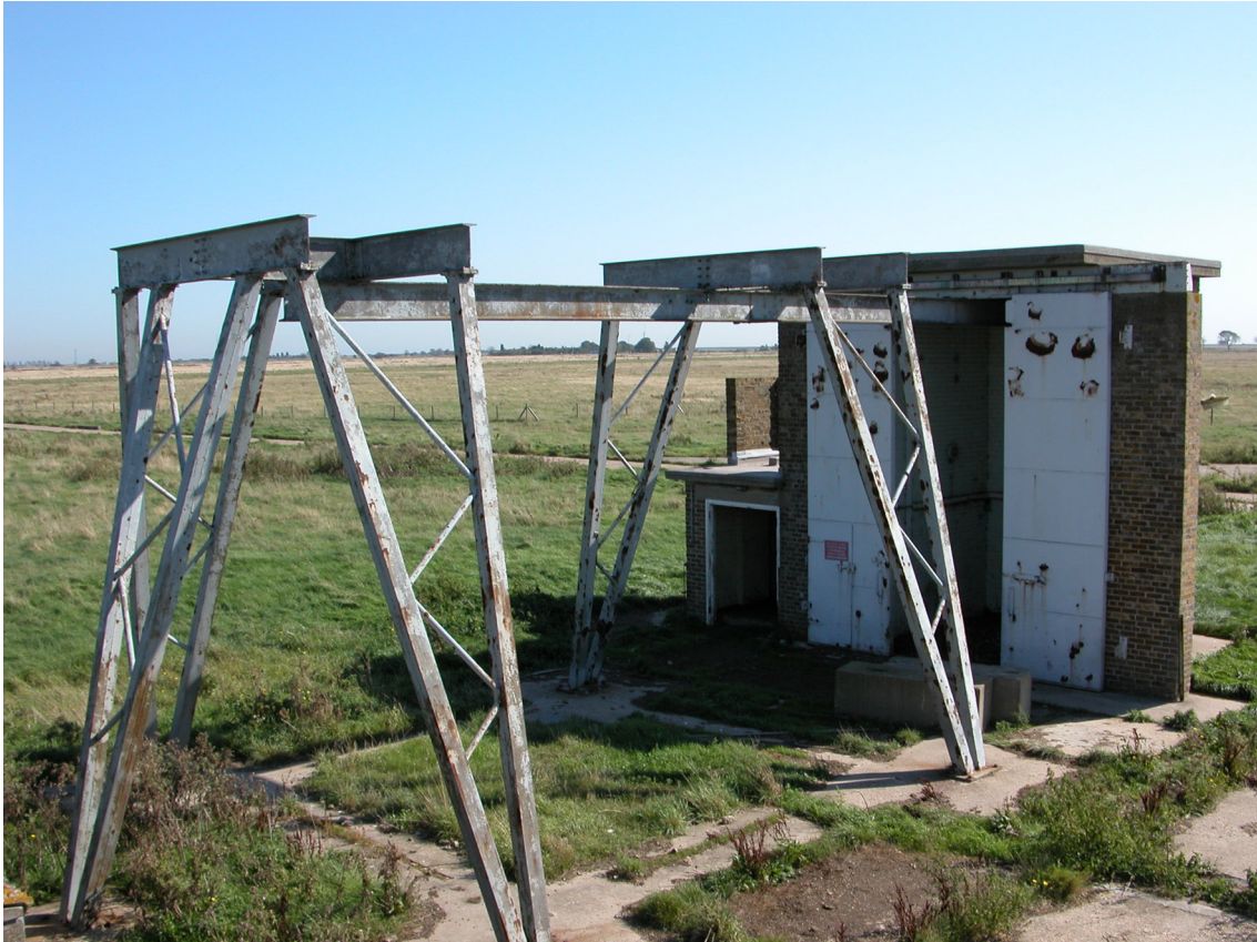
Figure 18: This building 110 was last used as a Fork Lift Garage, but was probably constructed for a more specialised function. (C) English Heritage
