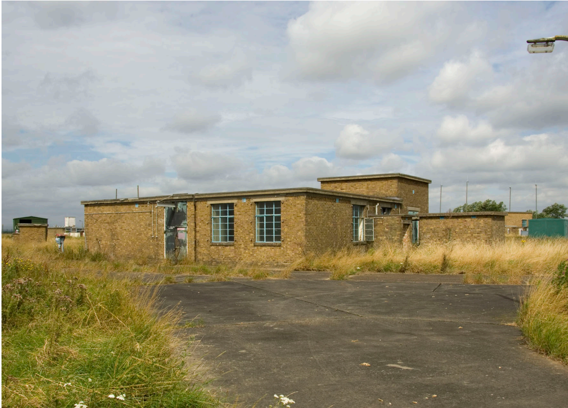
Figure 38 Explosives Preparation, Casting and Pressing X23, was 29, to the rear is the raised roof of the room that housed the 200 ton press. (c) English Heritage DP035935
