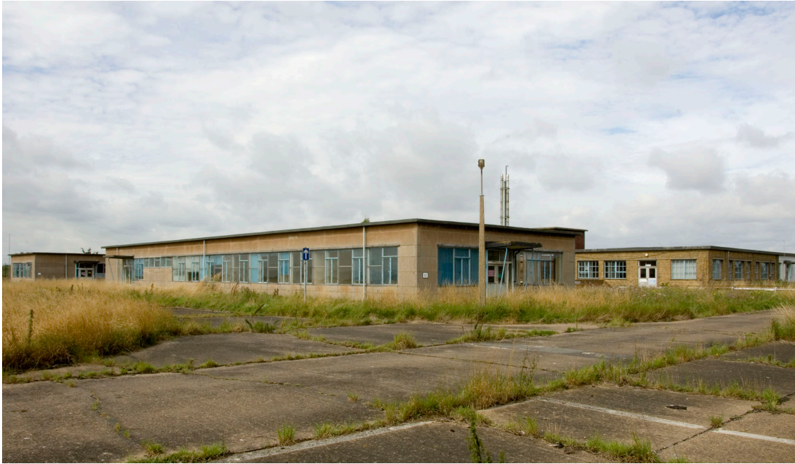
Figure 52: Prefabricated Laboratory L1 constructed about 1955 and to the right the slightly later brick built Electronics Laboratory L6. (c) English Heritage DP035967
