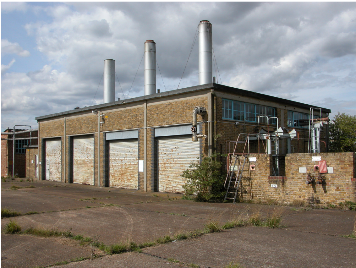
Figure 55: Boiler House E4. (c) English Heritage
