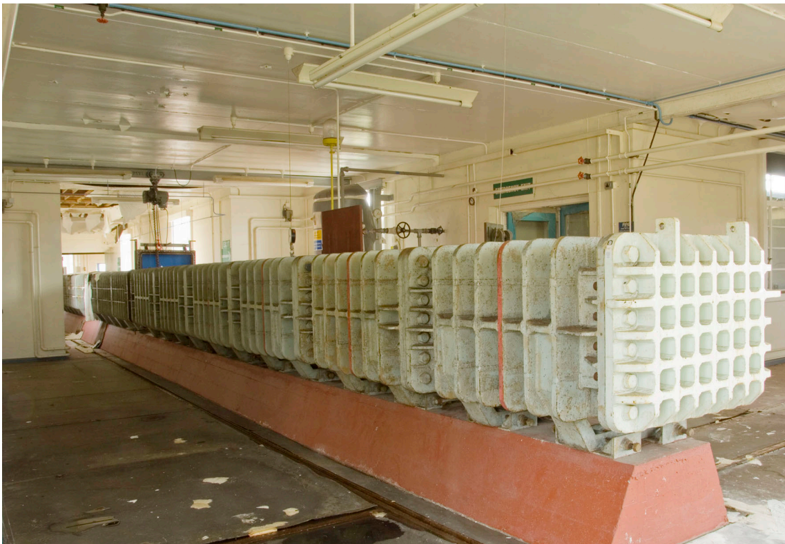
Figure 54: Shock Tube Laboratory H8, was 72, interior. (c) English Heritage DP035979
