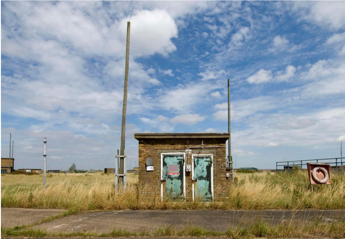
Figure 35: Special Store 22, now Magazine X3, was built in 1947, typical of this date is its brick construction and copper clad doors. Characteristic of explosives buildings are the lightning conductors, copper earth straps and external electrical fittings. DP035923 (C) English Heritage
