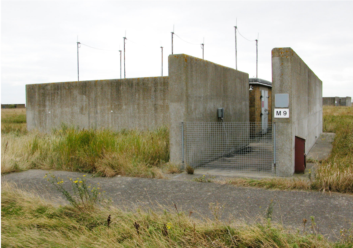
Figure 43: M9 Magazine, showing the typical protective L-shaped wall and inner brick magazine found in this area. (c) English Heritage
