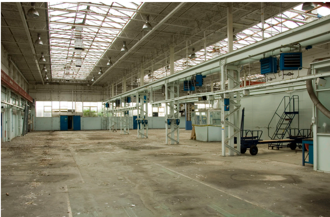
Figure 50: Main Mechanical Workshop E2, northern bay showing its steel framework construction and roof trusses formed from steel sections with tubular steel struts. (c) English Heritage DP035920
