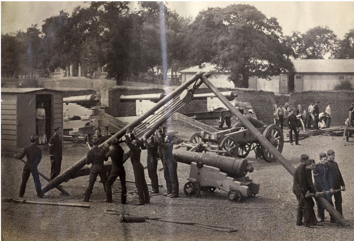
Figure 8: Cadets practising drill with a 'Triangle Gyn' in the southern-most bastion of the practice fortification. The photograph is probably one of a series taken by John Spiller in 1858 to illustrate the Repository exercises. Guns are visible mounted on fixed and travelling carriages and the buildings originally used as the gatehouse and for the horse artillery are visible in the background. Courtesy of the Royal Artillery Historical Trust (RAHT Collection AL27/26)
