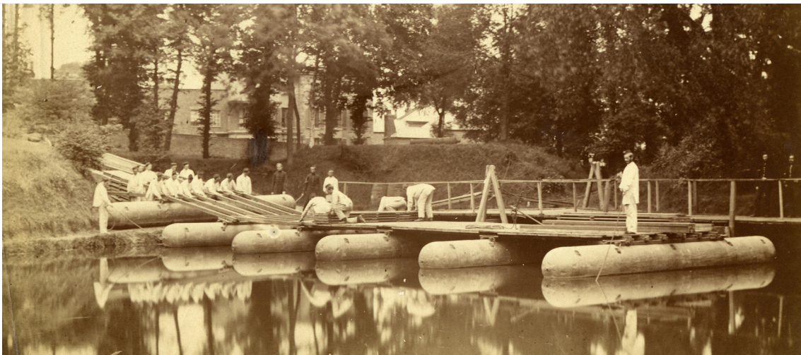
Figure 14: Cadets constructing a pontoon bridge across the north-western corner of the largest Repository pond circa 1858. A caption on a similar photograph, possibly taken at the same time, by Spiller described the components as 'Blanchard's cylindrical pontoons' (RAHT Collection AL28/12). The building marked 'Boat Store' on Bayly's 1867 map was located just out of shot to the left and houses located on Hillreach can be seen in the background. Courtesy of the Royal Artillery Historical Trust (RAHT Collection AL112 – no image number).
