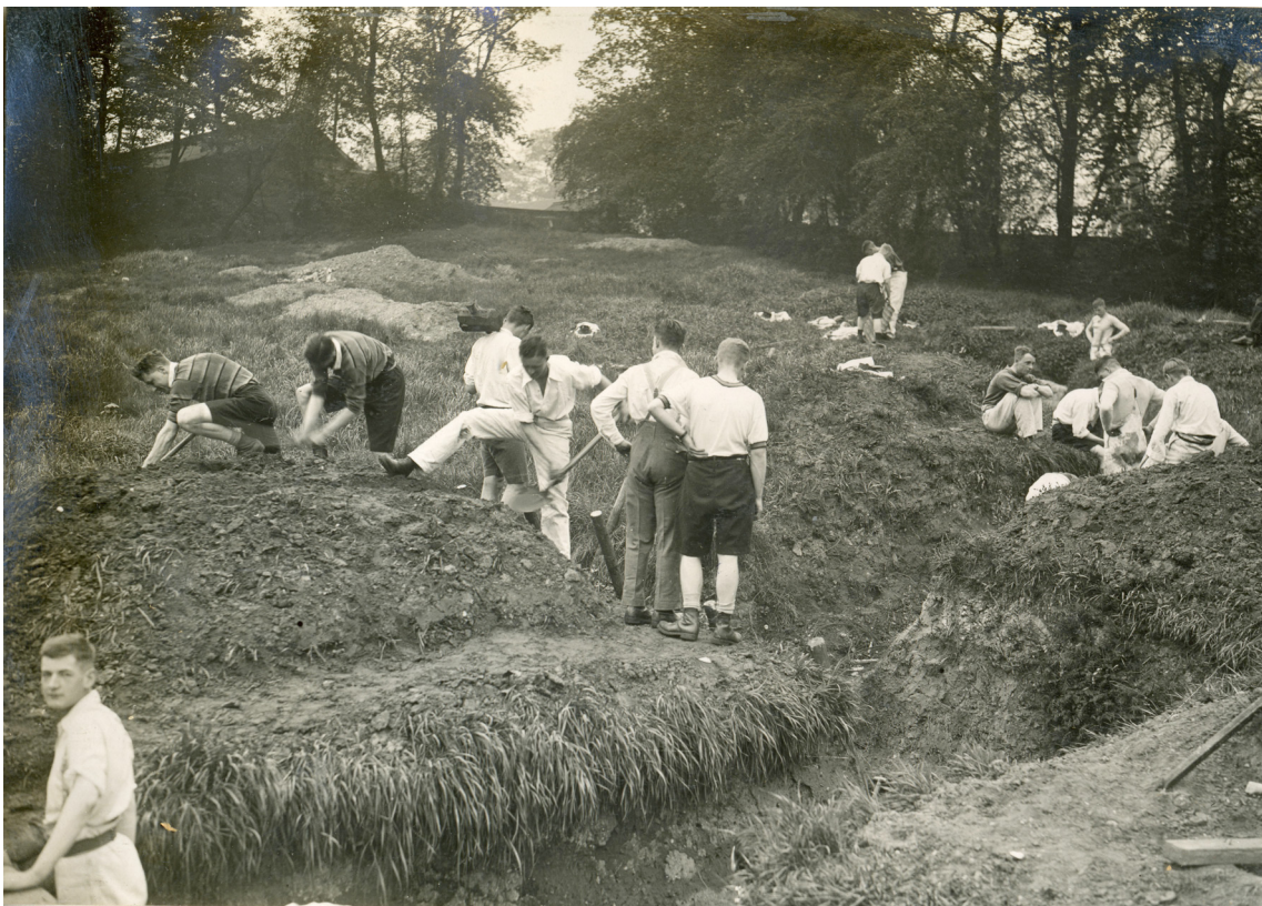
Figure 29: Cadets digging trenches in the Repository grounds at the western side of the small ponds some time in the early 20 th century. Photograph taken looking north-west. Courtesy of the Royal Artillery Historical Trust (RAHT AL27/64)
