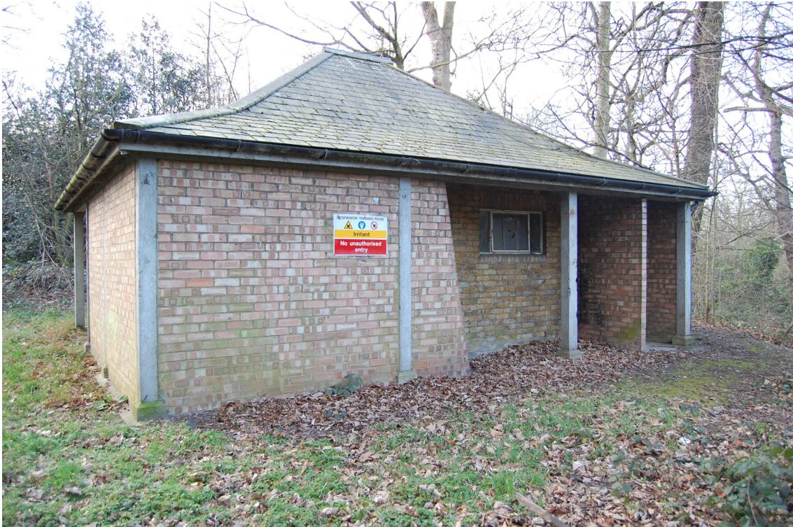
Figure 32: 20 th century pavilion-type building now in use as a 'Respirator Training Room'. Photograph: Sarah Newsome 2008 © English Heritage
