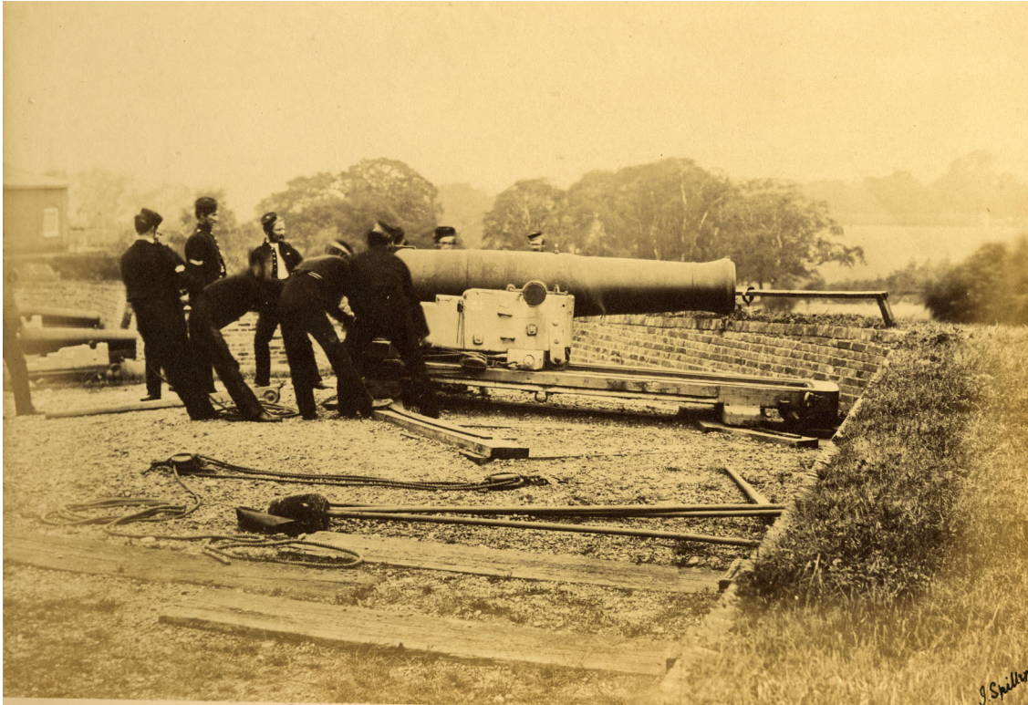
Figure 11: A photograph taken in 1858 by John Spiller showing a "10 inch gun 87 cwt on naval slide" positioned at the point of the Southern Bastion. The ground has been raised in this location in order to enable the gun to clear the parapet. The Rotunda is just visible to the left of the photograph. Courtesy of the Royal Artillery Historical Trust (RAHT Collection AL 933/15)
