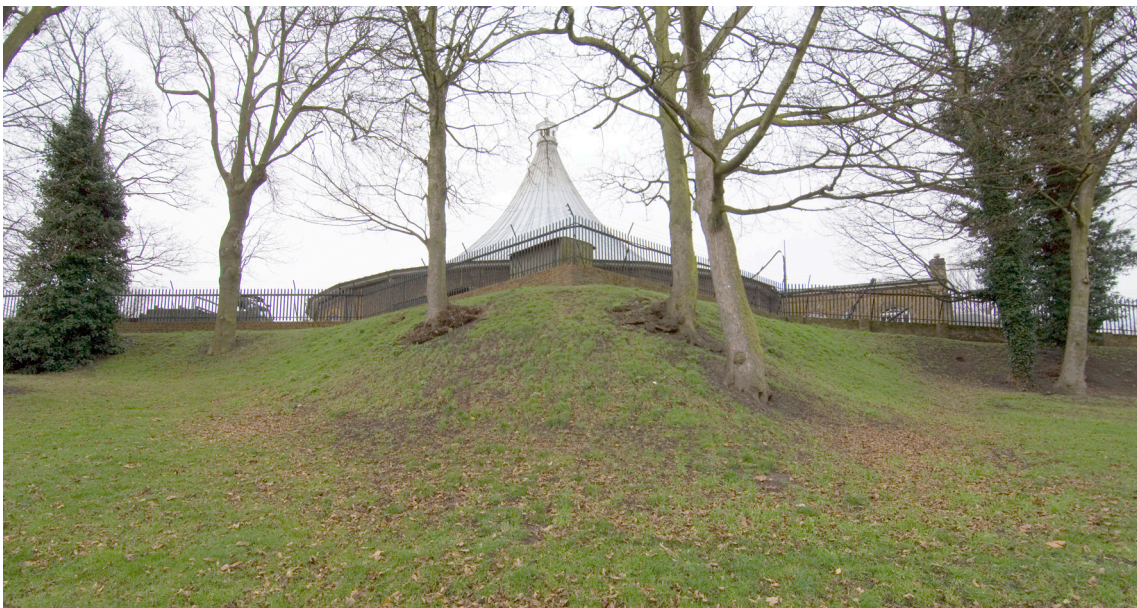
Figure 21: The Rotunda building from the east, framed by a large spur of the practice fortification. Photograph: Derek Kendall DP049765 © English Heritage
