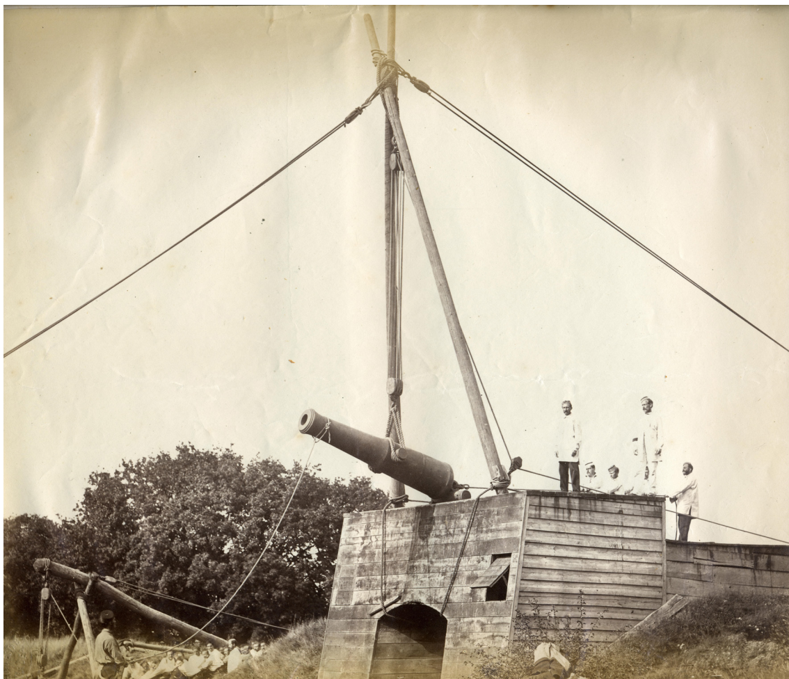
Figure 6: Earth and wood casemate probably located on the site of the 'dog kennels' in the modern Napier Line compound. The photograph is probably one of a series taken by John Spiller in 1858 to illustrate the Repository exercises. The same structure may be shown in this location on maps as early as 1808 and is depicted in detail on the Bayly map of 1867. Courtesy of the Royal Artillery Historical Trust (RAHT Collection AL27/42)
