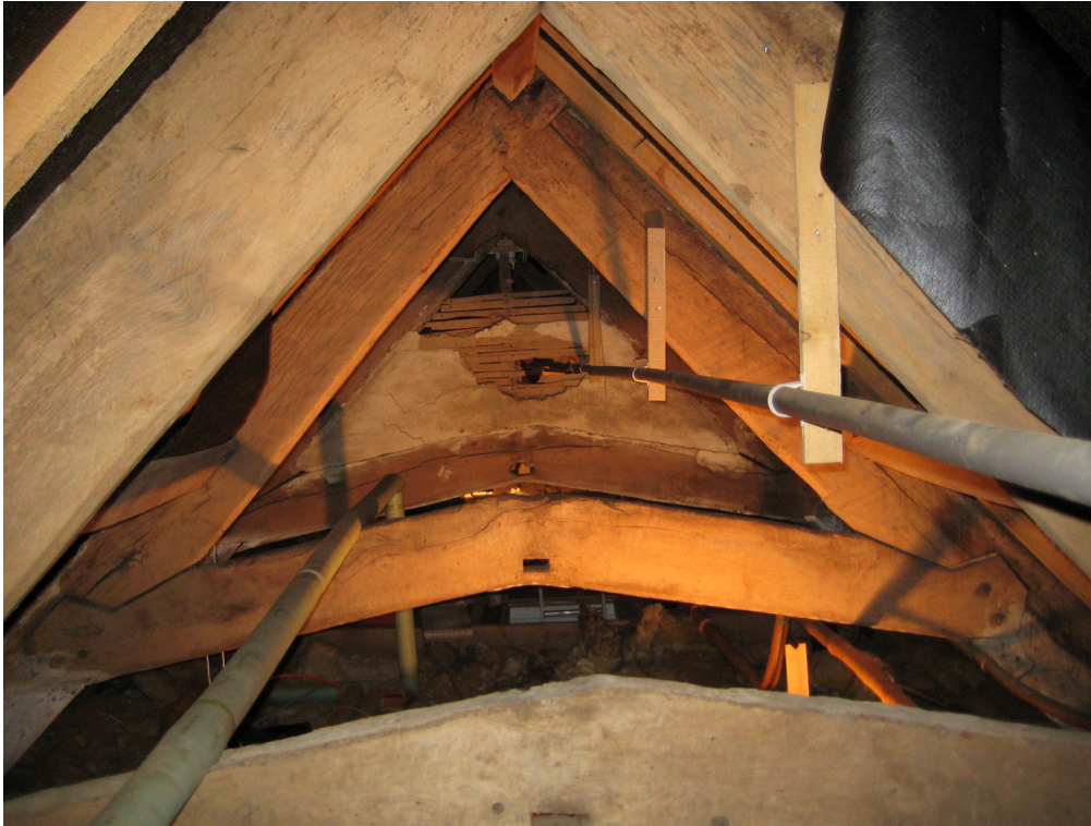
Figure 5: Roof timbers over the Great Hall viewed looking south-west
