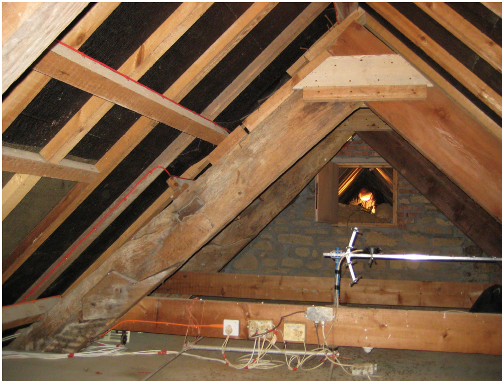
Figure 6: The east principals of Trusses 2 and 3 of the roof over the West Wing viewed looking south-east
