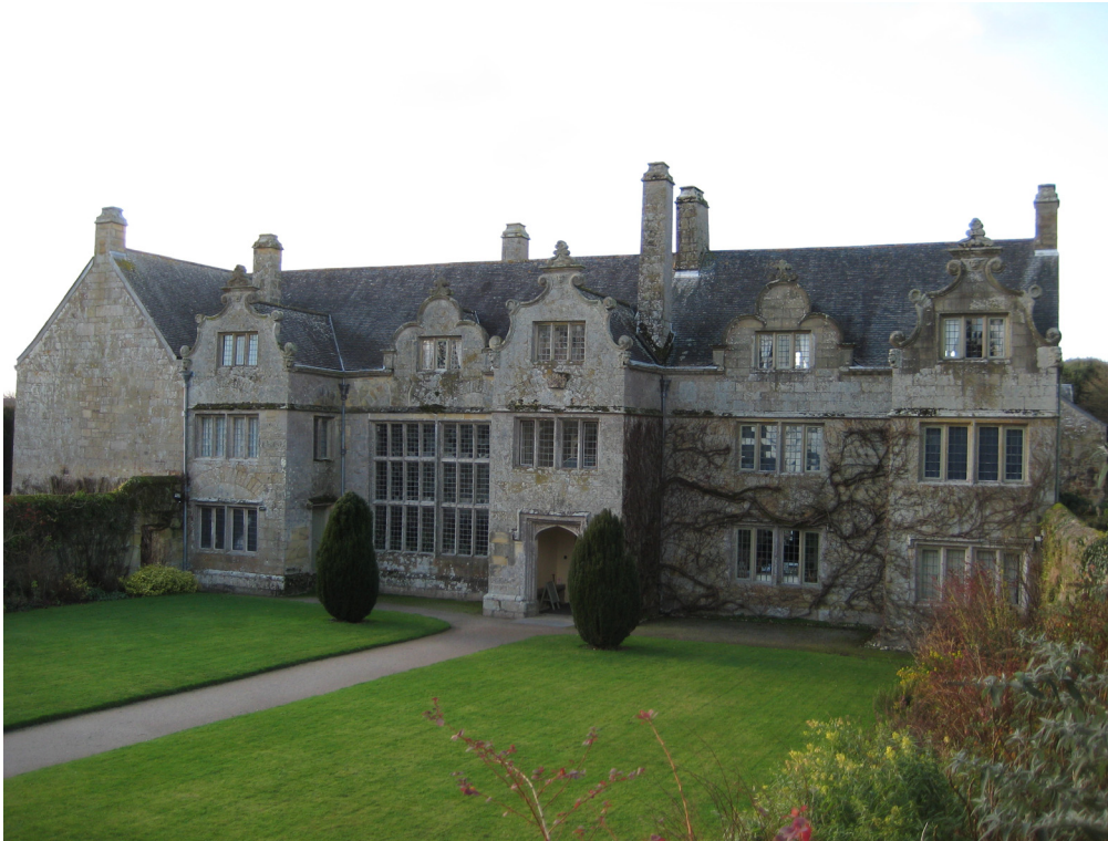
Figure 3: General view of the front north-east range of Trerice viewed looking west
