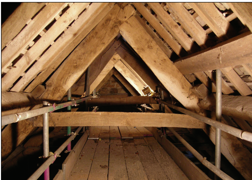
Figure 3: Cockle Park Tower; main range roof looking south (truss 3 in the foreground)
