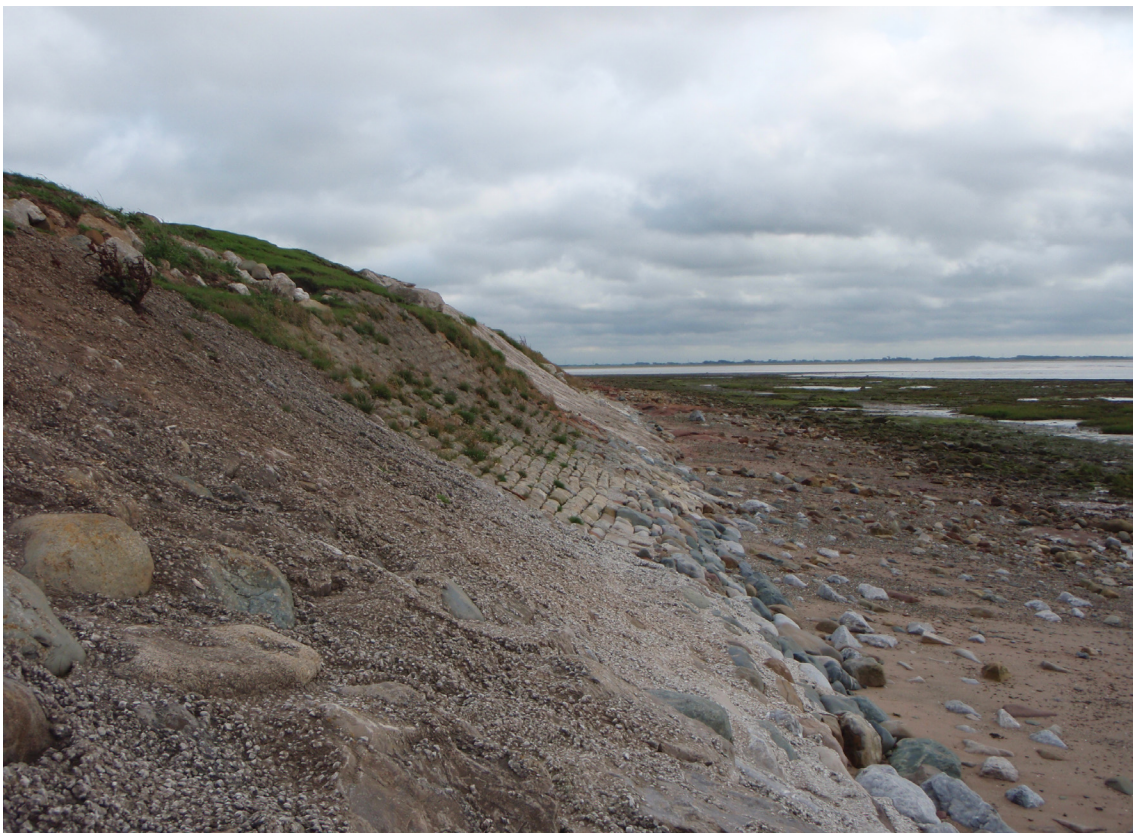
Figure 10. View south along the sea wall showing areas of erosion at its base
