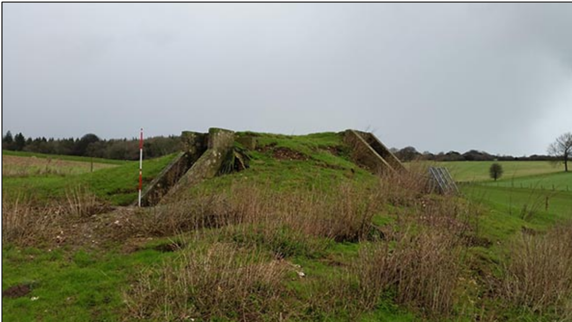
Figure 80 Gumber Farm decoy control bunker and generator remains photographed in January 2016 © SDNPA
