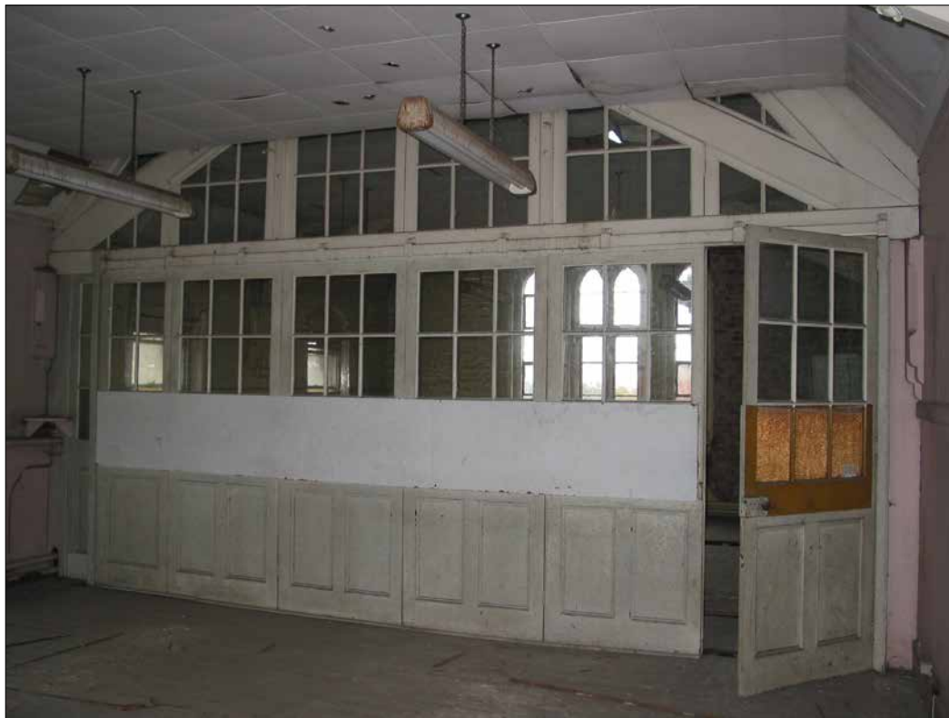
Figure 41: Second-floor interior of chapel-wing extension (© Historic England, photograph: Adam Menuge).
