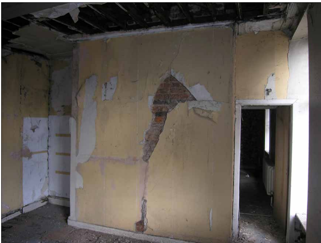
Figure 31: Bedroom 5 on the first floor (© Historic England, photograph: Adam Menuge).
