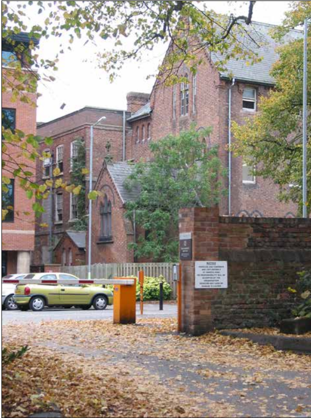
Figure 37: The rear of the chapel-wing extension (© Historic England, photograph: Adam Menuge).
