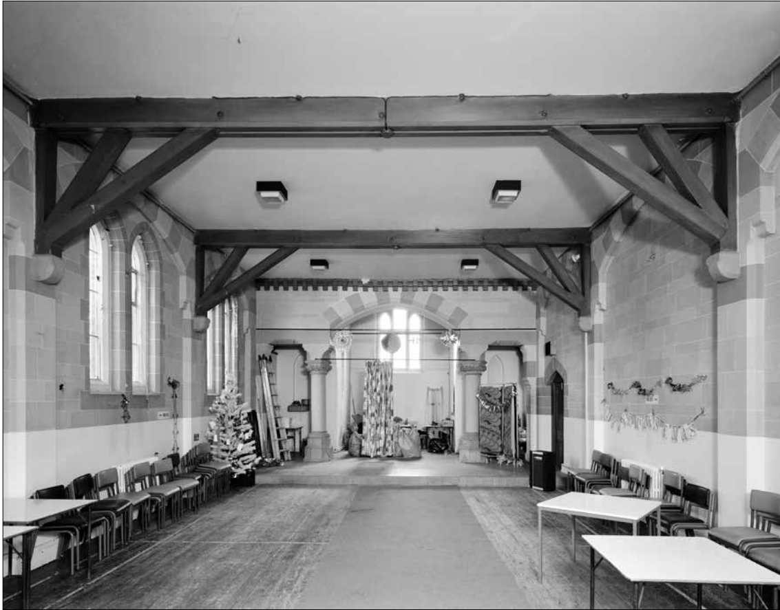
Figure 38: Ground floor of the chapel-wing extension looking south in 1991 (BB91/26355 © Historic England, photograph: Bob Skingle).
