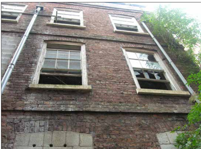
Figure 19: Window bays at the rear of the original house (© Historic England, photograph: Adam Menuge).
