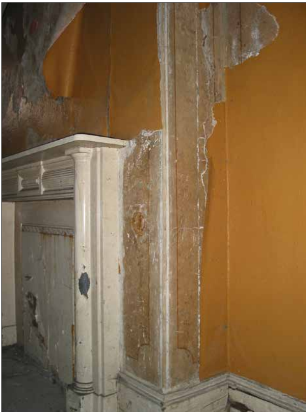
Figure 33: Early-19th-century applied decoration in the drawing room (© Historic England, photograph: Adam Menuge).
