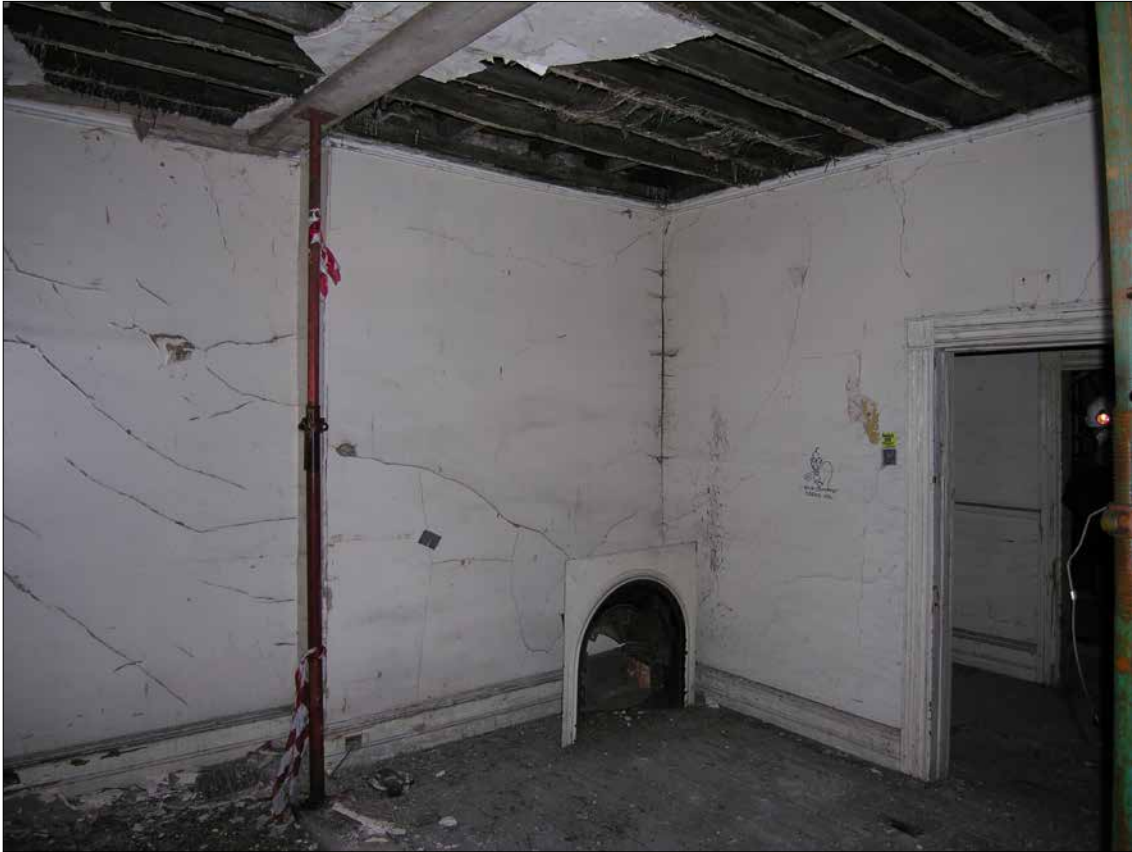
Figure 27: Bedroom 2 on the first floor (© Historic England, photograph: Adam Menuge).
