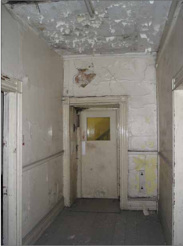
Figure 34: First-floor corridor between bedrooms 2 and 3 (© Historic England, photograph: Adam Menuge).
