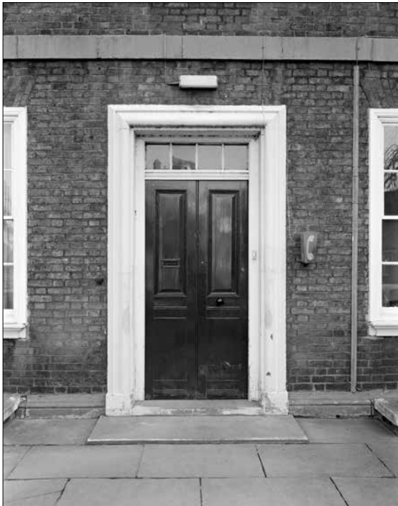
Figure 17: Bolection moulding on the original front entrance in 1991 (BB91/26352 © Historic England, photograph: Bob Skingle).
