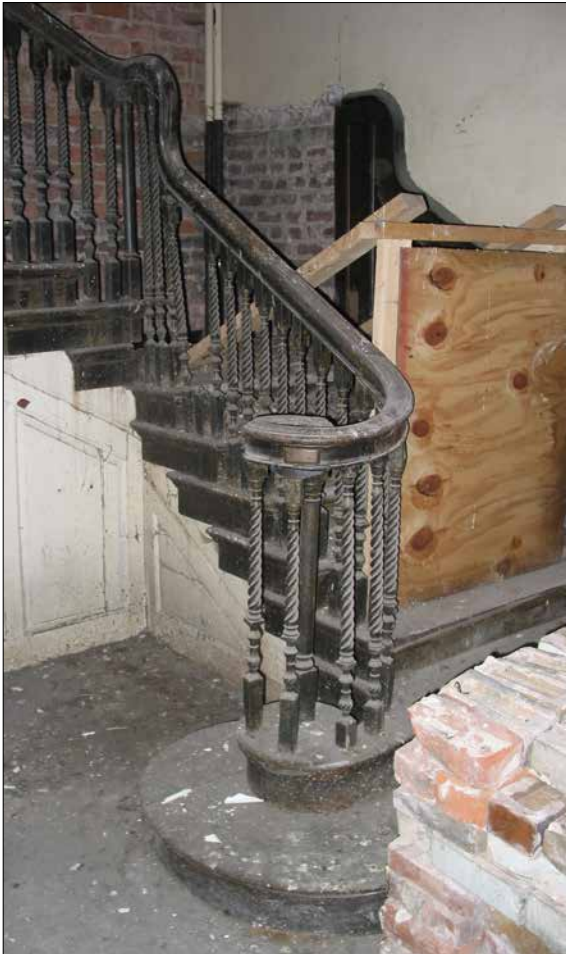
Figure 21: The main staircase (© Historic England, photograph: Adam Menuge).
