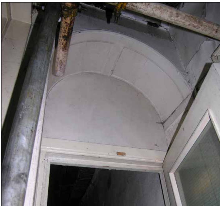
Figure 29: Panelled archway between the stair-landing and the rear first-floor corridor (© Historic England, photograph: Adam Menuge).
