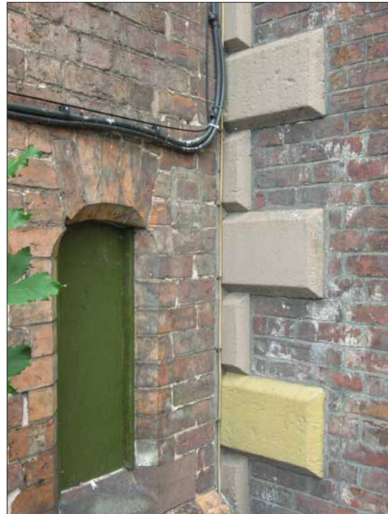
Figure 18: Partially concealed quoins at the north-east corner of the original house (© Historic England, photograph: Adam Menuge).
