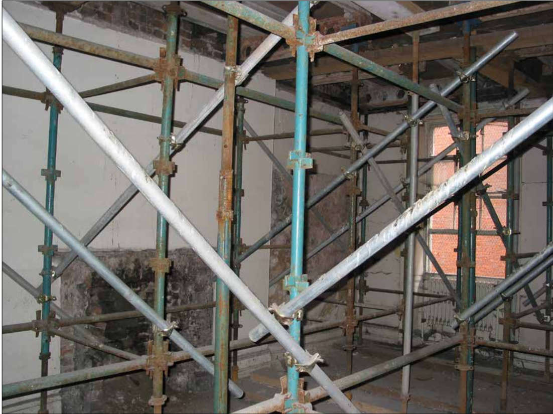
Figure 28: Bedroom 3 on the first floor (© Historic England, photograph: Adam Menuge).
