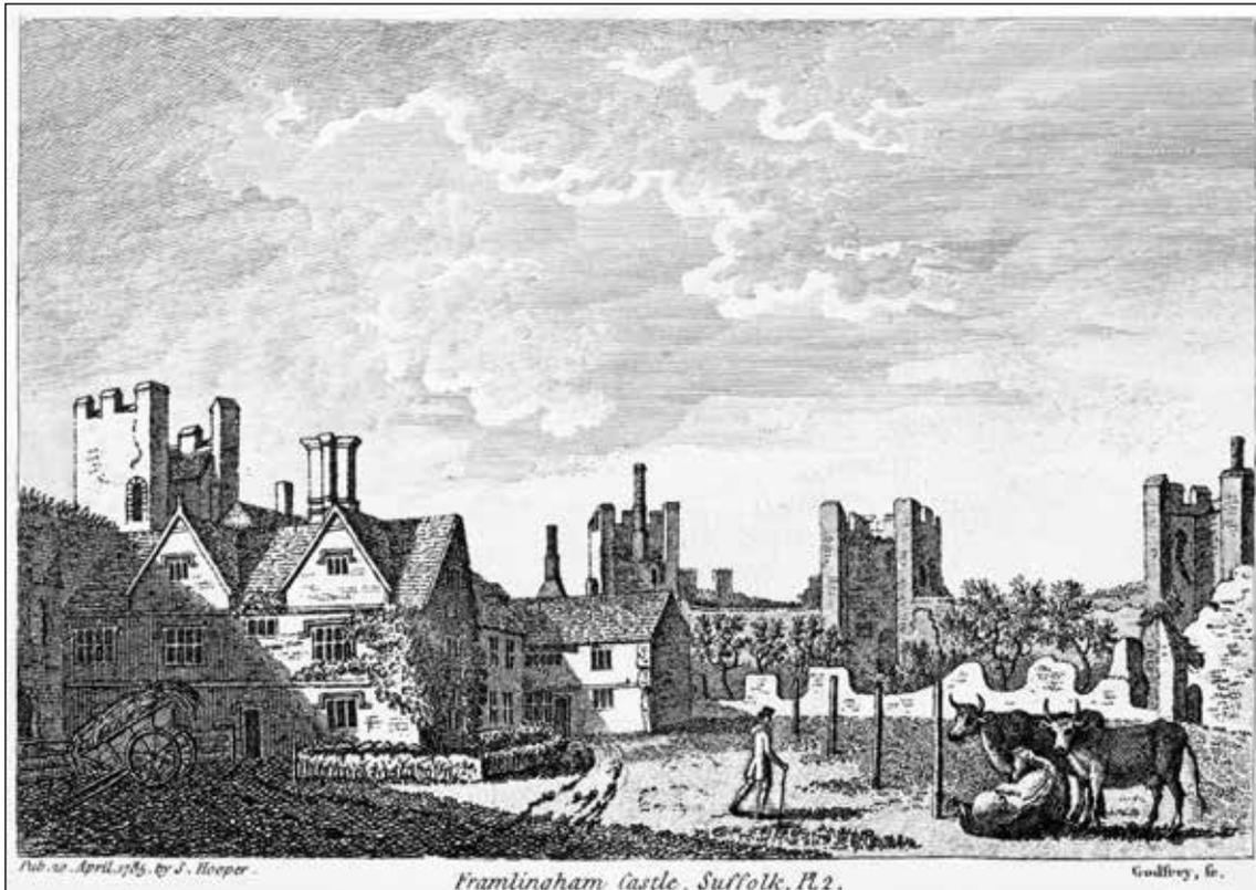
Fig. 15 An engraving by Samuel Hooper, showing Framlingham Castle after the demolition of most of the north range. Part of its rear wall was retained to enclose a garden on the north. Compare Fig. 13. (Historic England Archive)
