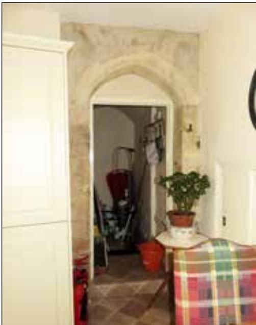
*Fig. 55 (left) Doorway within the curtain wall, in the present kitchen (west room). Note the serving hatch just visible to the right (see also Fig. 23). (© Historic England, K. Morrison)*
