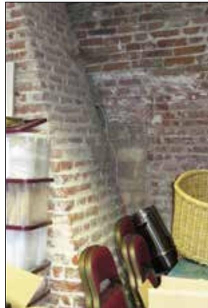
*Fig. 49 A blocked first-floor window on the north elevation of the Red House, visible to the right of the 1729 chimney stack. (© Historic England, K. Morrison)*
