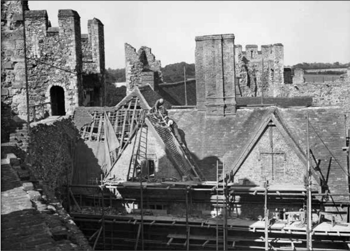
*Fig. 37 Repairs to the roof of the Red House, 12 September 1933. (© Historic England Archive, OWS01/02/F01172)*
