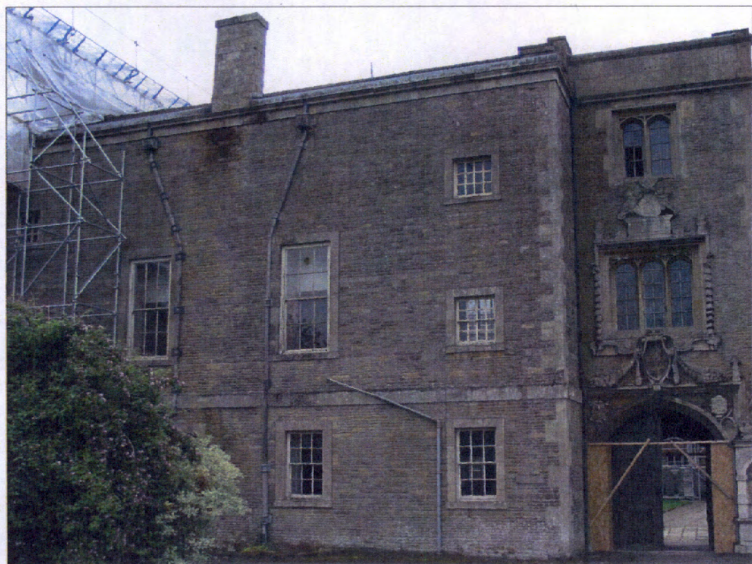
Figure 7.45 The north front of the Library Block.
