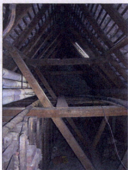
Figure 7.52 The roof over the Archway passage. Pete Smith 2006
