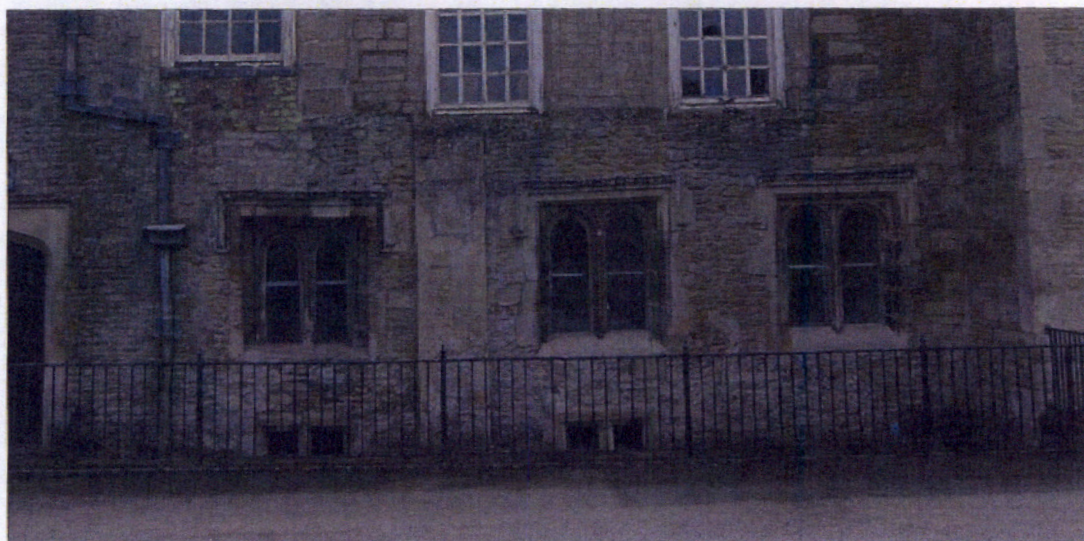
Figure 7.16 The north front of the former Housekeeper's Room and the Cellar.
