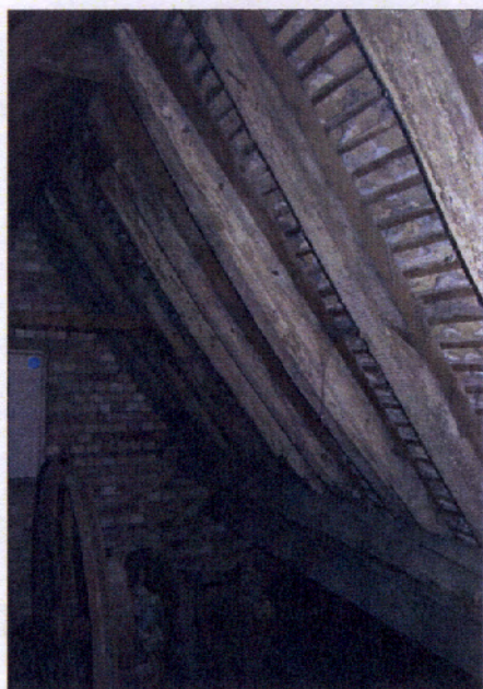
Figure 7.40 The roof of the former Brewhouse. Pete Smith 2006
