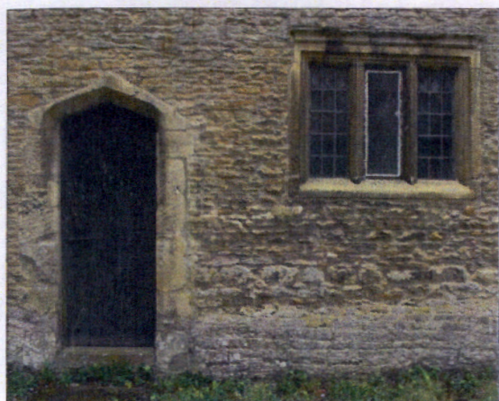
Figure 8.3 Laundry doorway and window, detail. Kathryn Morrison 2005
