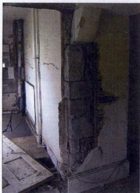
Figure 7.18 The quoins exposed at the north-west corner of the Service Block. Pete Smith 2006
