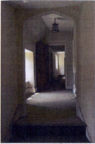
Figure 7.20 The inner side of the doorway on the first floor of the Service Block.
