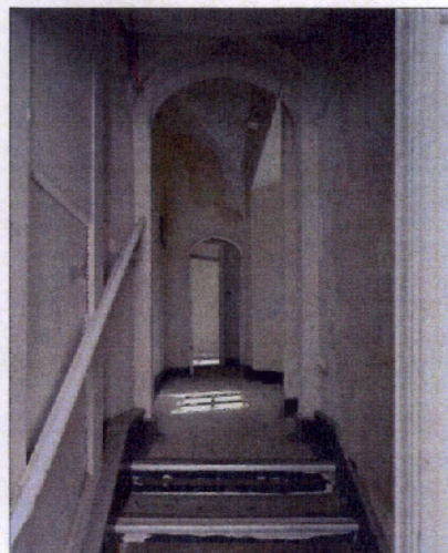
Figure 7.11 The inner side of the doorway on the first floor of the Gate Tower. © English Heritage BB039801
