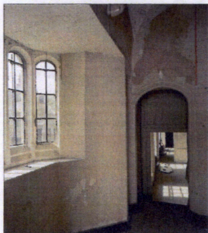
Figure 7.8 The doorway on the first floor of the Gate Tower.
