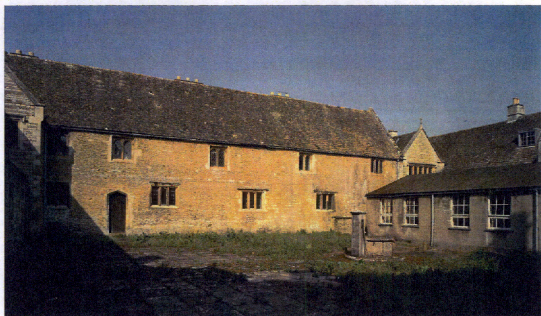
Figure 8.1 West Range, view from south-east, 2005.
