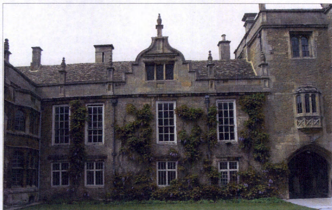
Figure 7.32 The south front of the North Lodging Block.
