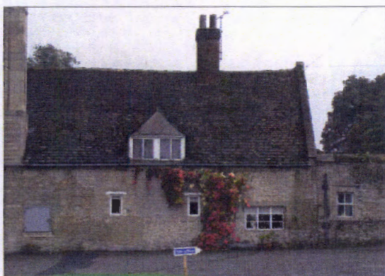
Figure 7.50 The north front of the Gardener's Cottage.
