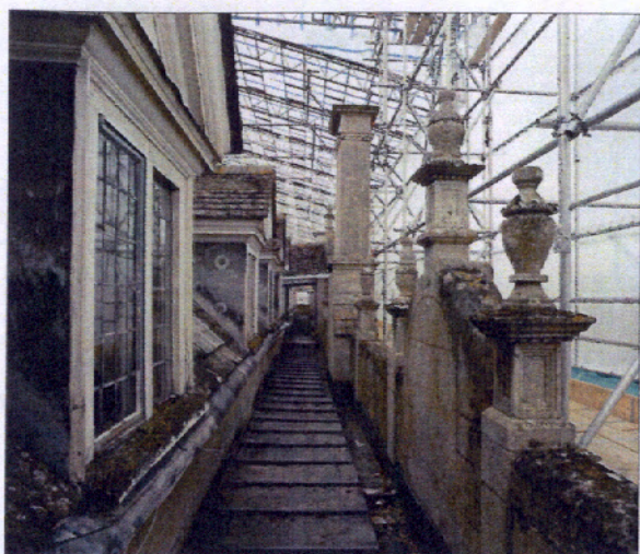
Figure 10.25 East range roof walk, looking north. © English Heritage AA052088
