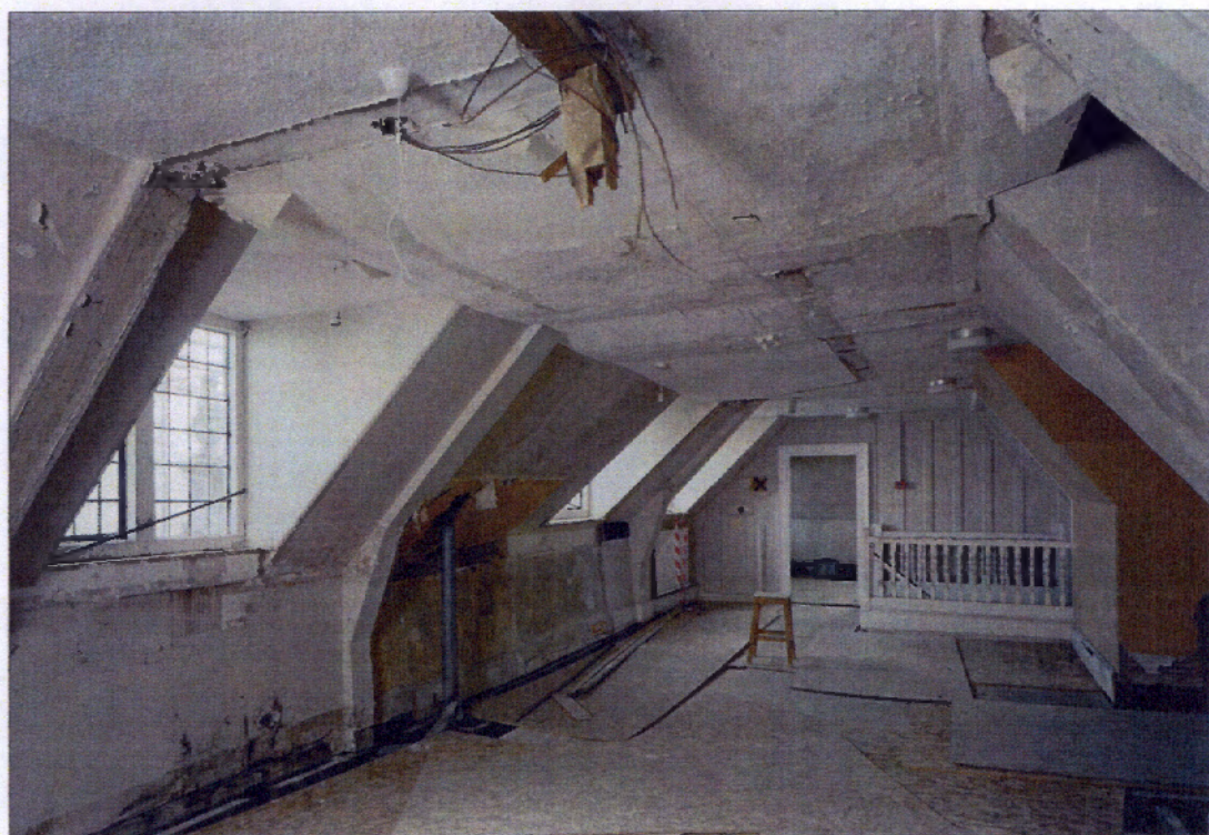
Figure 10.24 East range attic, looking south towards top of Spencer Stair.
