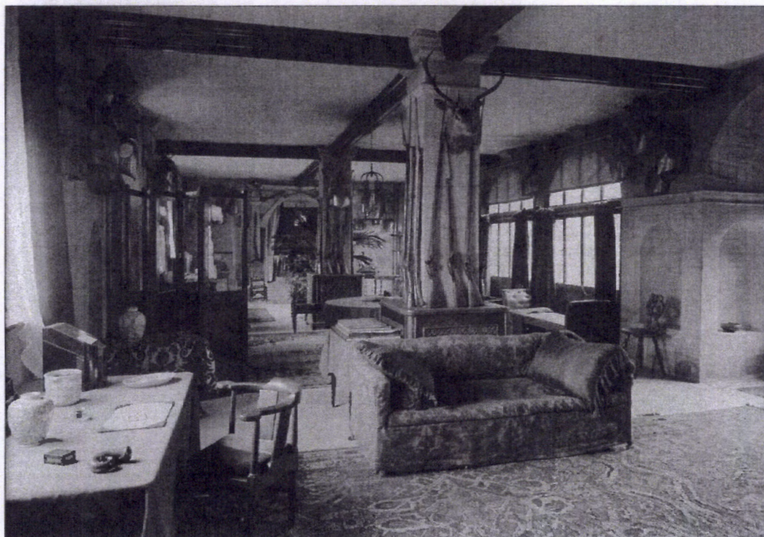
Figure 10.35 Front Hall looking south, by Bedford Lemere, 1904.
