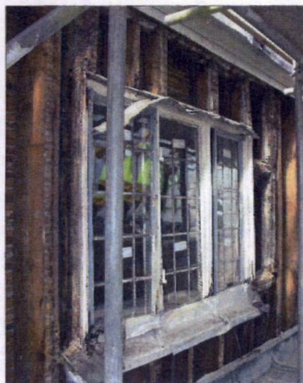
Figure 10.29 Window in south wall of attic, inserted within larger window opening, 2006.
