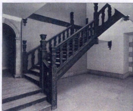
Figure 10.38 Oak Stair, installed 1922, RCHME 1978. © Crown copyright.NMR
