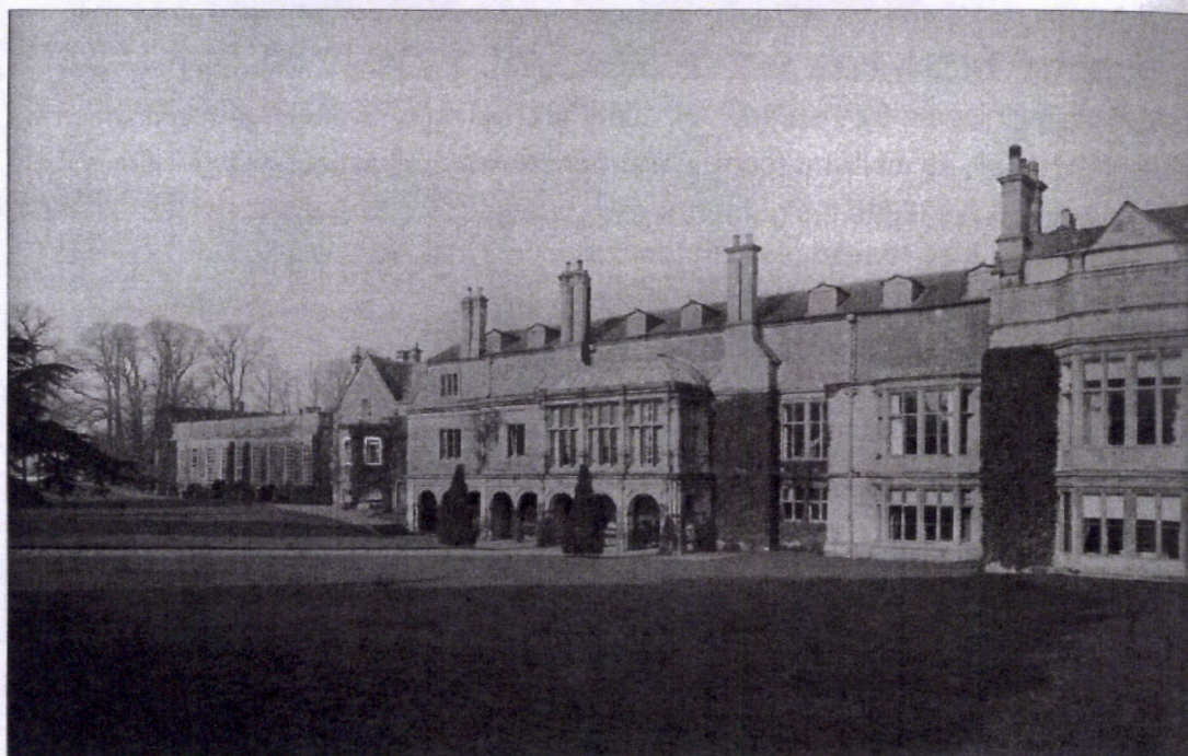
Figure 9.45 South range, view of south front showing dormers (c.1740) and conservatory (1846-49), by Bedford Lemere, 1904.
