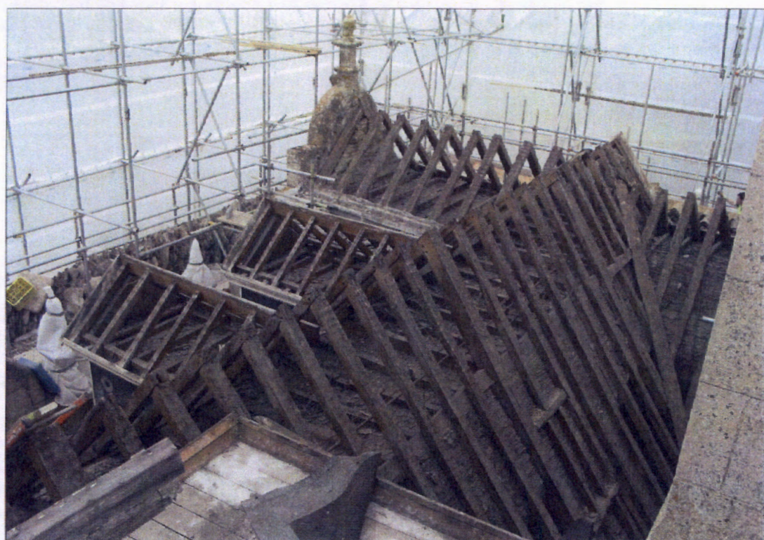
Figure 10.28 Roof over south end of east range, summer 2006.
