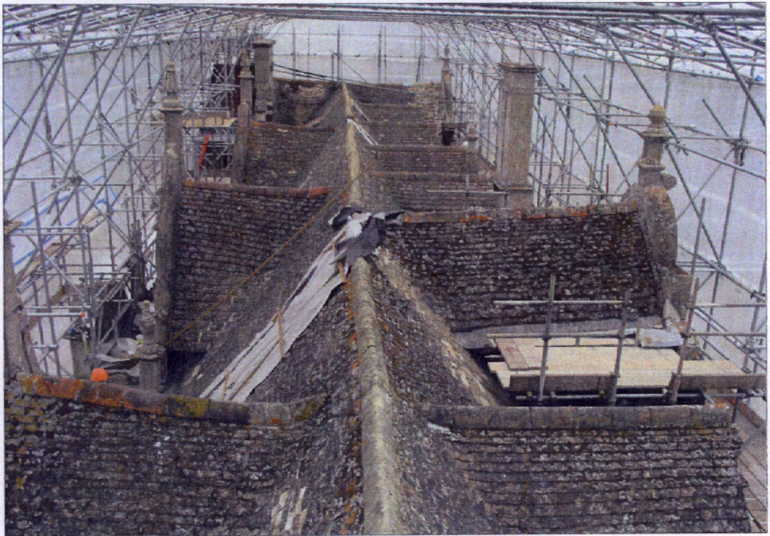
Figure 10.7 Roof of east range looking north, spring 2006.
