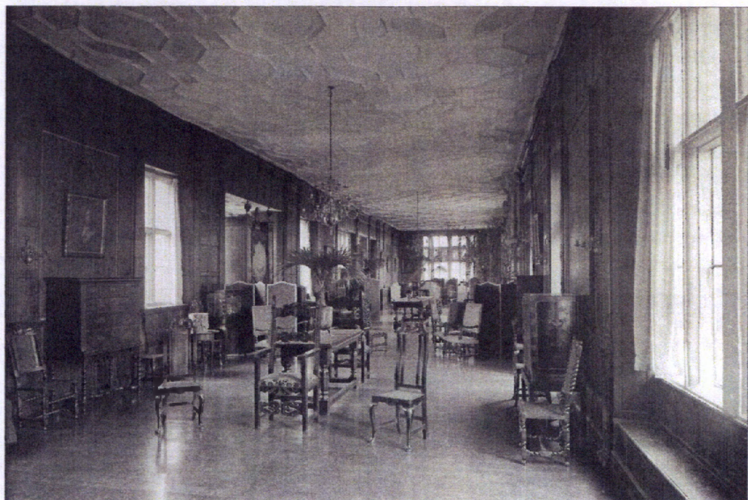
Figure 10.18 Long Gallery looking north, by Bedford Lemere, 1904. © English Heritage NMR
