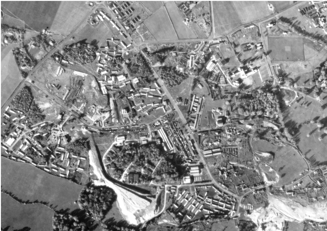
Fig 65: Military development at Corsham showing the extent of the camp by 1946. In addition to new buildings the development includes two large spoil heaps showing white at the bottom of the photo. (Detail of RAF CPE/UK/1821 3023 4-NOV-1946 Historic England RAF Photography)
