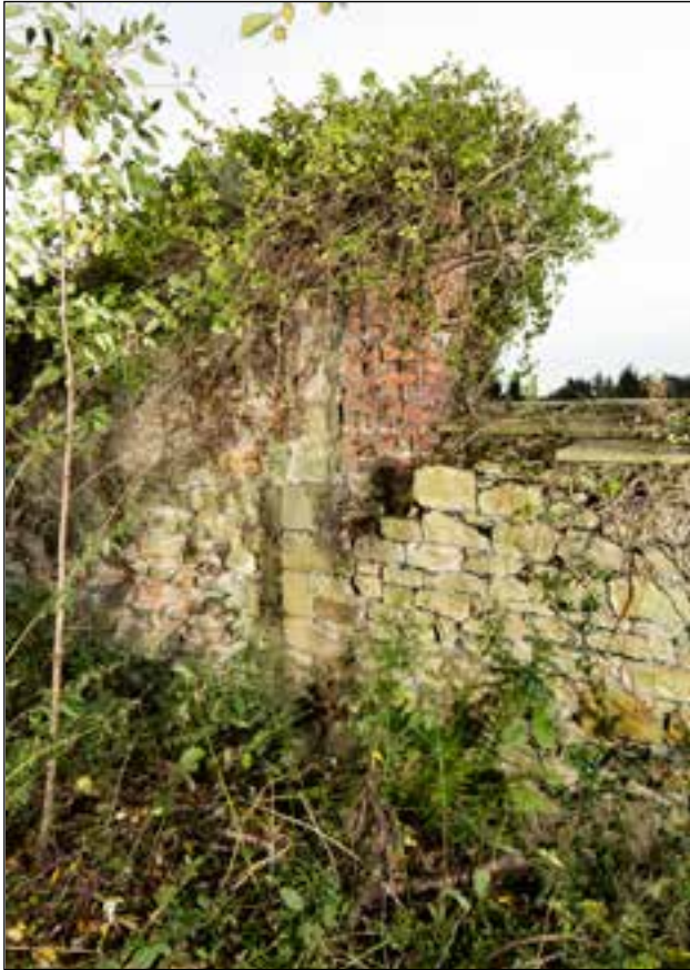
Figure 20: Straight joint (I) on the north face of the garden wall (DP174242 © Historic England, photograph taken by Alun Bull)
