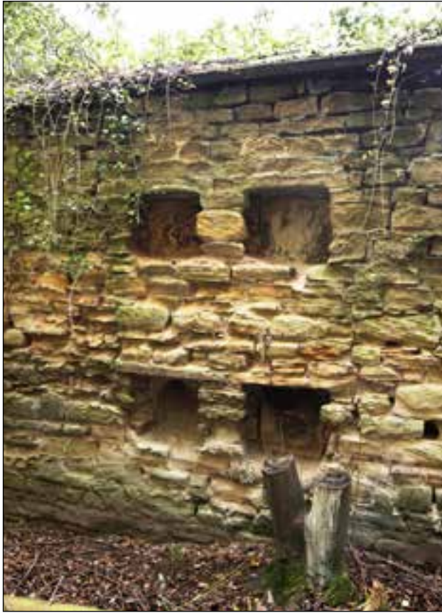
Figure 21: Flue openings on the north side of the garden wall, west of projection E (DP174238 © Historic England, photograph taken by Alun Bull)
