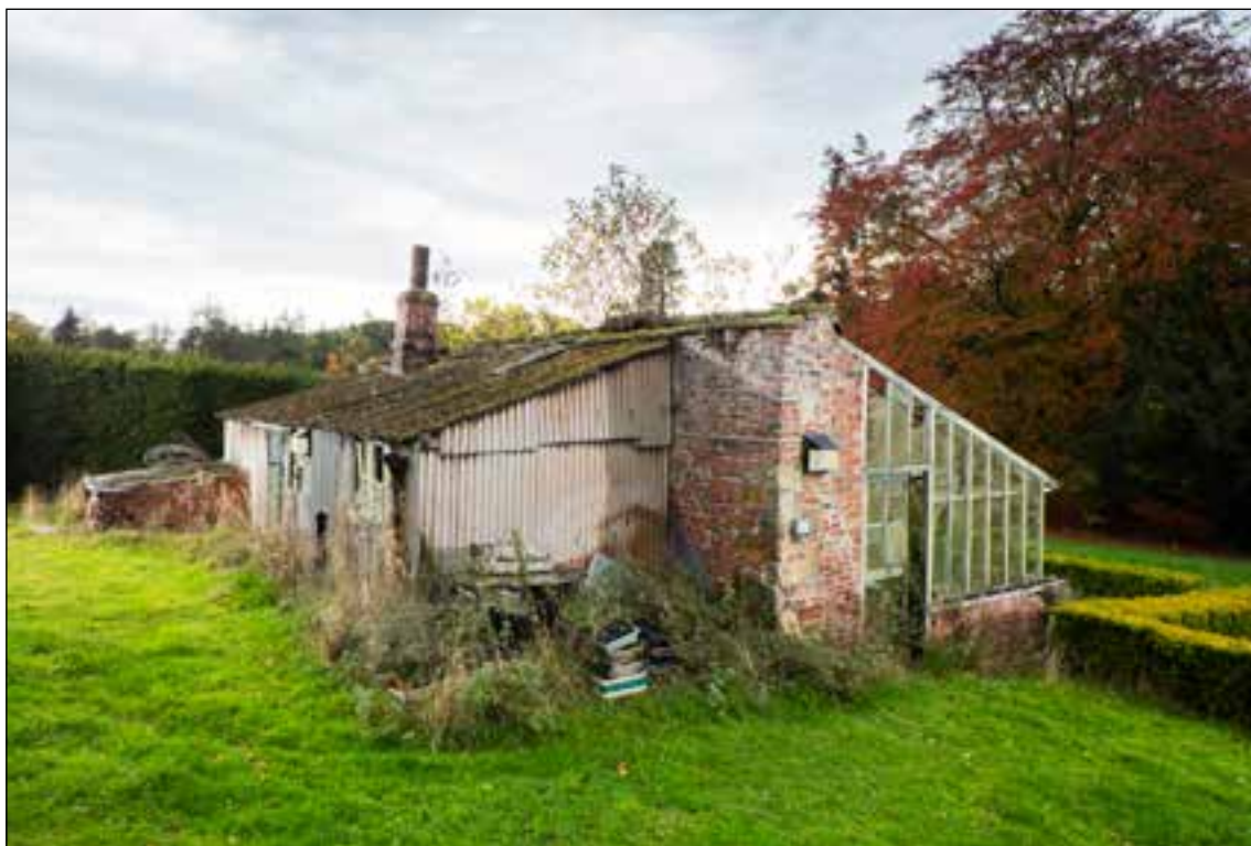
Figure 28: Glass house in the western part of the garden incorporating early brickwork and stone (DP174213 © Historic England, photograph taken by Alun Bull)
