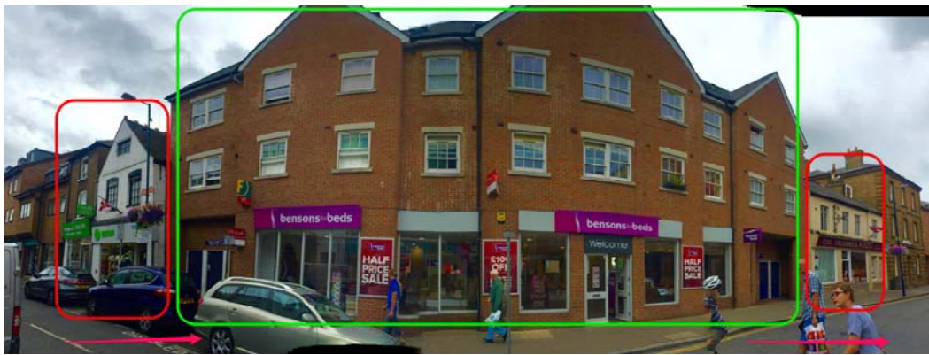
Nos 6-28: A low-quality historicist scheme of the 2000s which adversely affects listed buildings either side of it
