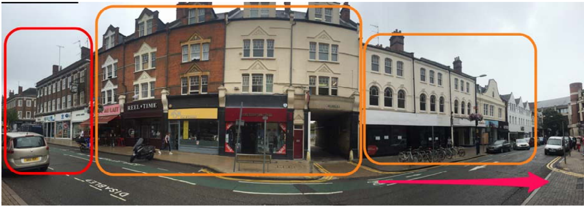
Fife Road: South side
