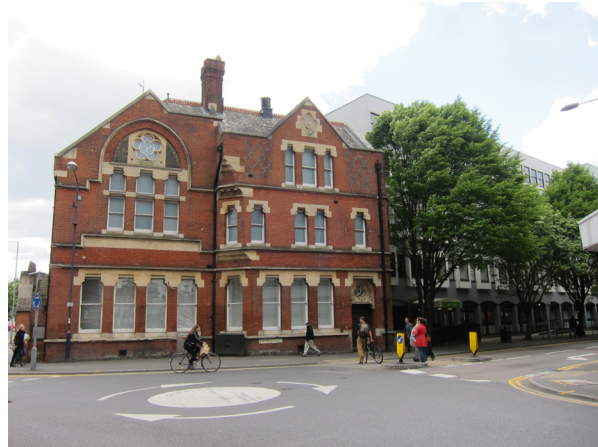
Fig.15 Post Office, Brook Street (listed Grade II) and job centre (right)
