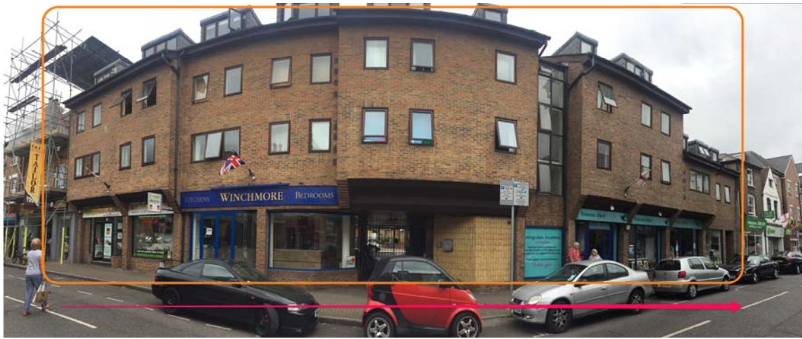
Nos 34-44: A housing/retail scheme of the late 1970s/early 1980s that fits comfortably into the diverse historic setting of Old London Rd, with a designed-in variety of massing across a large structure which acts to break up bulk
