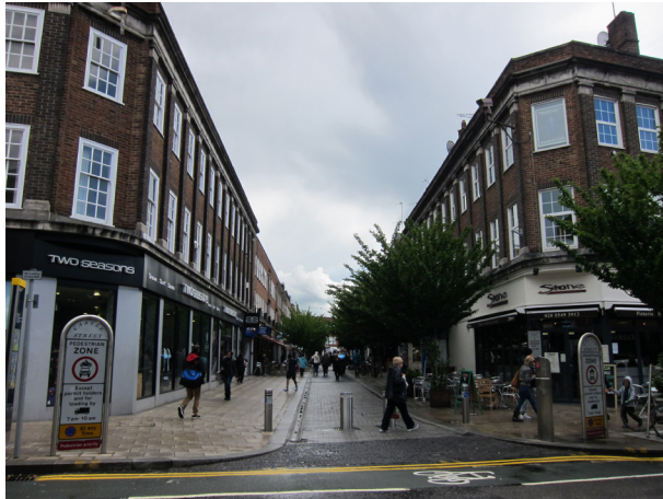
Fig.4 Castle Street: 1939 shopping parade with flats above, accessed from the rear. © Historic England
