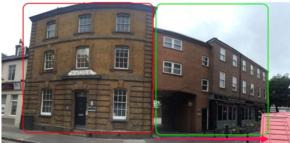
Nos 2-6: The Grade II listed old Police Station has low quality neighbours but historic patterns are maintained by the retention of a carriage arch
