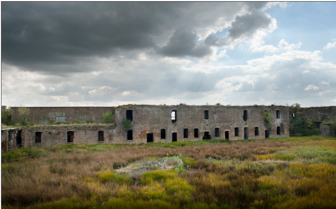
Figure 30: View of the south range across the parade ground. On the left are the single storey officers' quarters with loopedholed parapet above. The two-storey section on the right has the barracks on the ground floor with the hospital above. (DP 097500)
