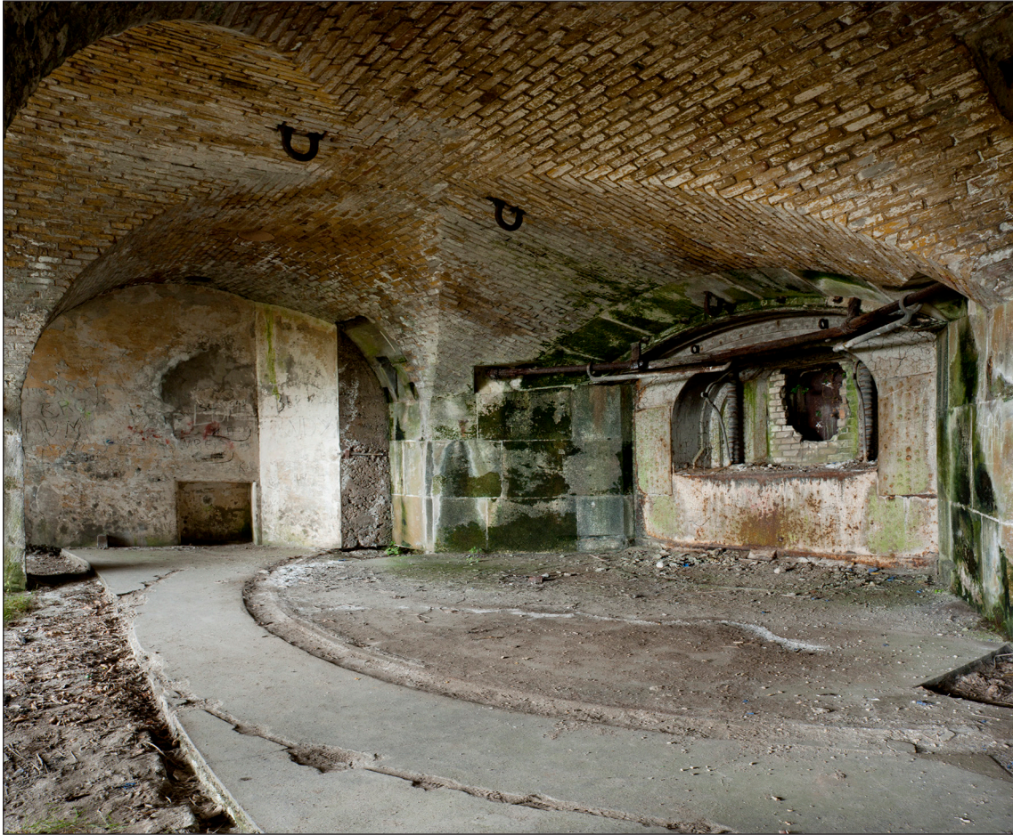
Figure 20: The remains of two racer rails for the 11-inch RML embedded in the floor of Casemate 8. The narrow slot for the training arc extends beyond the limit of the concrete floor in the northern portion of the casemate, suggesting another floor surface has been removed, perhaps timber boards. (DP097607)
