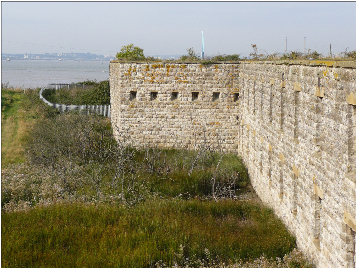
Figure 23: The loopholed flank wall of the south-west bastion looking west © Historic England
