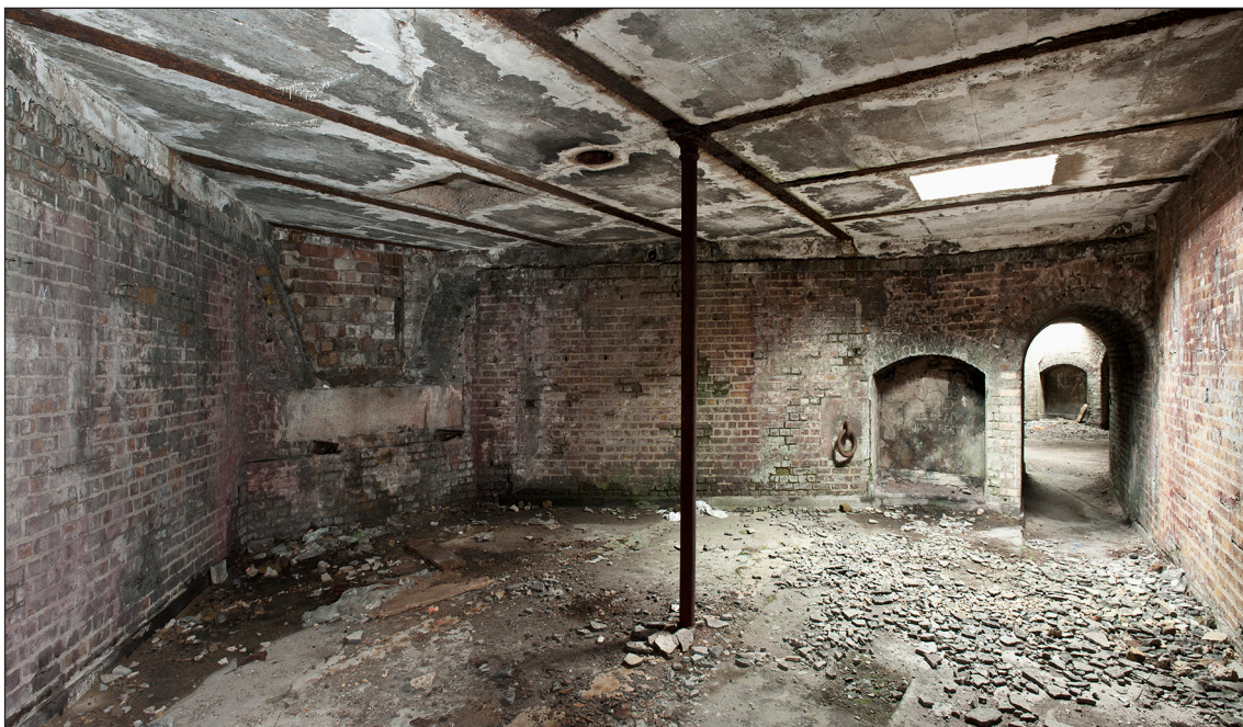
Figure 22: The southern former open gun emplacement looking north towards the second open emplacement. The blocked brick gun embrasure can be seen to the left of the image whilst the ring and set back associated with traversing the gun can be seen to the right adjacent to the passage which connects this emplacement to the one to the north. (DP097650)
