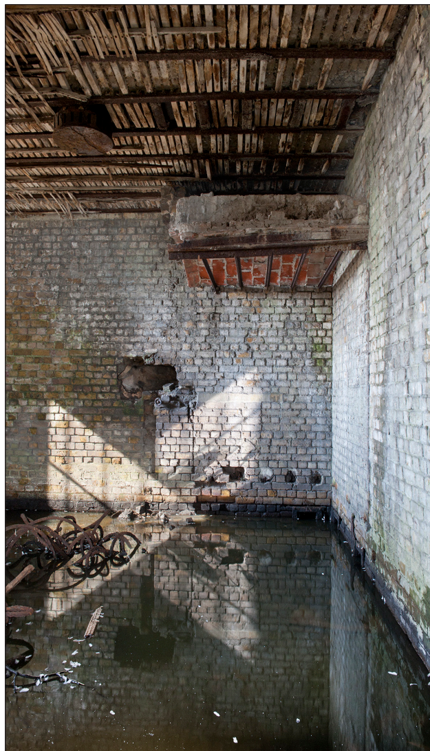
Figure 38: Possible remains of hot-air closet in north-western corner of the Wash Room and Laundry. (DP097512)
