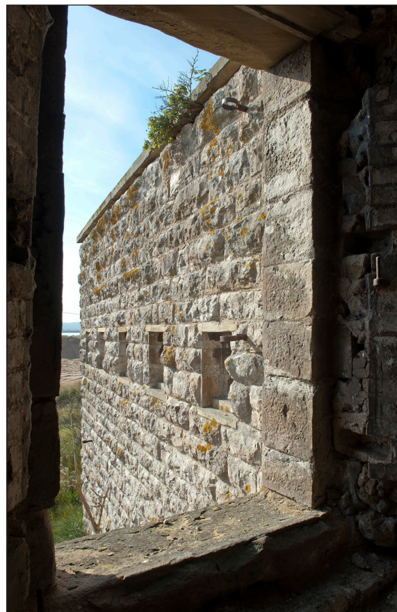
Figure 36: Loopholes on the eastern face of the south-eastern demi-bastion as seen from the hospital lavatory. Iron brackets that held downpipes can also be seen. (DP 097504)
