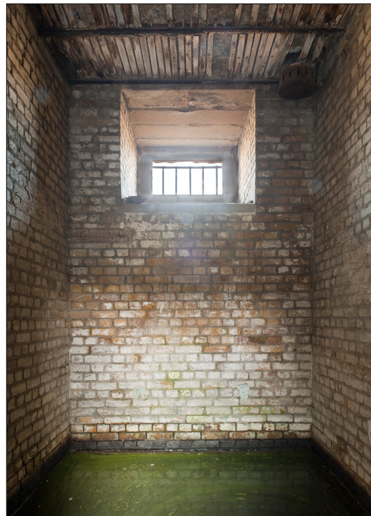
Figure 28: The high-set window of the eastern cell. (DP097466)
