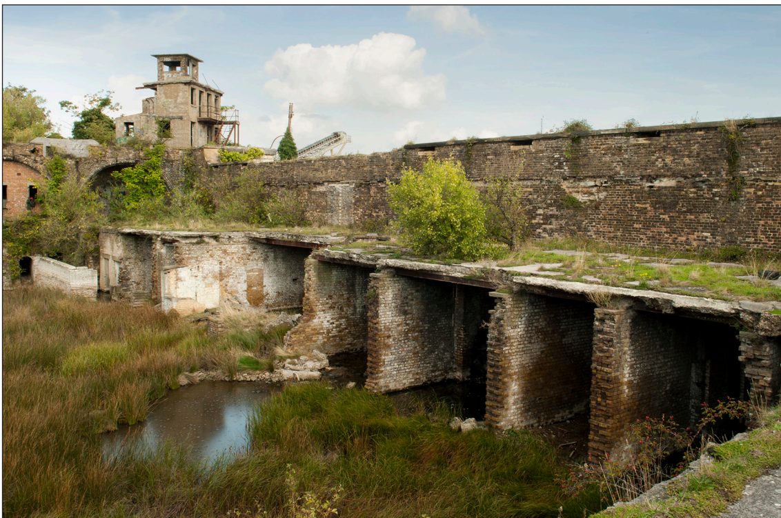
Figure 26: The fort interior in September 2010, from the southern range looking north-east. The fort entrance is in the centre of the picture and is flanked by the remains of the east range buildings which have had their front walls demolished. At the top of the gorge wall the loopholes set beneath the capping stones can be clearly seen. The horizontal scar beneath them indicates the course of the removed chemin de ronde. (DP097577)
