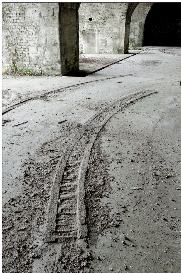
Figure 43: The cogged racer rail in Casemate 12 suggesting that alterations were made to the carriages in this casemate. (DP097629)
