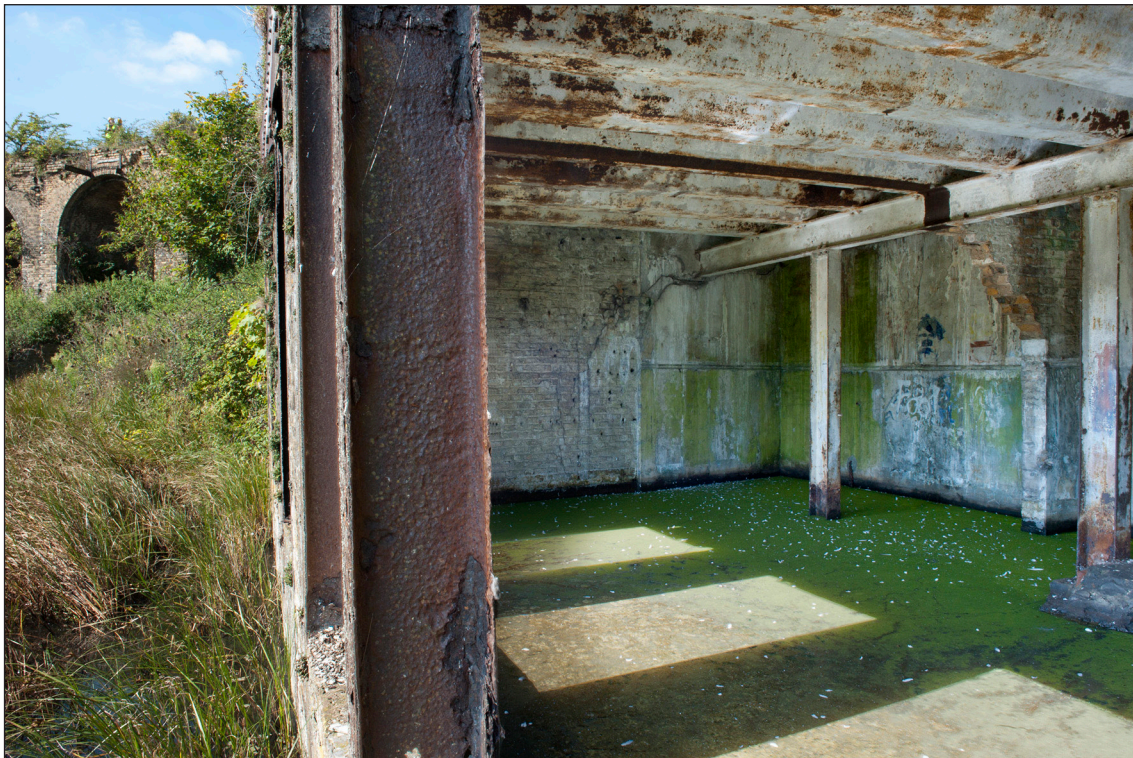
Figure 73: The interior of the Engine and Dynamo House [70, 71]. The later (presumed Second World War) steel-beam and ribbed-section roof can be clearly seen. The black stripe running across the roof indicates the position of the former dividing wall between the Engine and Dynamo Rooms. The corner of the engine base can just be seen to the right of the picture. (DP 097558)
