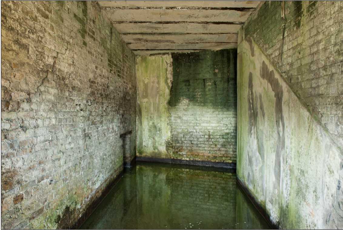
Figure 63: The interior of the coal store with the coal hatch at the base of the left hand wall and the render on the right hand wall marking the line of the original traverse. (DP097545)
