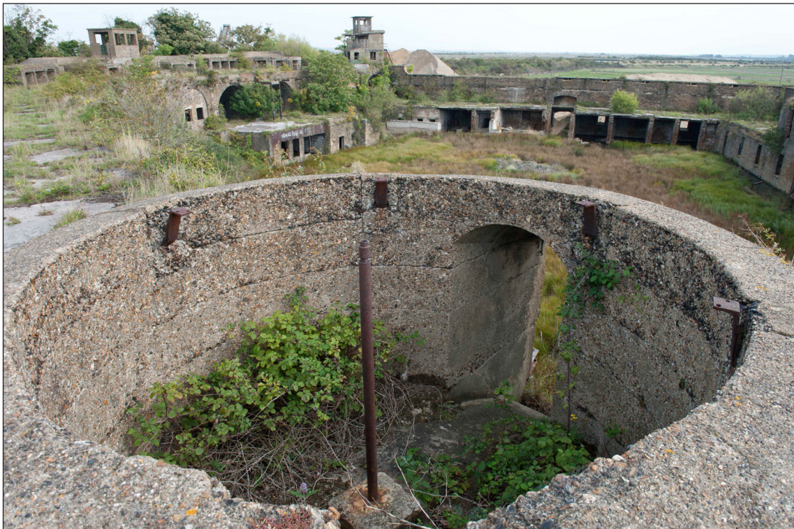
Figure 71: The interior of the collar for the rising tower looking north. The horizontal marks in the sides of the cone mark successive pours of concrete. The steeply sloped ramp between the interior of the cone and the opening in the gable end of the earlier observation position can be seen on the right hand side of the picture. The rod set in the centre is thought to be a mounting for a Second World War light machine gun sitting on an inserted timber floor. (DP097558)
