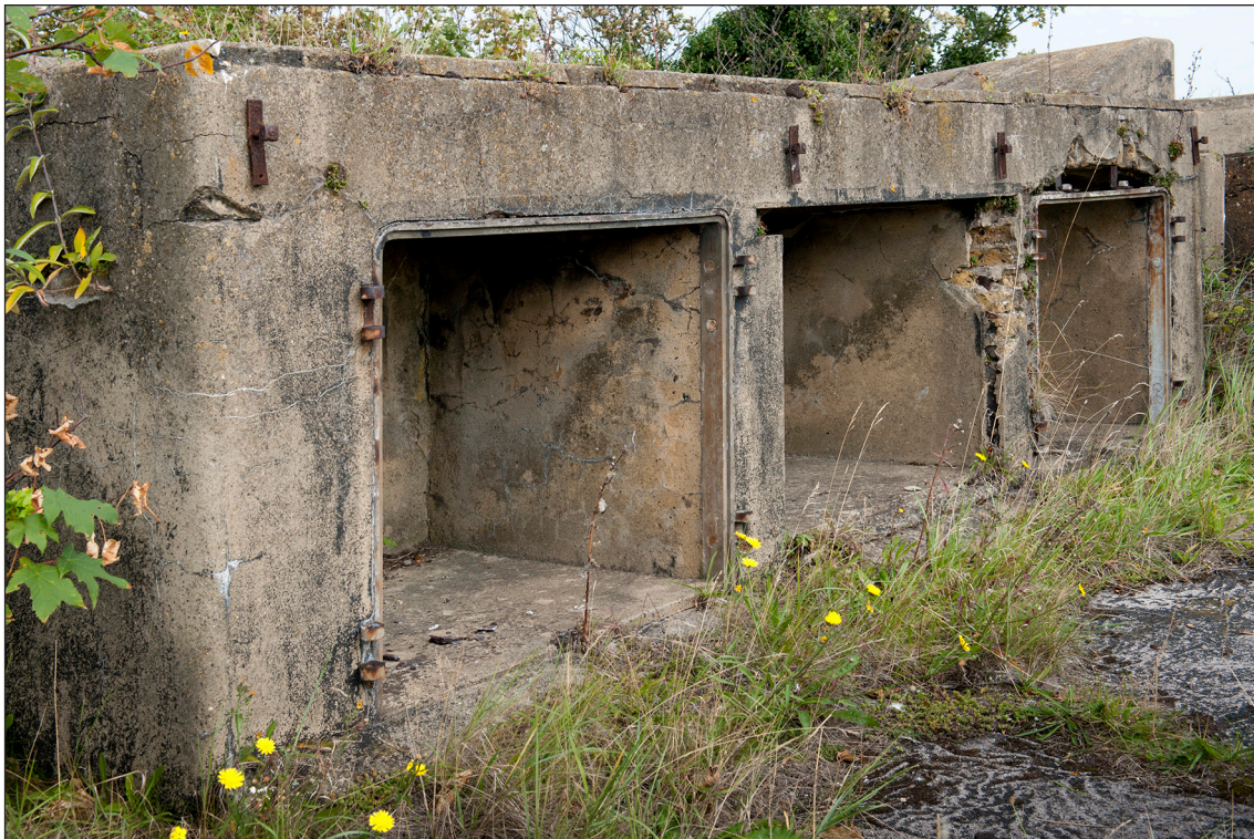
Figure 52: Ammunition lockers associated with the western 6-inch gun position. Hinges for doors on the two flanking cartridge lockers are visible as well as bolts that carried a rain hood above all three lockers. (DP097746)
