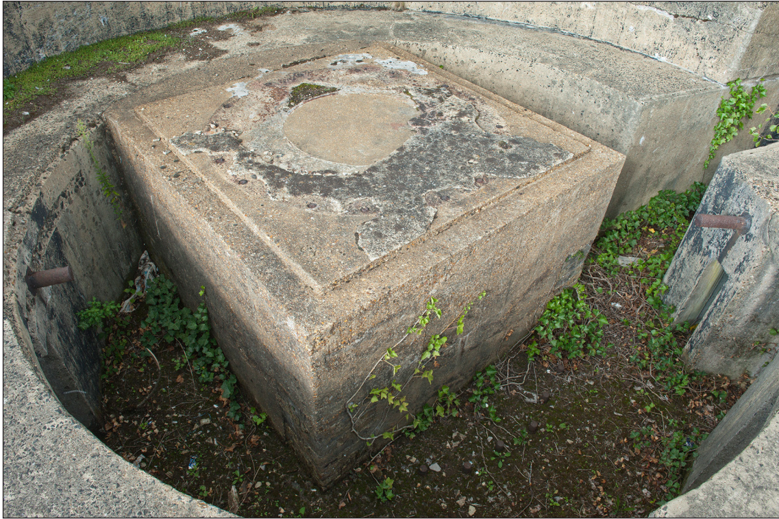
Figure 79: Concrete block inserted to modify the 6-inch gun emplacements during the Second World War. (DP097671)
