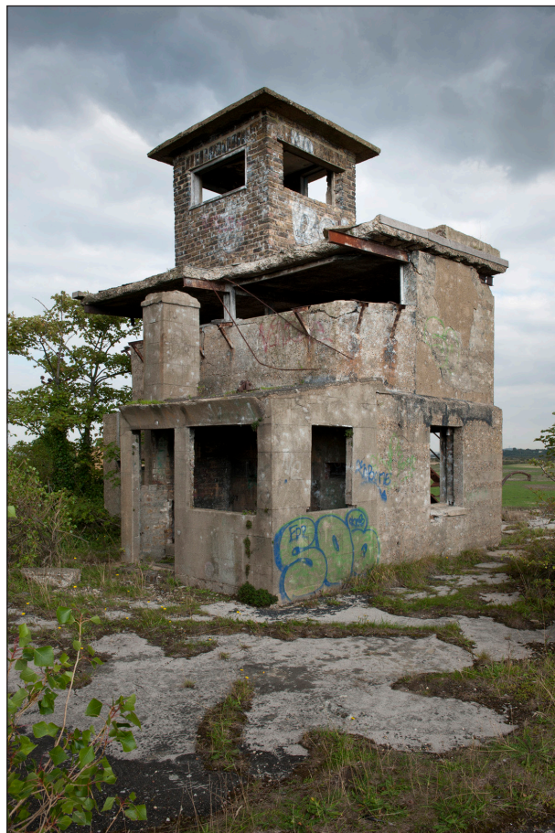
Figure 53: The Battery Observation Position looking east. The chimney stack of the projecting single-storey structure obscures the view from the observation slits. The hut on the roof dates from the Second World War. (DP097671)
