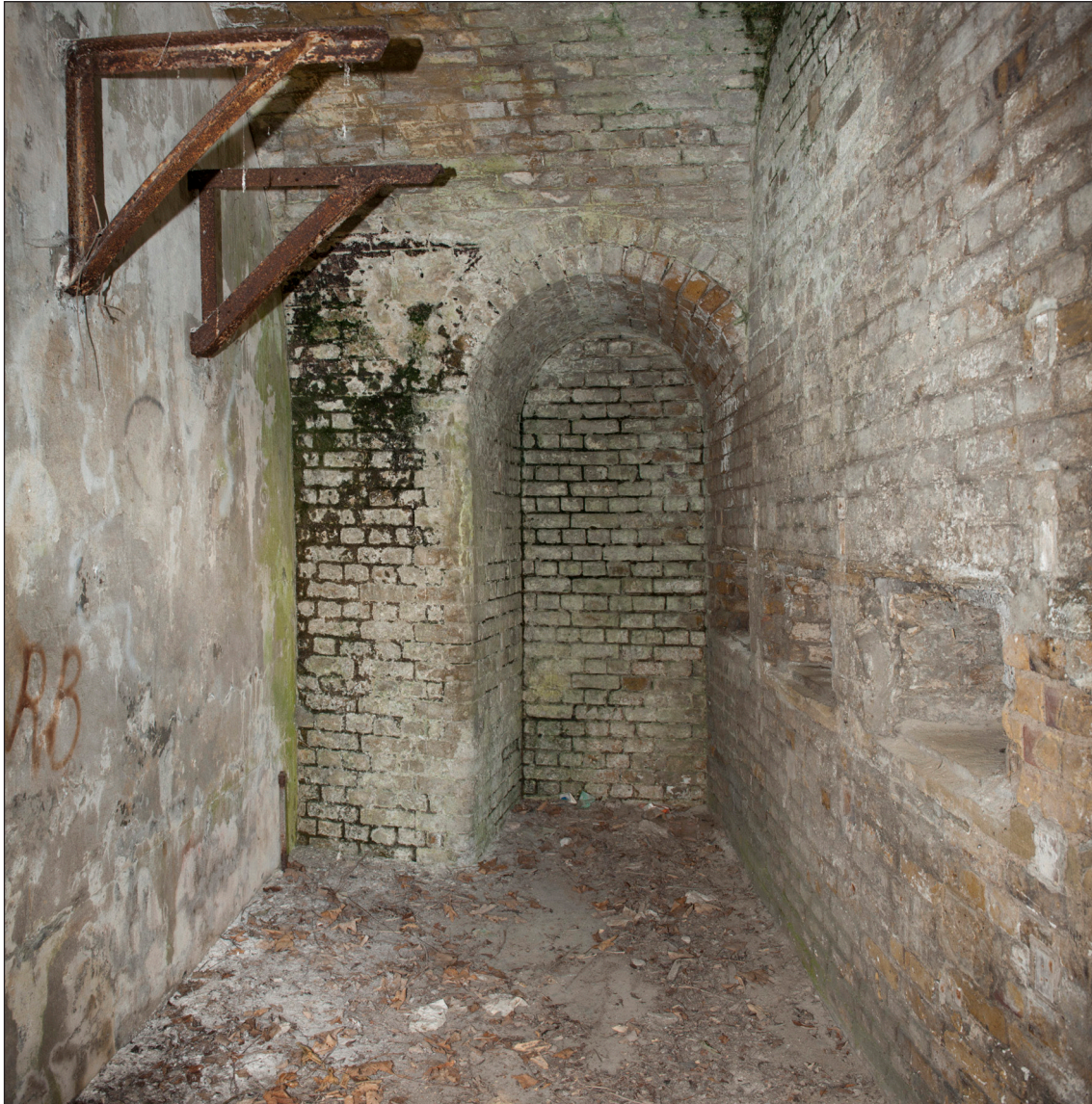
Figure 42: The south-east corner of Casemate 1. To retain access to the loopholes in the bastion wall on the right-hand side of the picture this corner of the casemate was not filled with concrete when the rest of the position was converted to a traverse. The smooth concrete wall of the traverse is on the left-hand side (the brackets are later additions). (DP097610)
