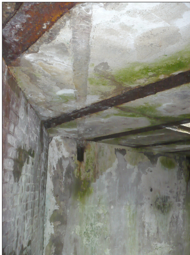
Figure 61: The interior of the north gun position of the former open battery looking west, showing the position of the pulley beam for the original south slipway. The cut off end of this beam is visible as a dark coloured square in the wall with a corresponding witness mark running along the ceiling.
