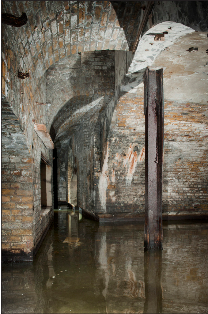
Figure 68: The former lighting passage running at the rear of the Brennan Installation. The Engine Room is in the vaulted casement to the right with the later condenser tank and pumps in the adjacent casemate, the entrance to which is just visible at the end of the passage. The rectangular recess visible in the wall on the left side may be connected with the support for the engine steering beam. The manhole that opens into the former open gun emplacement above is in the cut out section of the lighting passage vault. (DP 097528)
