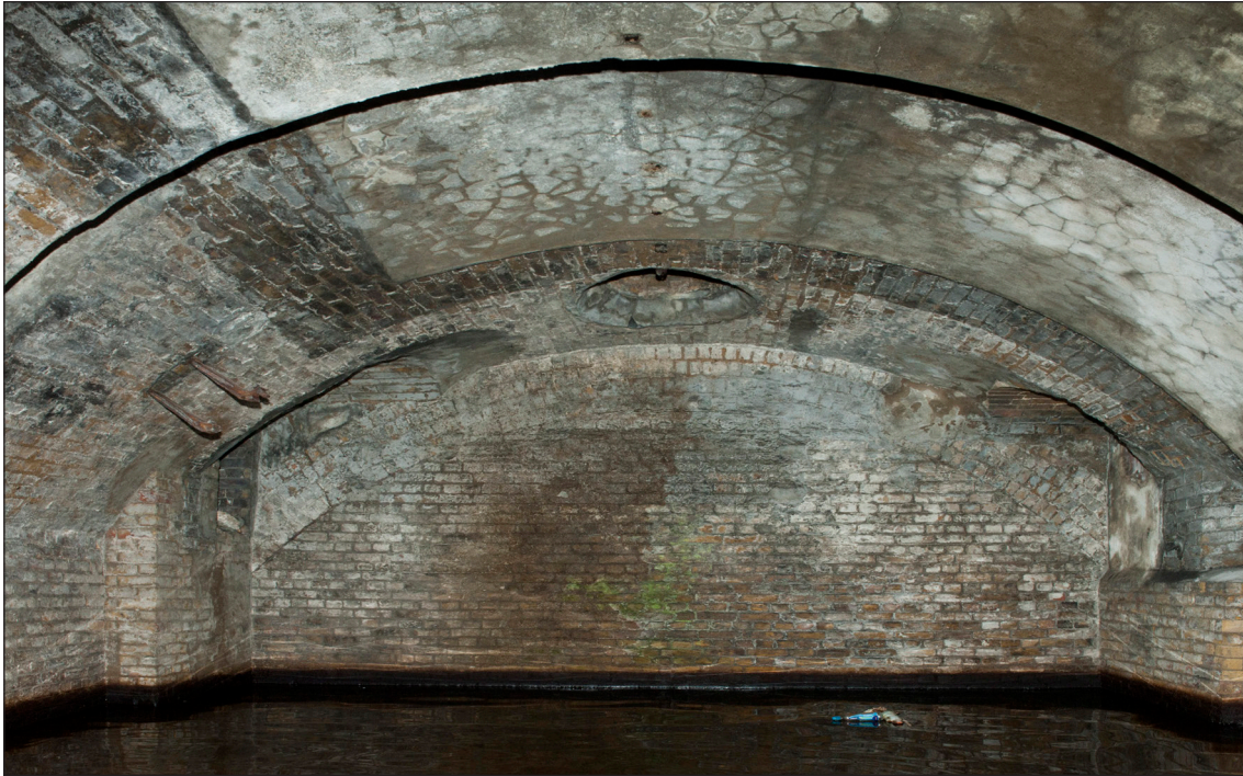
Figure 62: The interior of the former boiler room and oil store looking west. The scar of the removed wall between the ammunition store and the shifting passage is visible on the vault along with the shaft for the ammunition lift to the former open battery. The brick piers beneath the vaulted openings to the blocked shifting passage are the remains of the base and flues for the Cornish boilers. (DP 097540)
