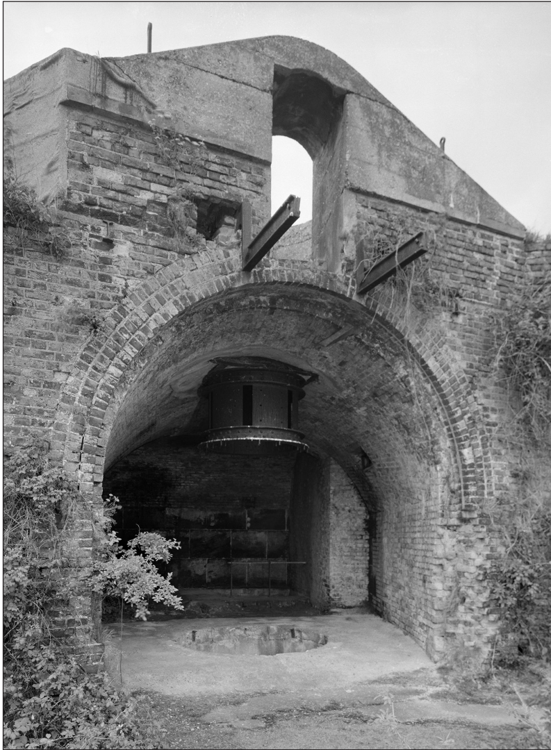
Figure 66: The gable end of what was probably the original Brennan observation position above Casemate 15. The later concrete cone for the rising tower installation appears to have engulfed the earlier handrail stanchions. (bb93_20789)
