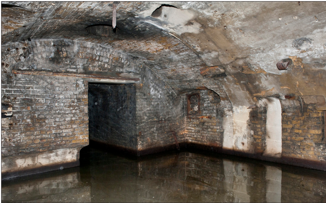
Figure 64: The interior of the Engine Room looking west. The entrance to the Torpedo Store is in the centre of the frame and to its left is the segmental head for the entrance to the caponier. In the vault, and surrounded by light coloured concrete, is the shaft pierced for the driving wire to the north slipway. The projecting iron strap is possibly a support for a pulley wheel. The deep recess at the foot of the wall on the left marks the course of the sea water supply pipes to the surface condenser. On the right the blocked arched headed opening for the shifting passage has a metal framed opening for a flue rodding point inserted in its centre. (DP097535)
