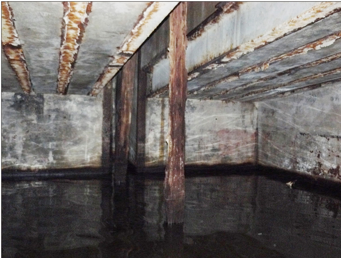
Figure 60: The interior of the Torpedo Store looking west and showing the slope of the roof to accommodate the top of the south launching slipway. The vertical timbers in the foreground mark the course of the torpedo handling slot © Wayne Cocroft
