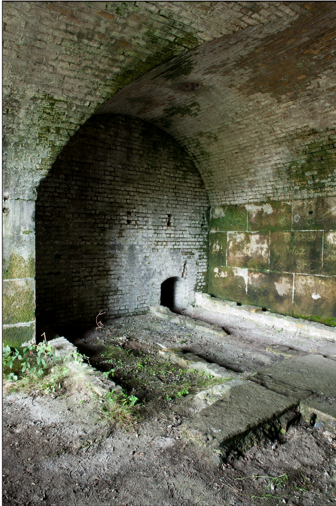
Figure 69: The southern wall of Casemate 15 showing the low tunnel that may have been inserted to enable the installation of the machinery for the rising tower. (DP097642)
