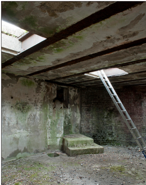
Figure 67: The opening for the north slipway pulley beam in the concrete block that occupies the embrasure of the former northern open gun position. It is located just below the ceiling with the securing studs for a pulley and the shaft leading down to the Engine Room on its left side. On their right is the short flight of concrete steps for access to the pulley beam. (DP097783)
