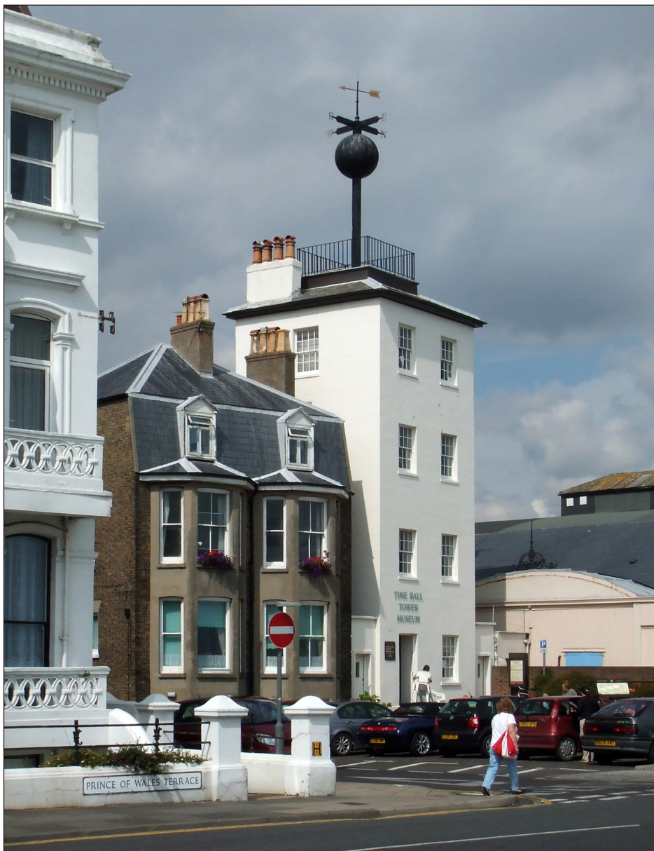
Fig. 7: The former semaphore tower, with its time ball, at Deal. DP026931 © Historic England Archive
