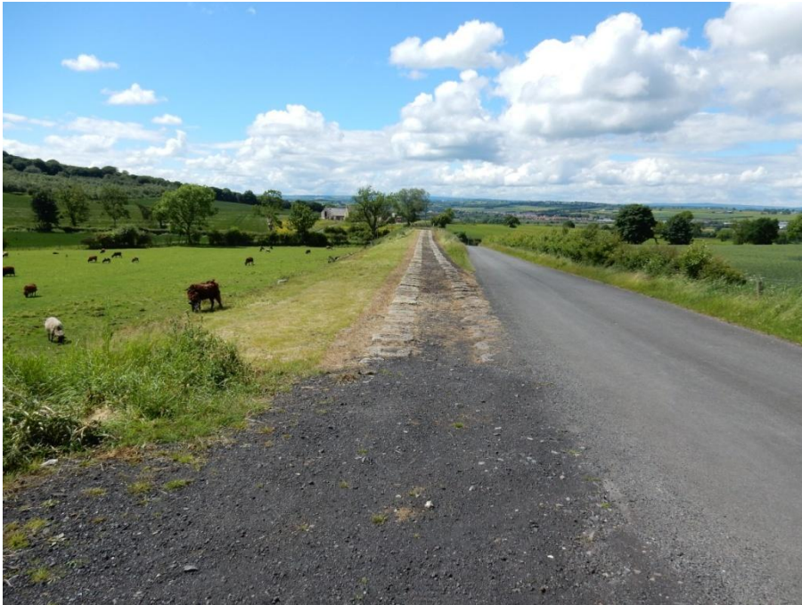
Stone blocks were commonly used to support cast- or wrought-iron rails, as in this view of the Brusselton incline on the Stockton & Darlington. © Julia Elton
