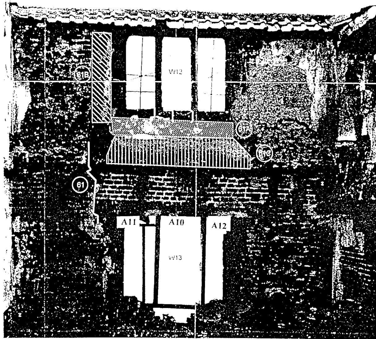
Figure 3c: Drawing to show positions of samples FAW-A10, A11 and A12 from window 13 in the south wall
