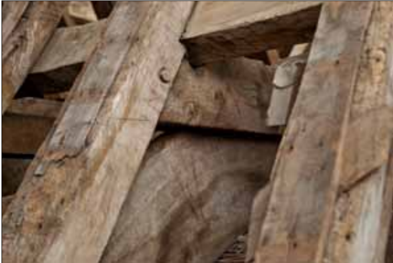
Fig 2.1 Red carpenter's marks to roof over H2.10/2.12.
