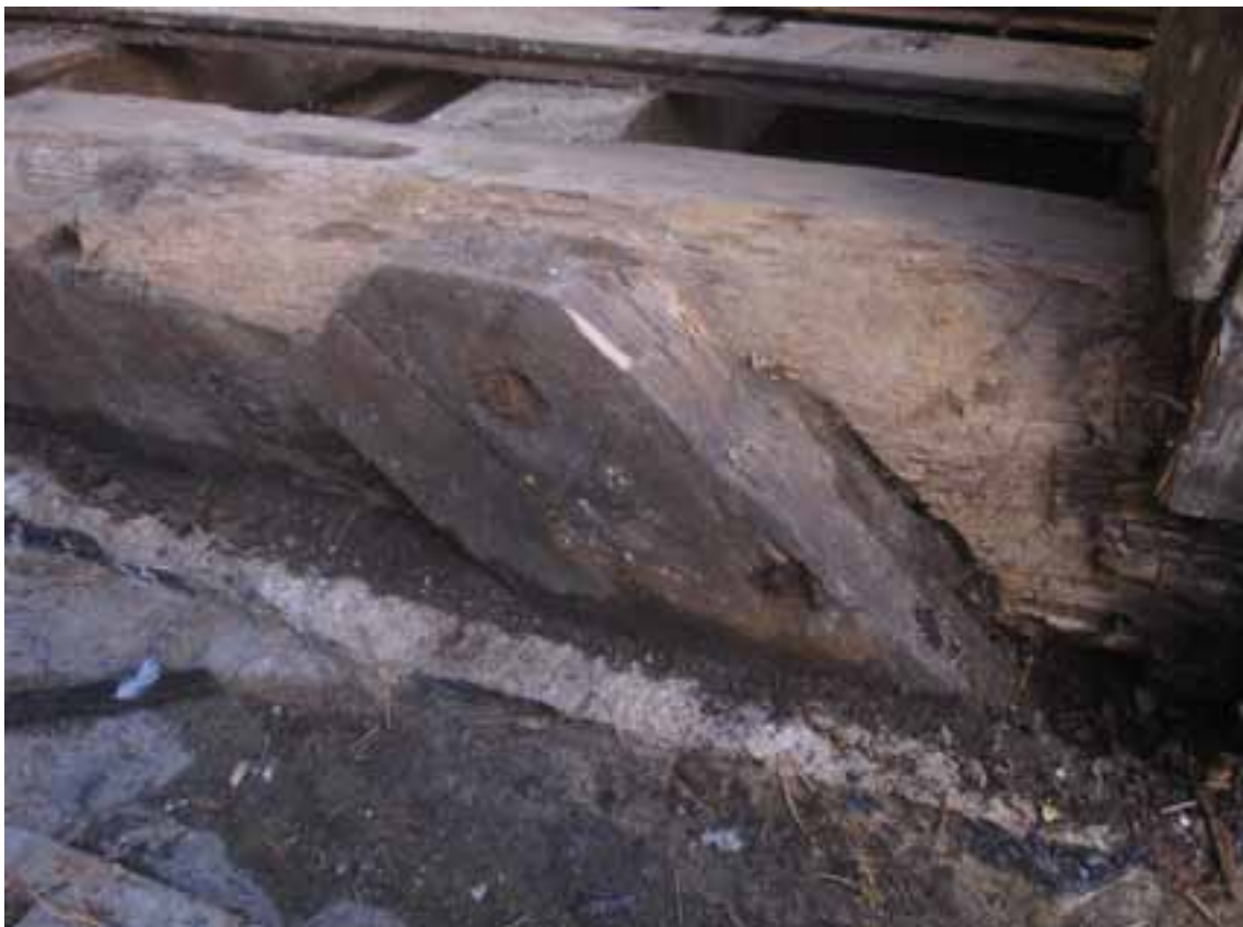
Fig 4.3 Detail of raking brace, fixed with nails.
