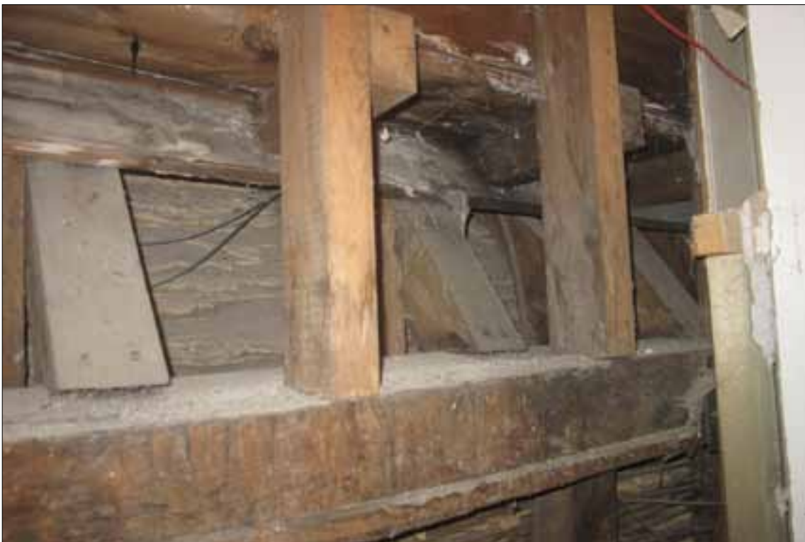
Fig 8.4 West wall of H2.16, north end.
