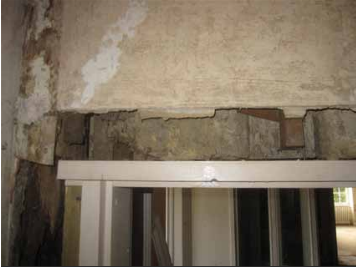
Fig 3.5 Detail of studs and mud infill panel over doorway.
