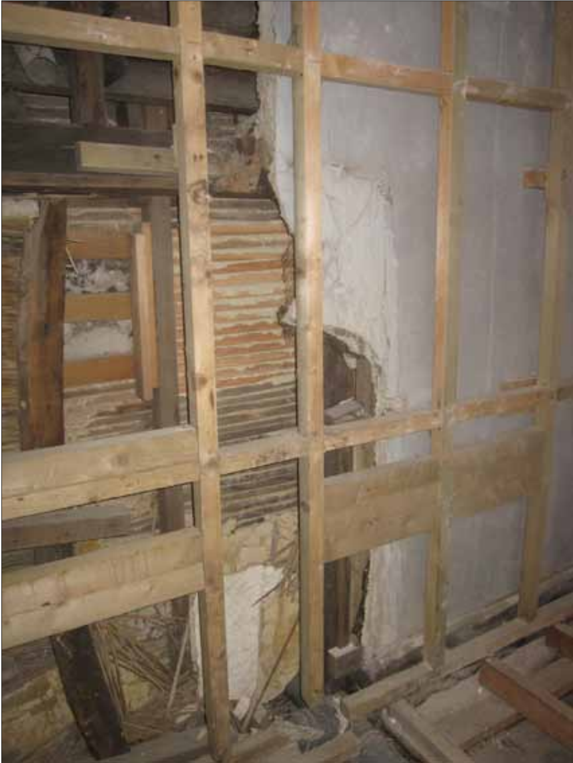
Fig 8.2 West wall of H2.16, centre.
