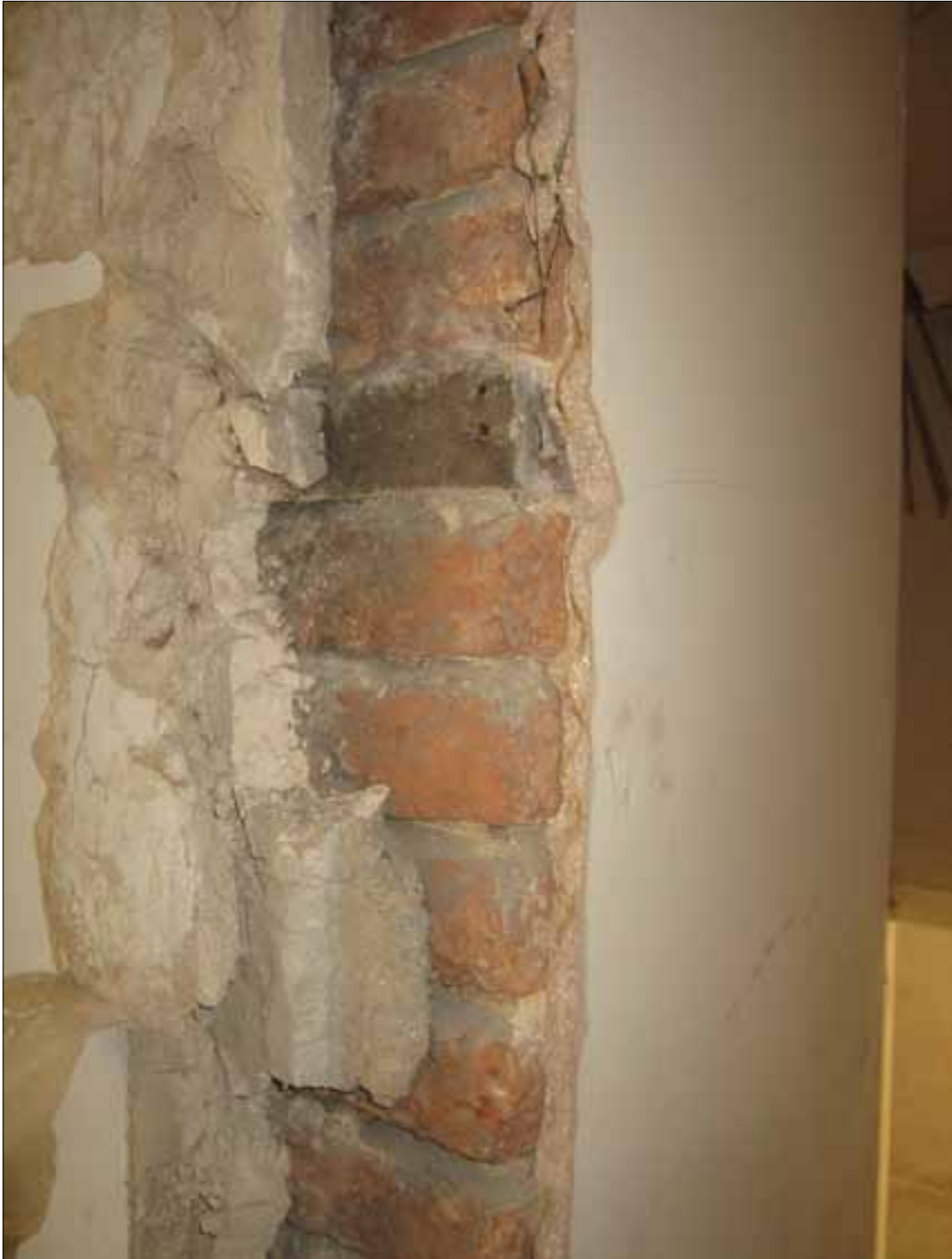
Fig 6.2 Detail of brick door jamb.
