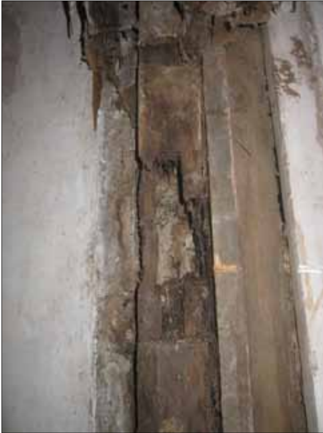
Fig 3.3 Side view of mortice for doorway lintel.
