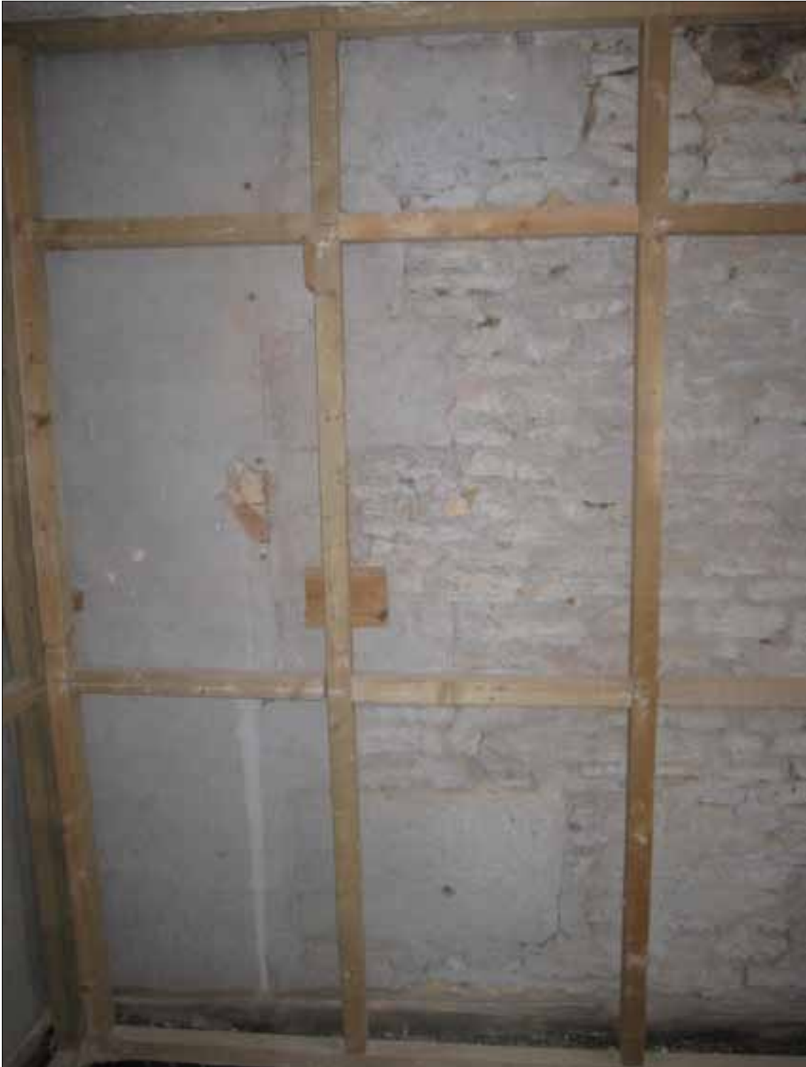
Fig 7.2 Stone quoins to north wall of H2.16
