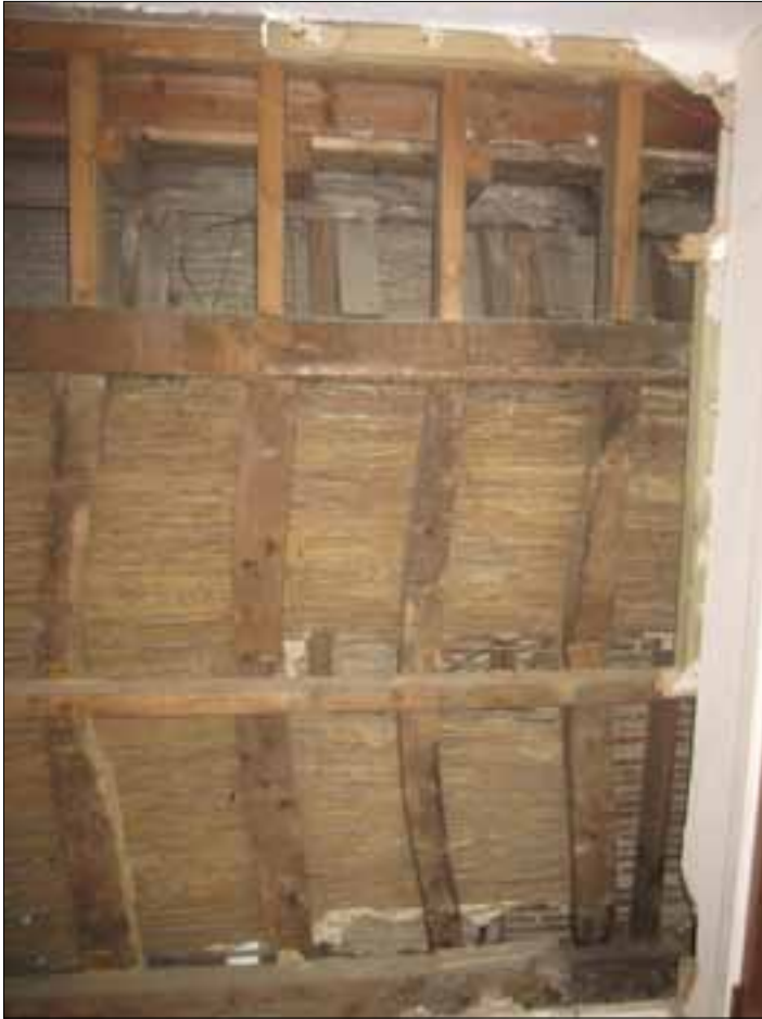
Fig 8.3 West wall of H2.16 - wallplate.
