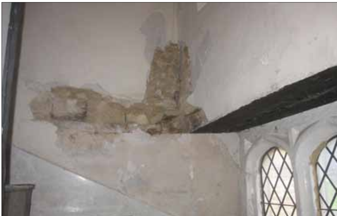
Fig 9.1 Junction of south and east walls to H2.14 stair.
