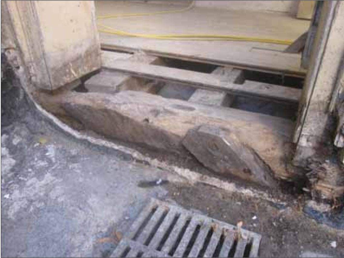
Fig 4.2 Oak cill with raking brace.
