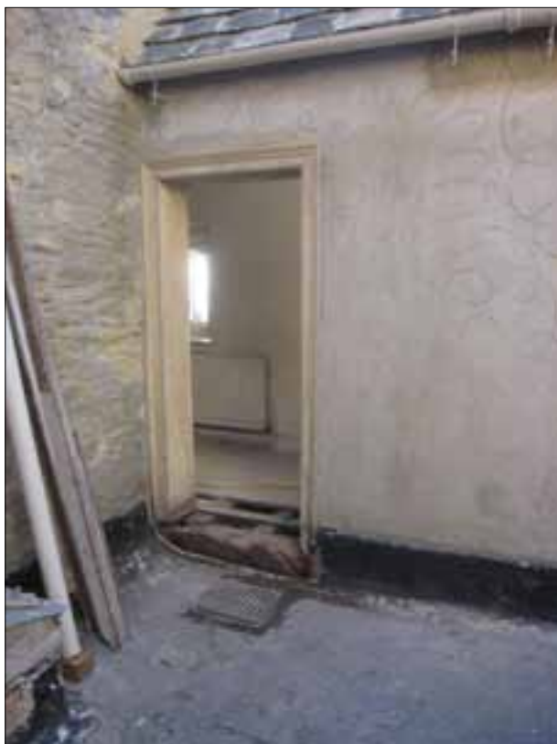
Fig 4.1 View of doorway off H2.05a.
