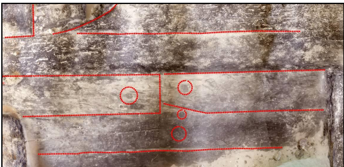
Figure 21: Close-up of a section of exposed planking in Area 3 © PAS.
