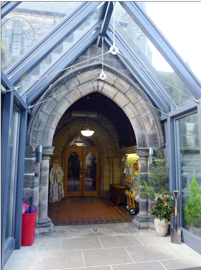
Figure 40: Glazed corridor linking church porch with the later parish centre at the Church of St Margaret, Horsforth (© Historic England, photograph: Clare Howard)
