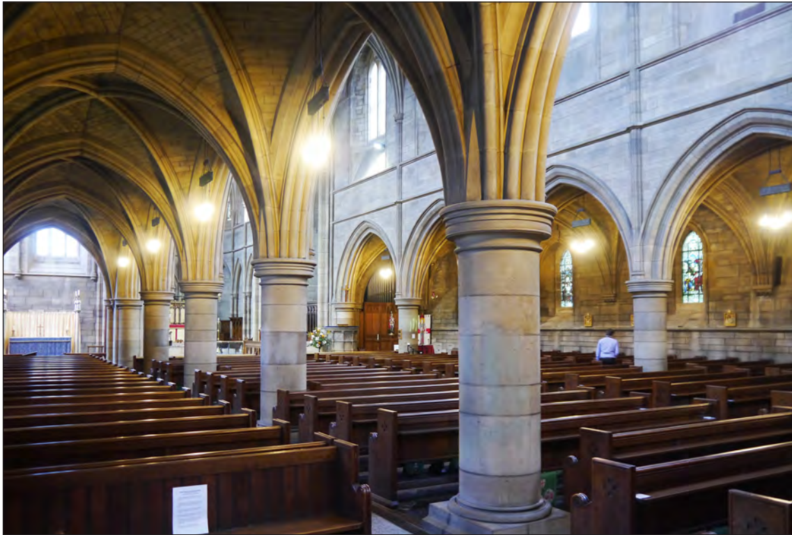
Figure 101: View from the north aisle of the Church of St George, Cullercoats, (© Historic England, photograph: Simon Taylor)
