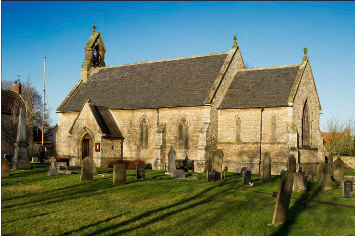
Figure 44: The Church of St Anne, Ellerker, taken from the south-east (D168569 © Historic England, photograph: Alun Bull)
