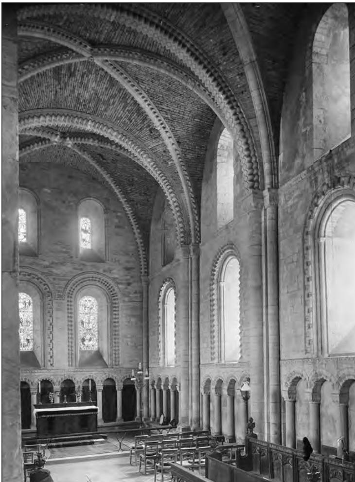
Figure 10: The chancel at St Mary's, Stow, taken from north-west circa 1920-60 (CC83/00752 © Historic England Archive)
