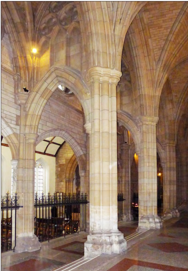
Figure 22: Stone vaulting between the chancel aisle and the incorporated St Mary's Aisle at Truro Cathedral (© Historic England, photograph: Clare Howard)
