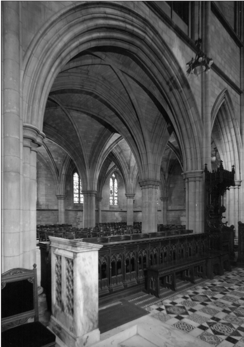
Figure 113: The north chapel of the Catholic Apostolic Church, Maida Avenue, taken from the west in 1967 (67/00904 © Historic England Archives)
