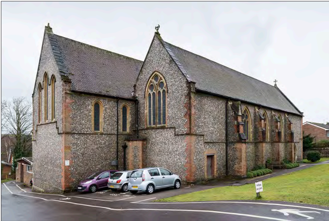
Figure 106: The Church of All Saints at Highcliffe, taken from the north east (DP172520 © Historic England, photograph: James O Davies)
