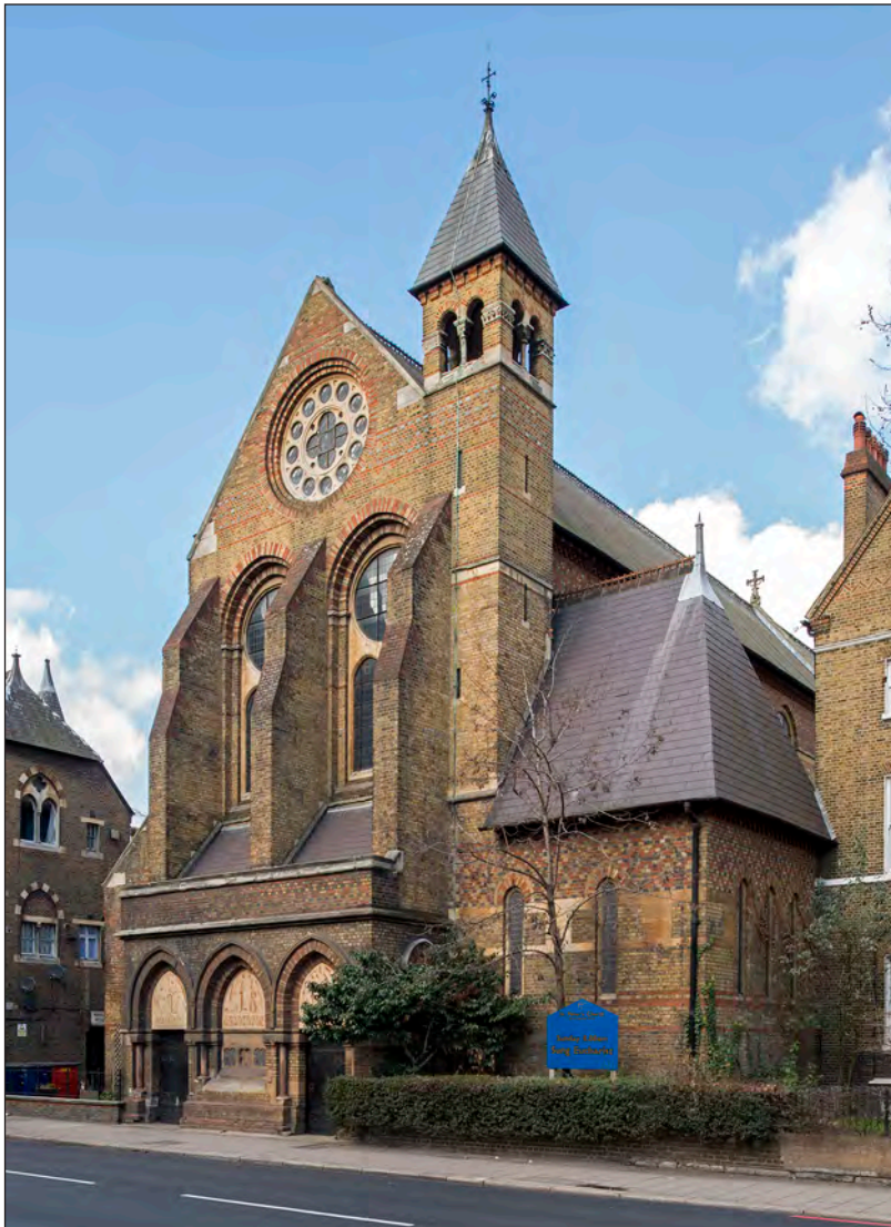
Figure 69: The Church of St Peter, Vauxhall, taken from the south-east (DP164363 © Historic England, photograph: Lucy Millson-Watkins)
