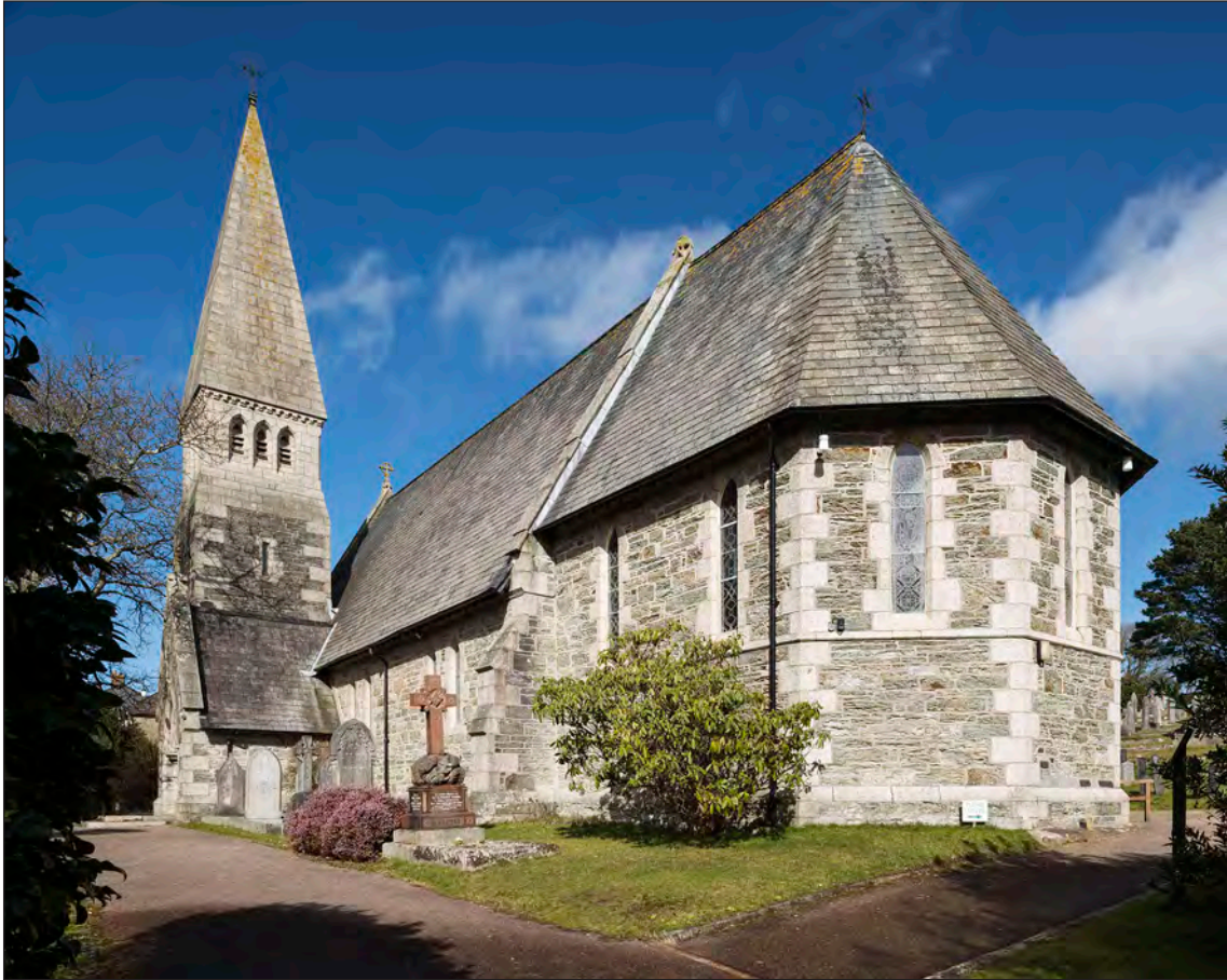
Figure 48: The Church of St John and St Petroc, Devoran, taken from the south (DP172549 © Historic England, photograph: James O Davies)
