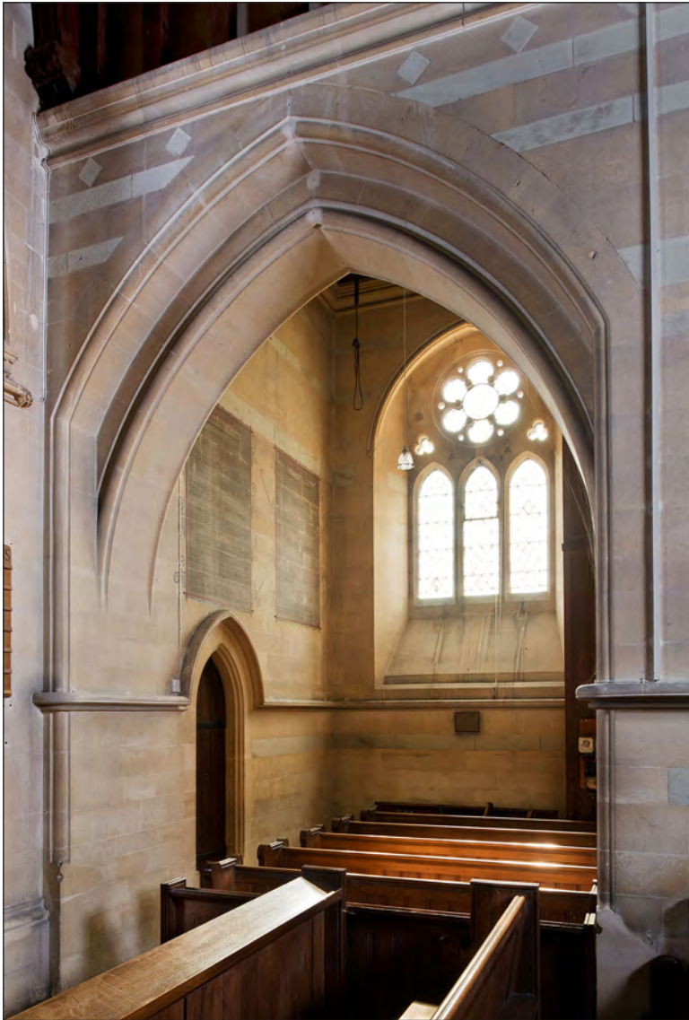
Figure 63: The south transept in the Church of St James, Titsey, taken from the west (DP167295 © Historic England, photograph: James O Davies)
