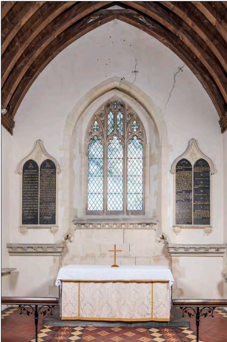
Figure 60: The chancel of the Church of St Peter, Charlton, taken from the west (DP164995 © Historic England, photograph: Steven Baker)
