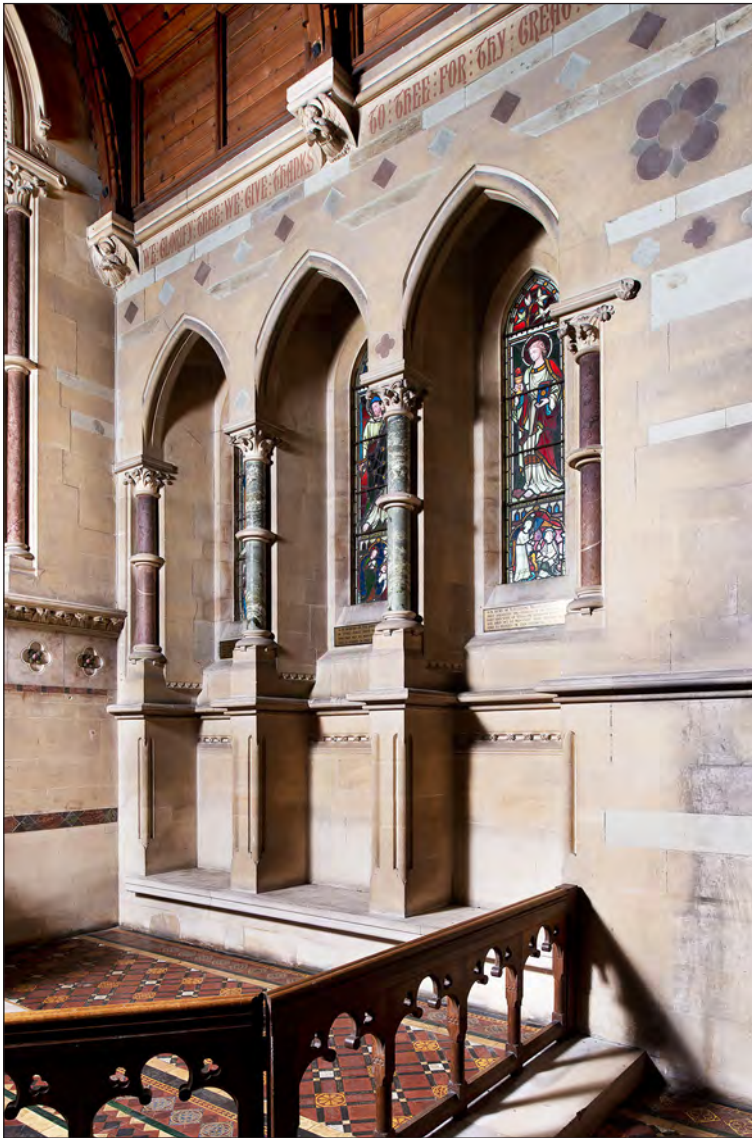
Figure 13: Constructional polychromy in the Church of St James, Titsey (D167319 © Historic England, photograph: James O Davies)
