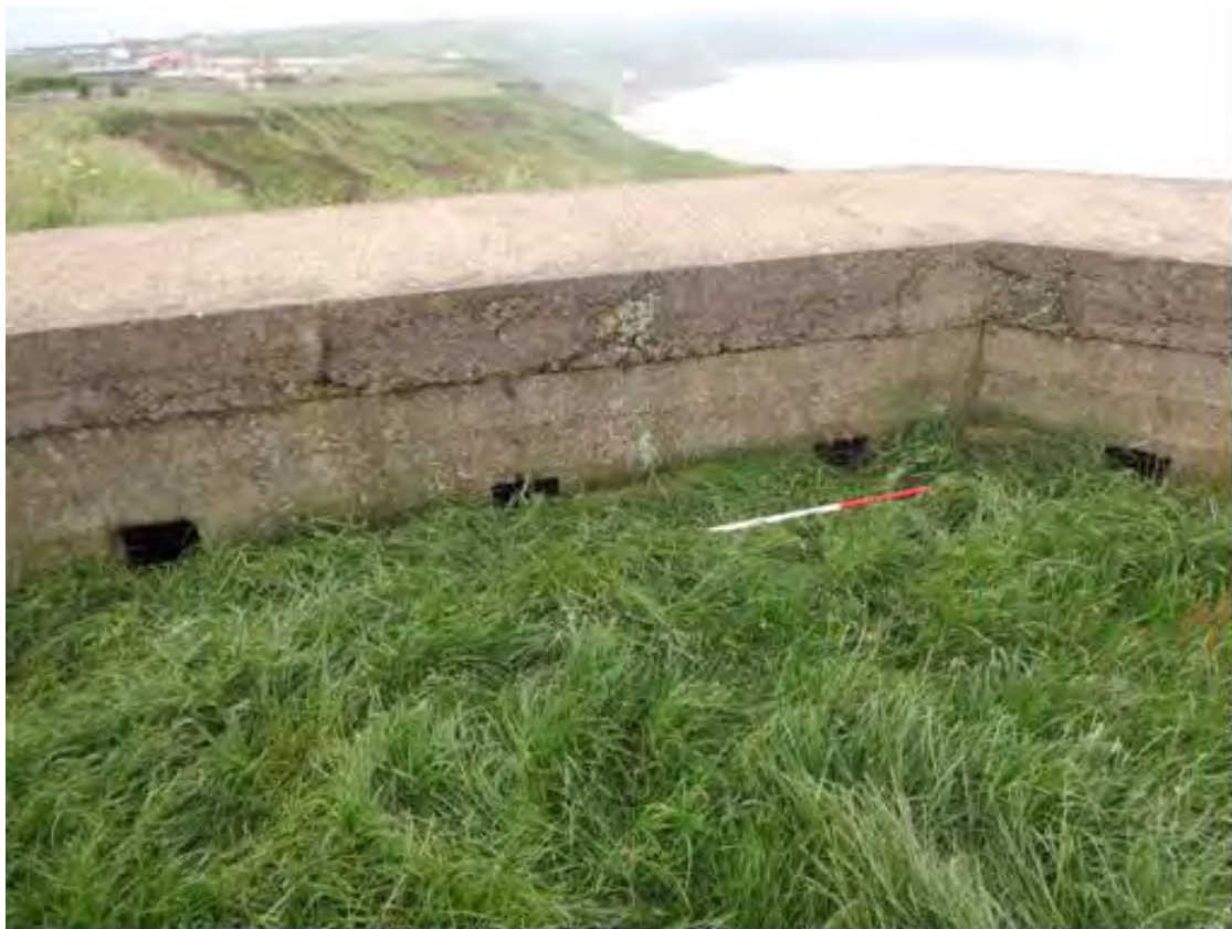
Plate 128 Second World War section post CY11, ground level gun loops in the eastern side, showing thickness of roof slab, looking north-west (1m scale)
