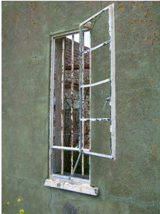
Plate 195 RAF Theddlethorpe, turret range maintenance building, detail of typical metal-framed window
