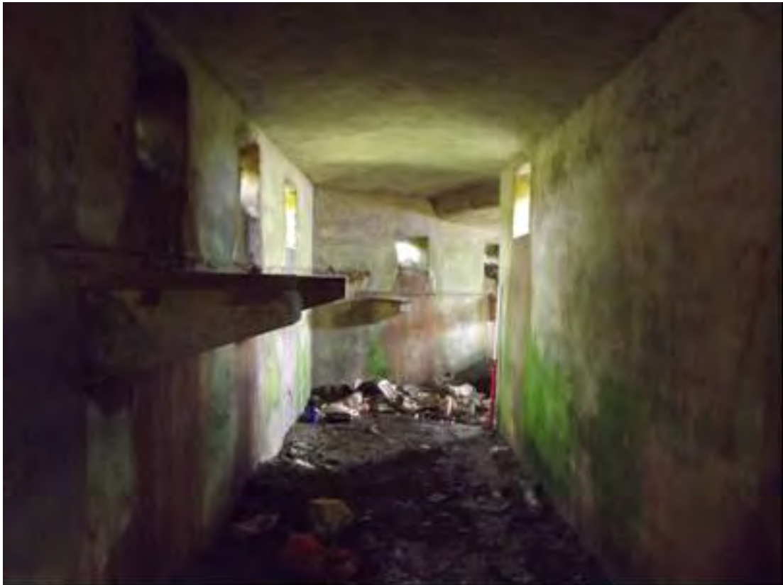
Plate 111 Second World War section post FD80, internal view looking north towards seaward end of pillbox, with step in ceiling visible at angle (1m scale)
