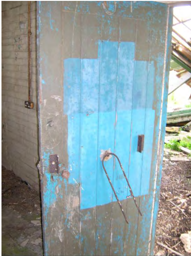
Plate 201 RAF Theddlethorpe, original door of north-west lean-to
