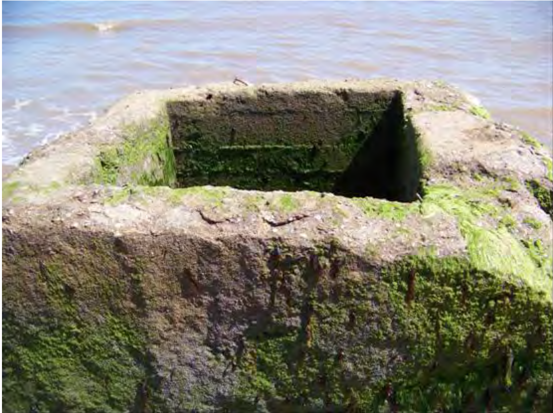
Plate 55 Inverted base of SK49, showing wall thickness and shuttering details
