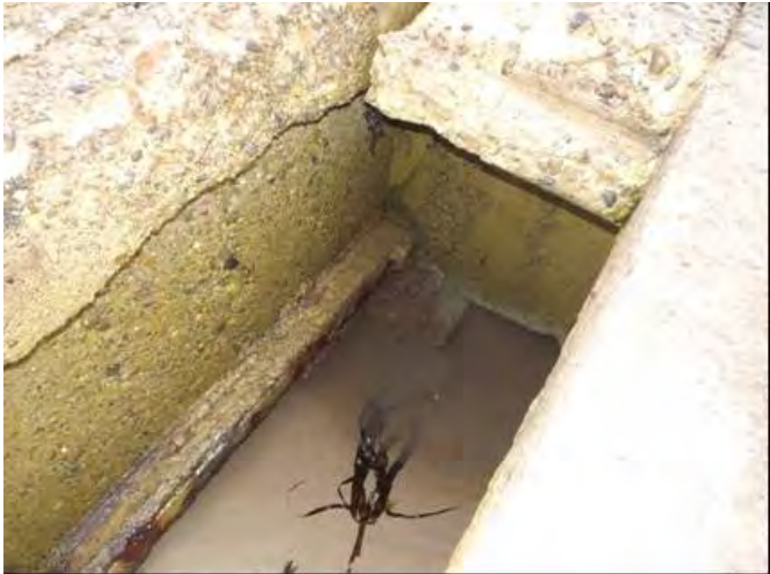
Plate 117 Second World War command/communications post OS10, cast iron beam in roof
