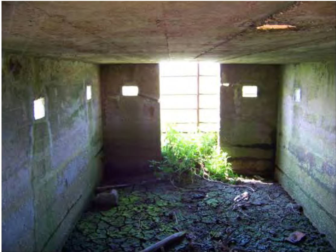
Plate 17 Interior of blockhouse BA19, showing western doorway, embrasures and impressions of shuttering on walls and roof. A ceramic vent pipe is also visible
