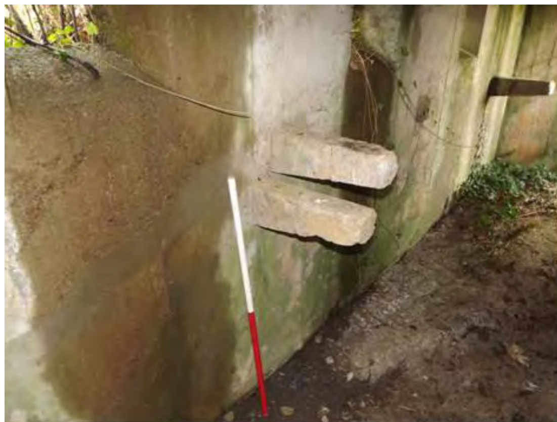
Plate 102 Second World War section post FD60, change in height of support shelf at south-western end (1m scale)
