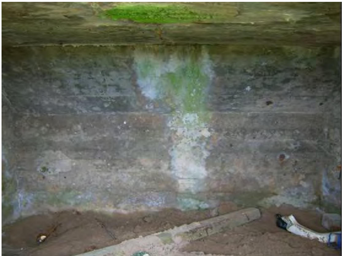
Plate 86 Interior of front wall, SH1, showing batter of upper section
