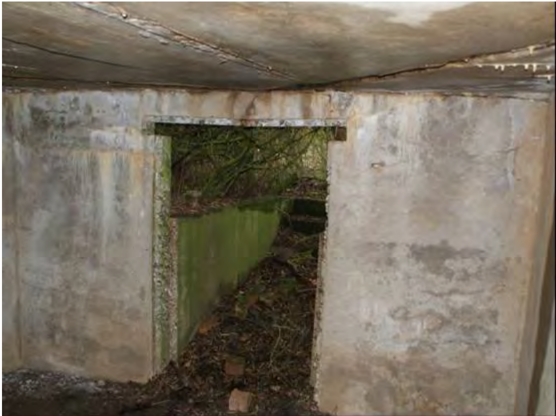
Plate 71 Interior of EG27, showing angled girders across corners of the ceiling and the void left by the salvaged doorframe
