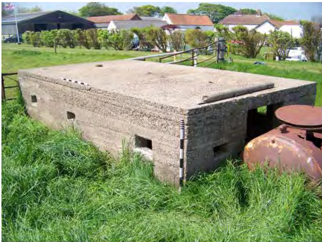
Plate 13 Blockhouse BA19, showing doorway in east wall, three roof vents and impressions of shuttering, looking north-west. (2 x 1m scales)
