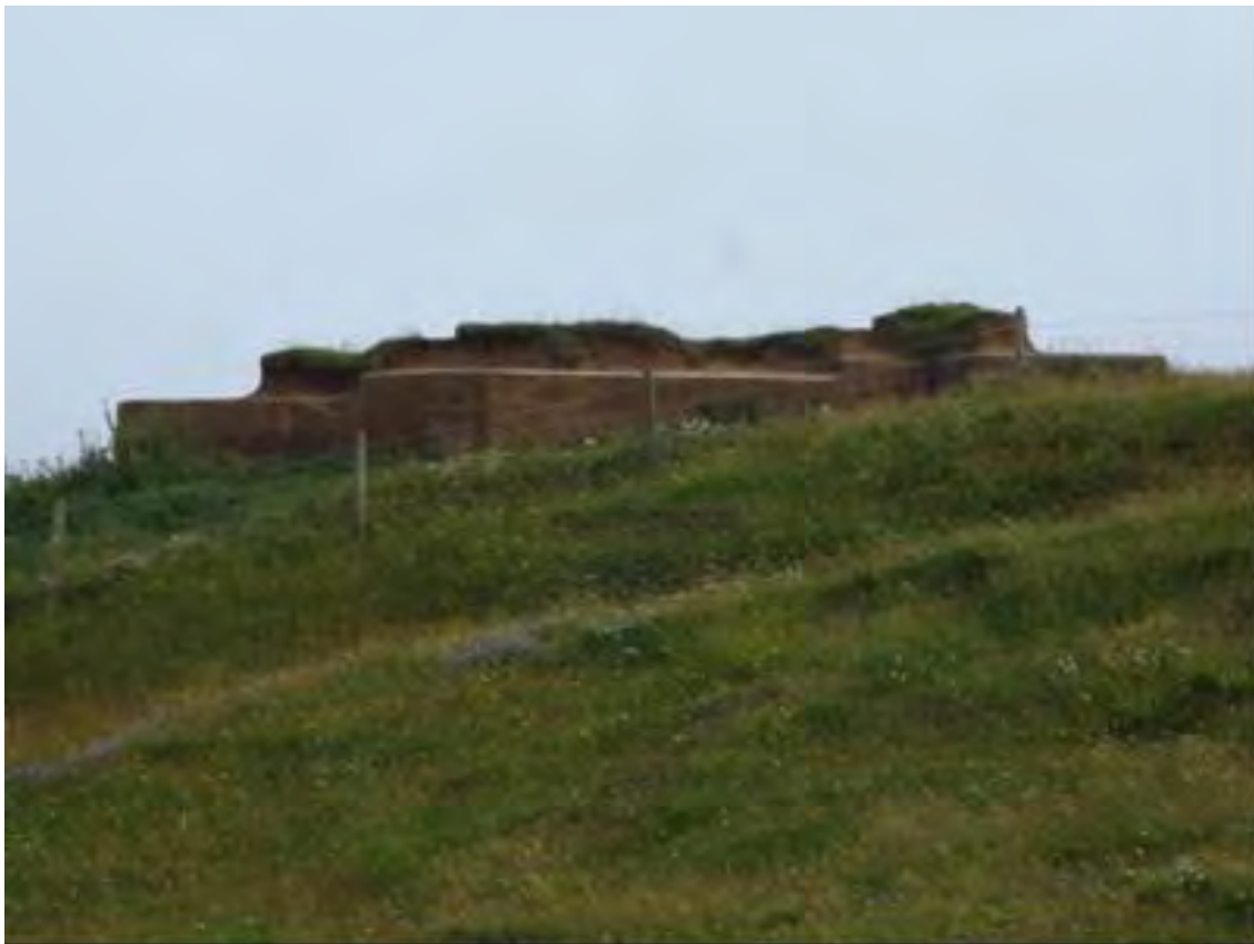
Plate 108 Second World War section post FD80, general view, looking east
