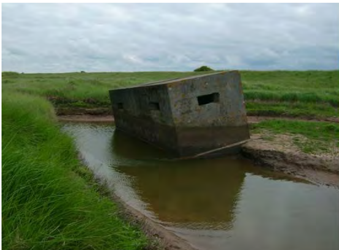
Plate 156 Second World War Lincolnshire-variant pillbox NS59, view of north and east walls, showing embrasures of twin blockhouses at ends
