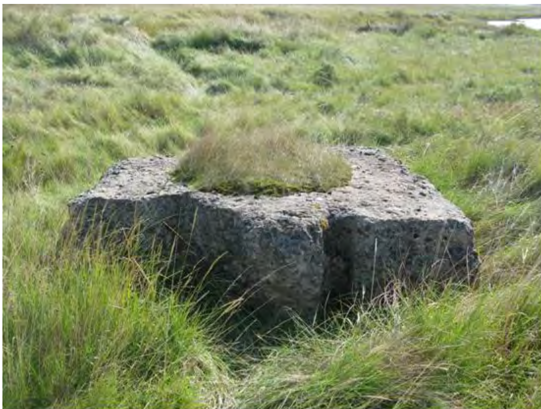
Plate 74 Roof fragment of NS65 in 2009, showing vertical impression of vent pipe
