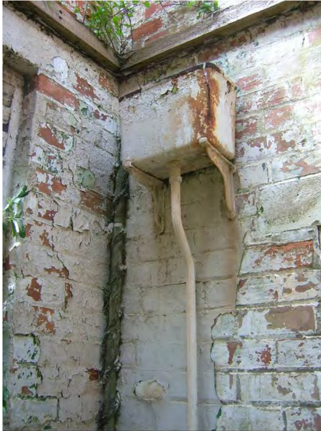
Plate 199 RAF Theddlethorpe, possible post-war overhead toilet cistern
