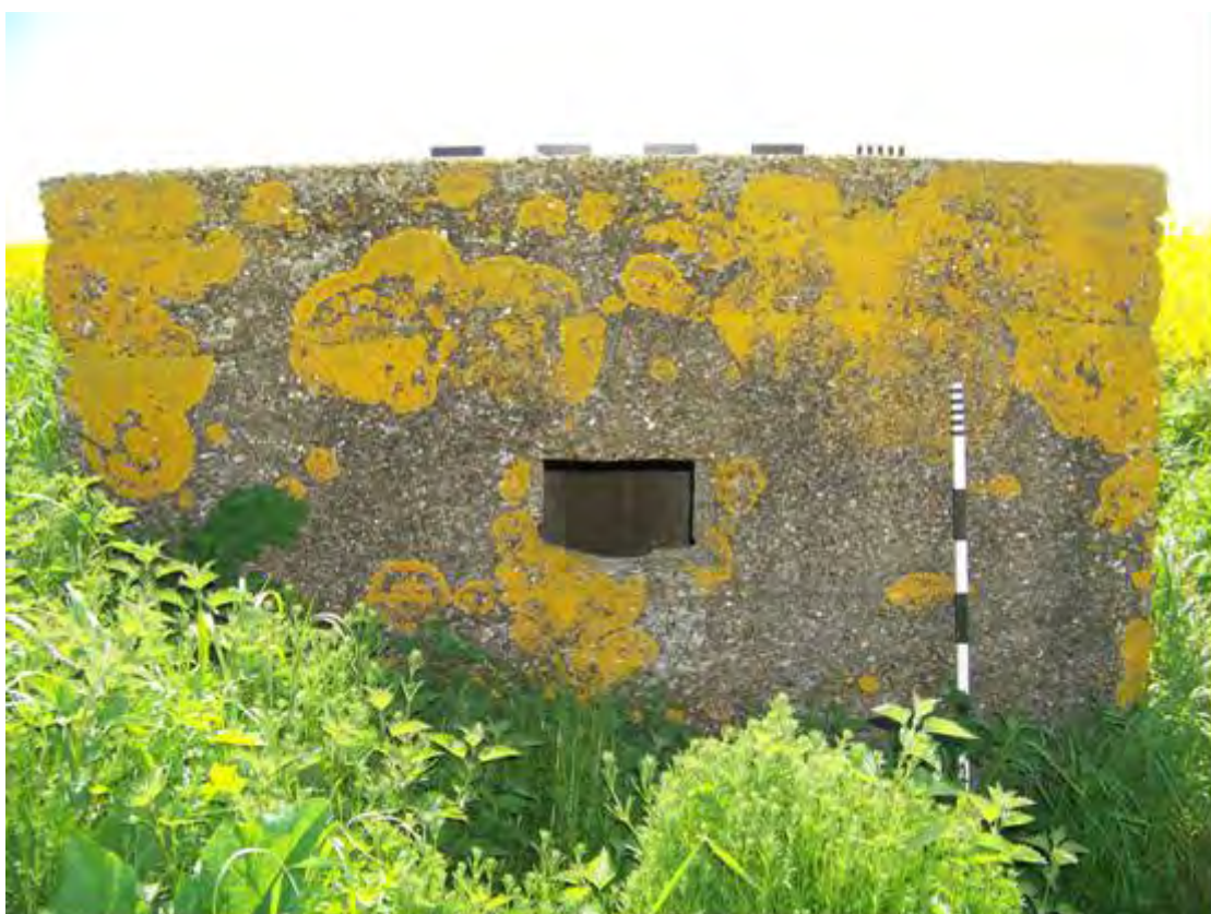
Plate 36 Pillbox BA74, showing embrasure in east wall, looking west along hedgerow (2 x 1m scales)
