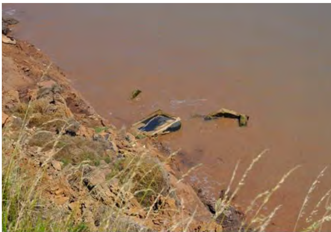
Plate 174 Second World War Ringbrough Battery, Aldbrough (AL55), collapsed remains of southern magazine, looking north-east
