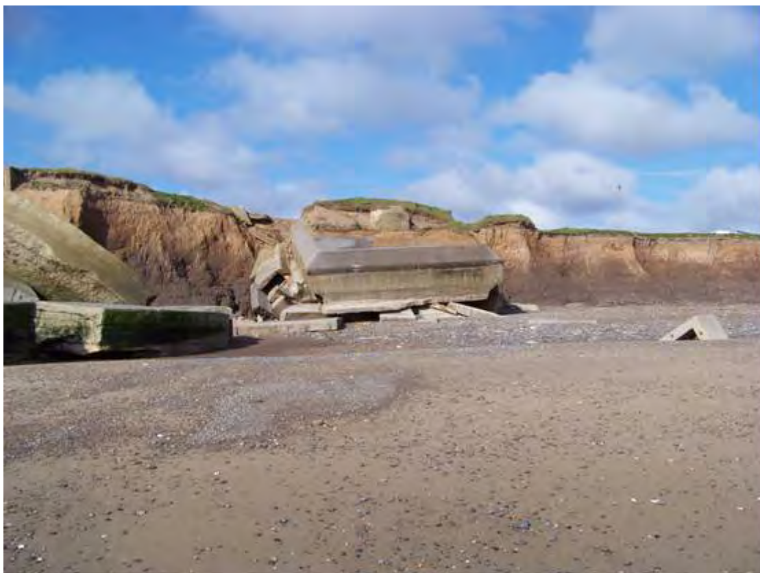
Plate 184 Godwin Battery, Easington (EA182), remains of northern magazine, looking west
