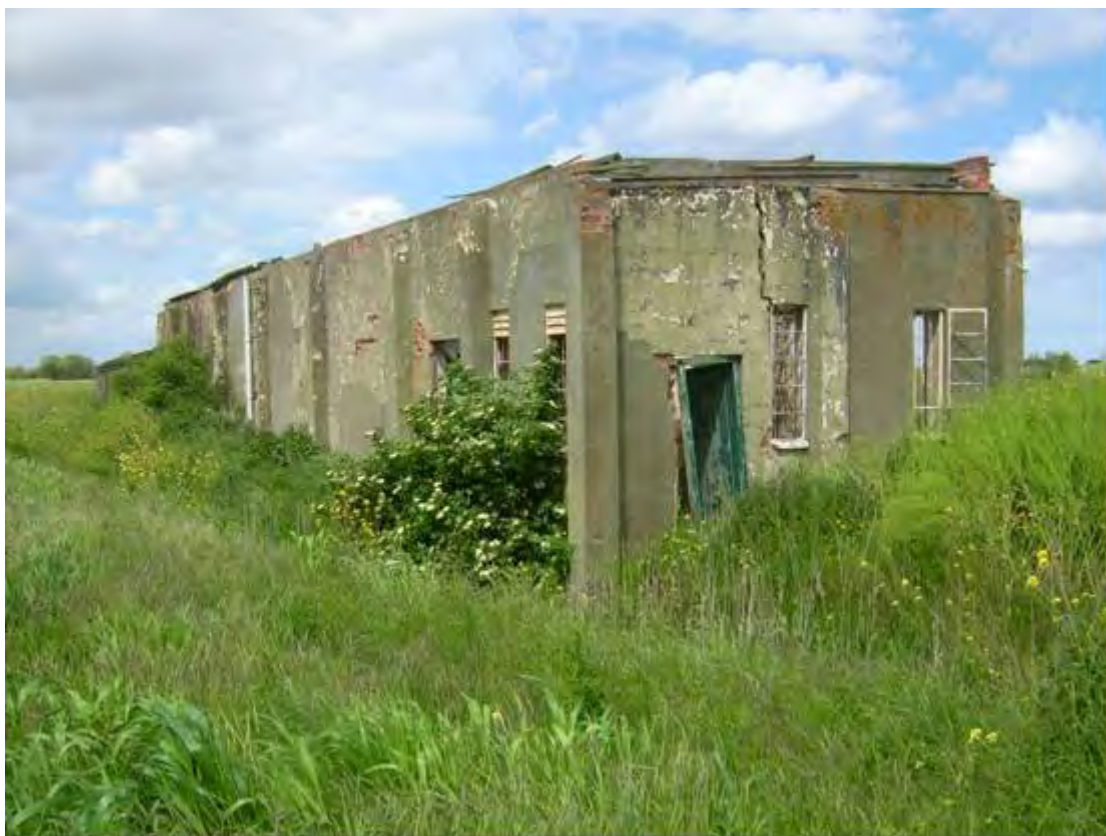
Plate 190 RAF Theddlethorpe, rear and south wall of turret range maintenance building, looking north-east
