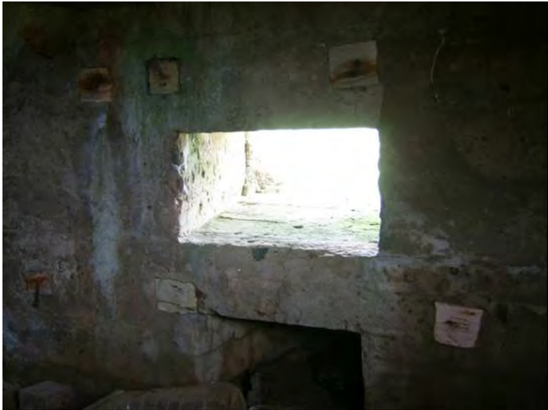
Plate 85 SH1, interior of embrasure, showing built in storage locker below, evidence of plank shuttering and wooden pads which probably mark scaffold support positions
