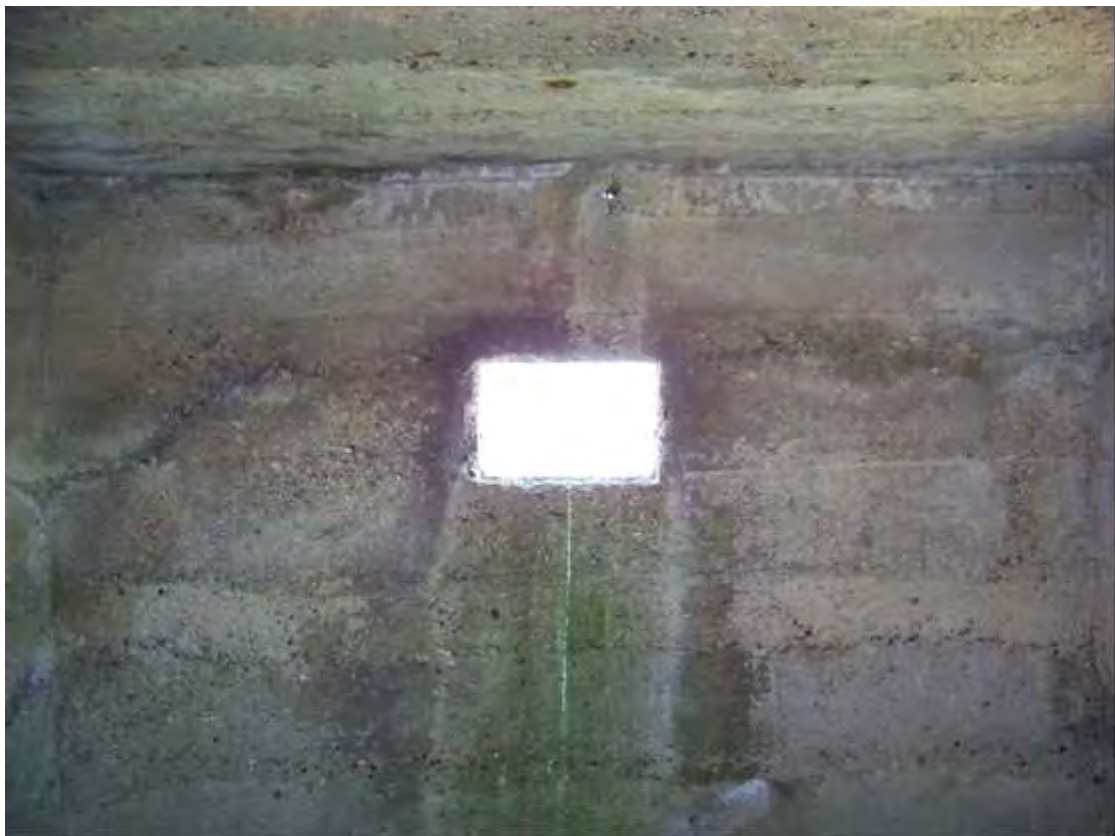
Plate 60 Interior of SK50 showing very small embrasures in this pillbox
