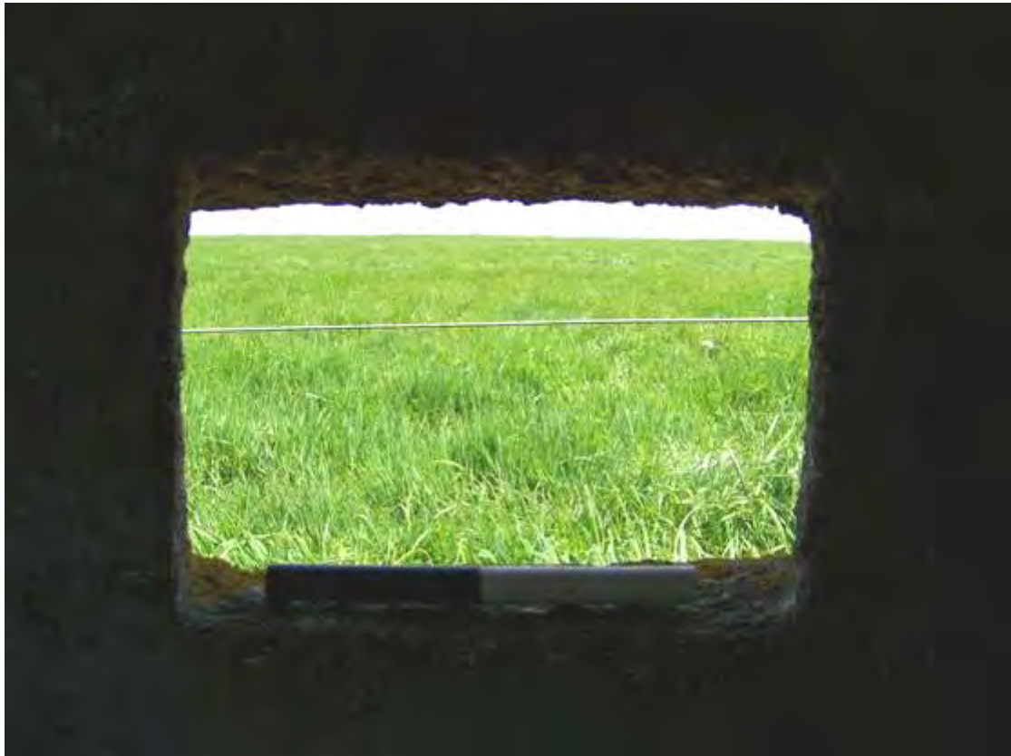
Plate 33 Interior of embrasure, BA30, showing restricted view ( 0.2m scale)
