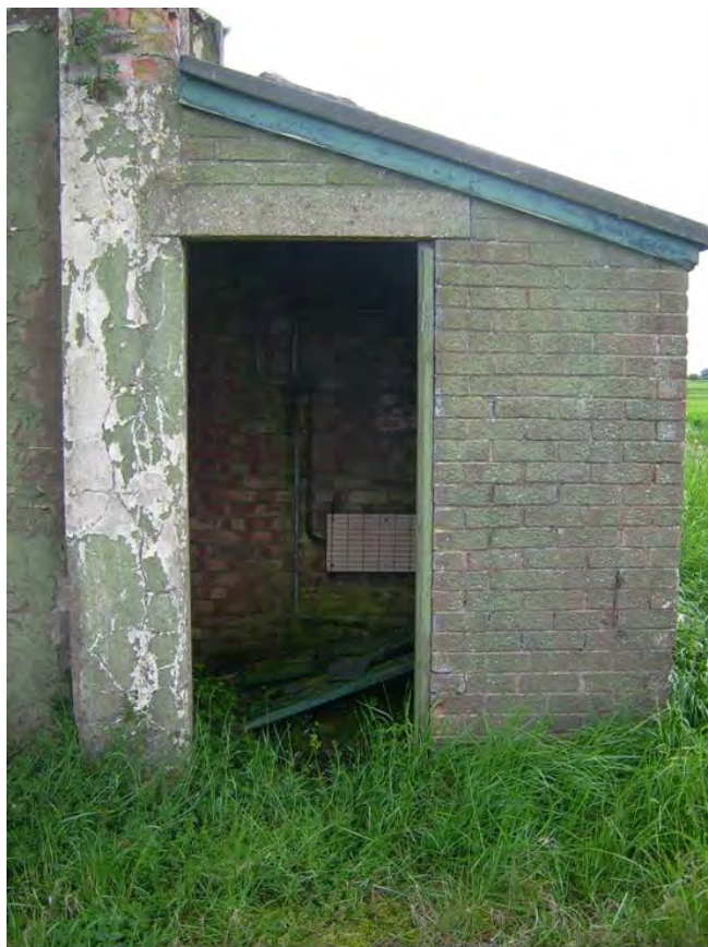
Plate 200 RAF Theddlethorpe, small lean-to, north-west corner
