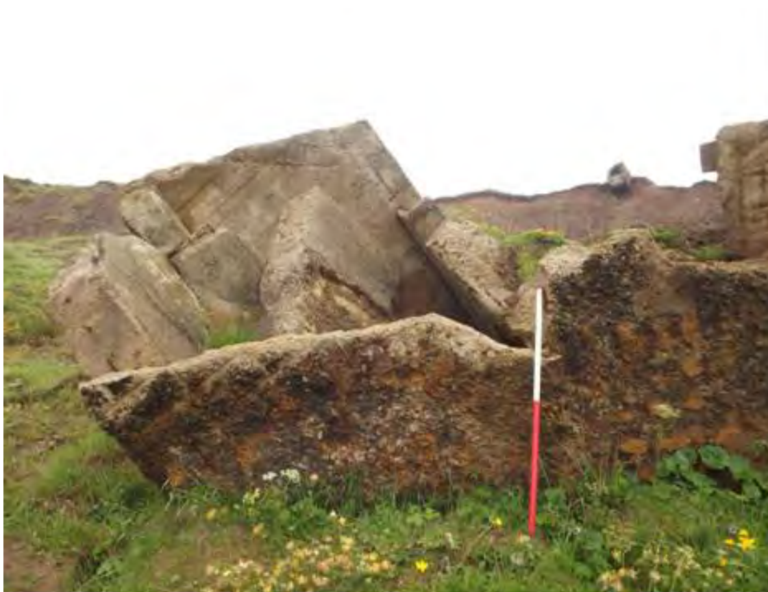
Plate 120 Second World War section post CY9, damage at eastern end, looking south (1m scale)
