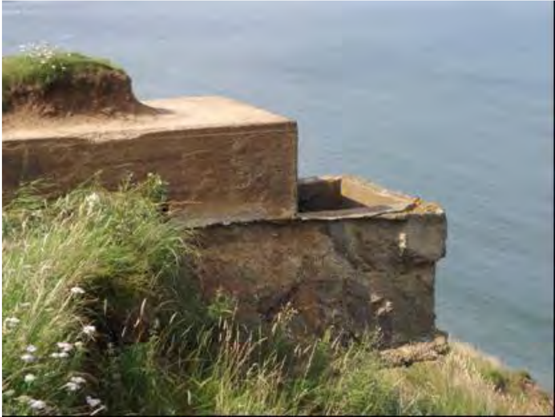
Plate 107 Second World War section post FD80, undermining of the seaward end
