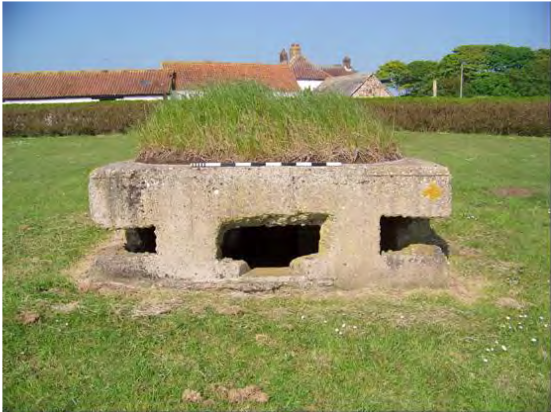
Plate 3 East wall of possible heavy weapons pillbox BA10, modified in Second World War, looking west towards Auburn Farm (1m scale)
