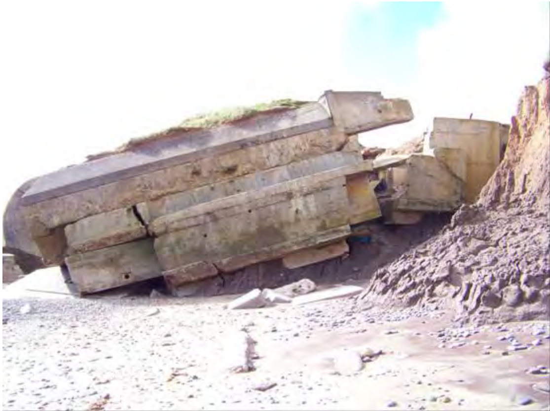
Plate 185 Godwin Battery, Easington (EA182), remains of northern magazine, looking south
