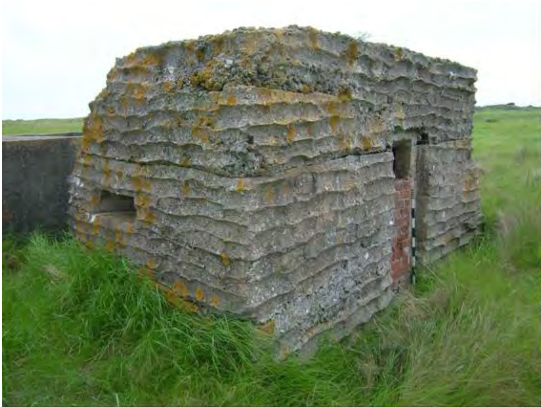
Plate 79 Pillbox SH1, Saltfleetby showing rear entrance, machine gun embrasure in the angled side and clear impressions of sandbag shuttering (1m scale)
