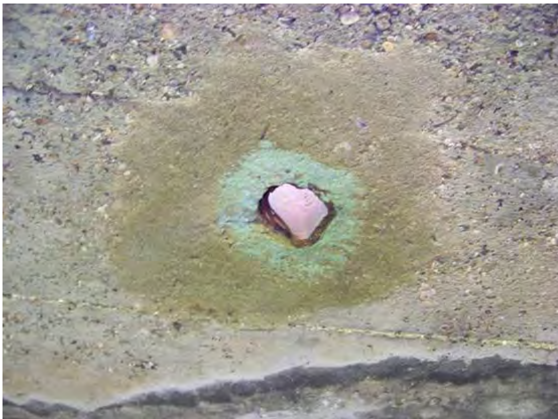
Plate 35 Ceramic pipe roof vent, BA30
