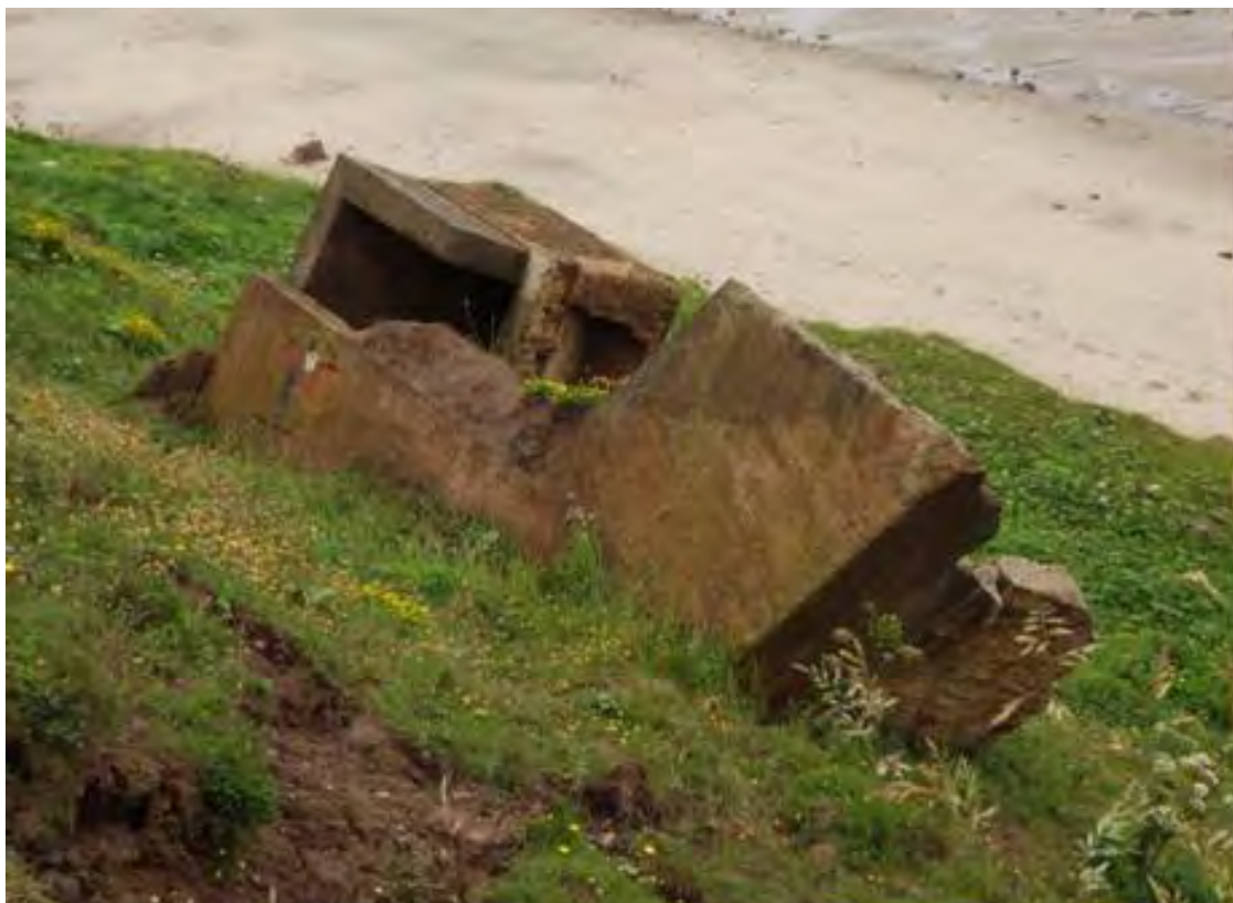
Plate 119 Second World War section post CY9, general view of roof, looking north-west
