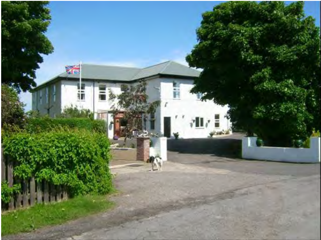
Plate 187 RAF Theddlethorpe, main block next to entrance, converted to residential home
