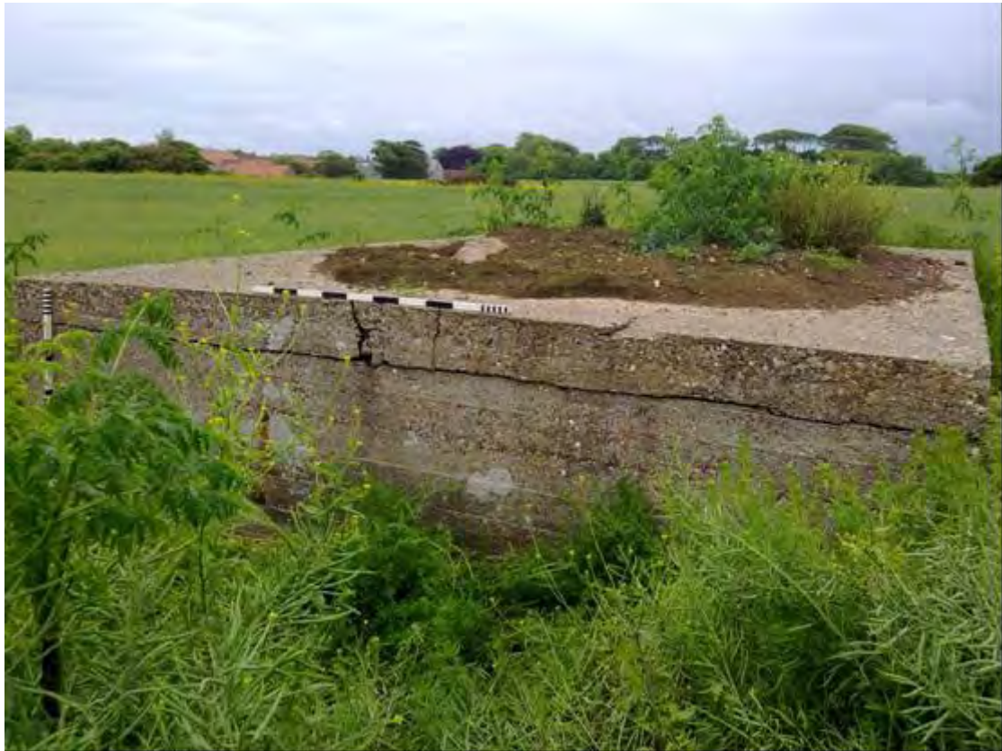
Plate 65 Semi-sunken command/communications post AT24, looking west (2 x 1m scales)
