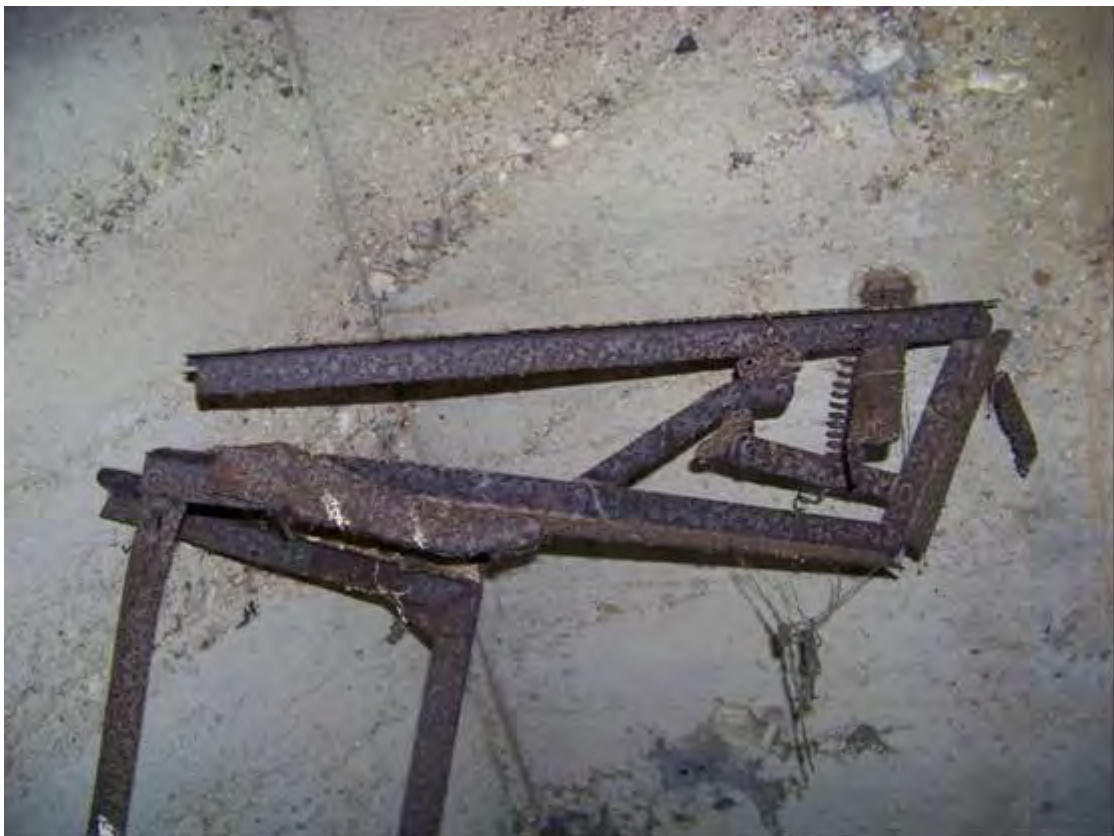
Plate 142 Second World War lozenge pillbox BA104, remains of upper section of Turnbull mount for machine-gun
