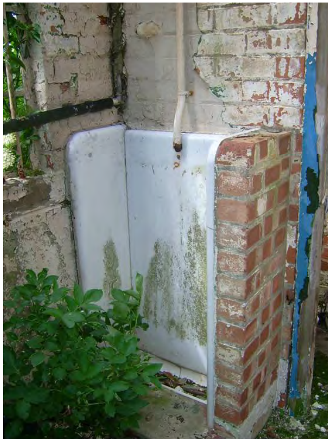
Plate 198 RAF Theddlethorpe, detail of possible post-war toilet
