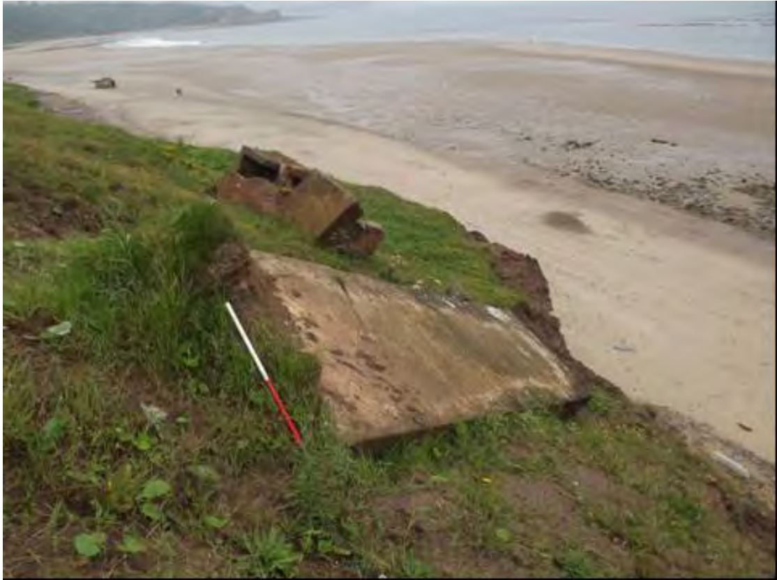
Plate 125 Second World War building close to section post CY9 (in background), looking north-west (1m scale)
