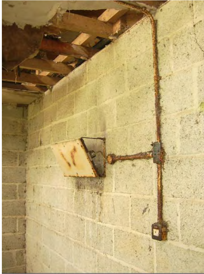
Plate 197 RAF Theddlethorpe, interior of end block, showing light fittings
