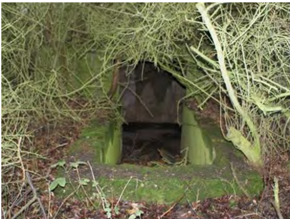
Plate 70 Entrance to command/communications post EG27, showing intact concrete retaining walls of passage
