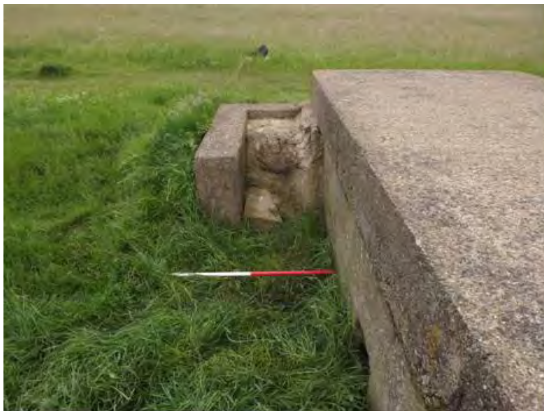
Plate 130 Second World War section post CY11, filled in access steps on the south-eastern corner, looking south (1m scale)
