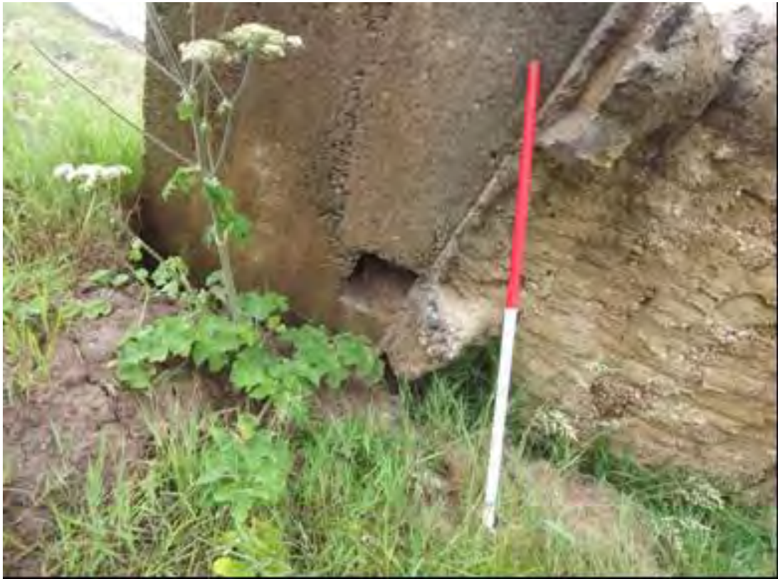
Plate 121 Second World War section post CY9, forward facing gun loop, showing rough cast concrete of the below ground portion and the overspill 'apron' of concrete at ground level, looking west (1m scale)
