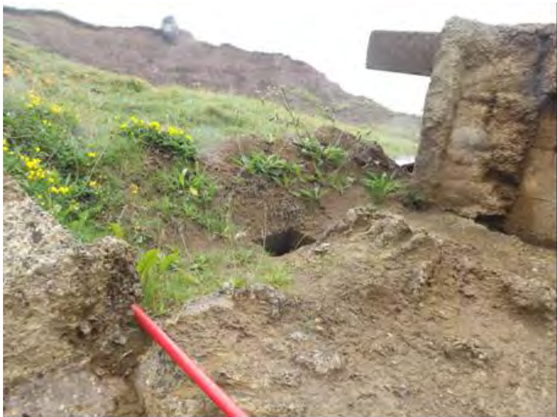
Plate 122 Second World War section post CY9, rear facing gun loop, looking southwest
