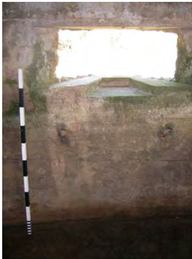
Plate 162 Second World War Lincolnshire-variant pillbox, detail of interior of embrasure, showing traces of metal firing shelf support brackets below (1m scale)
