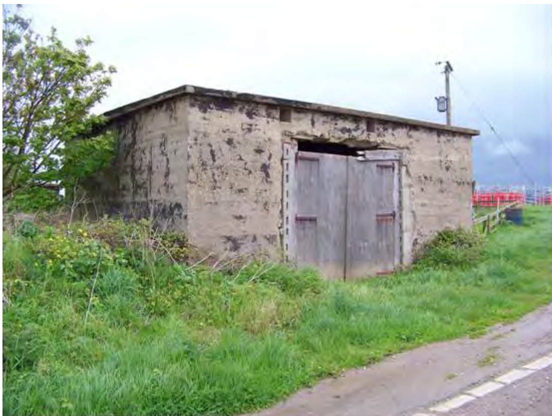
Plate 170 Second World War Ringbrough Battery, Aldbrough (AL55), battery plotting room, looking north-east
