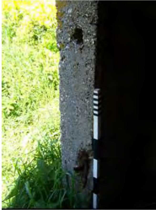
Plate 49 Pillbox BA190, detail of doorway, showing frame fittings (1m scale)
