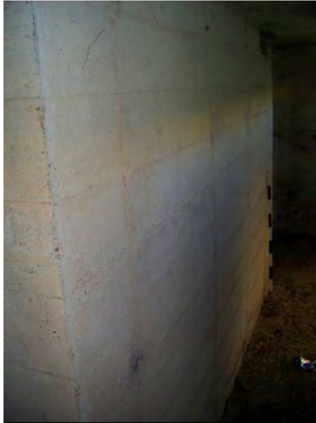
Plate 145 Second World War lozenge pillbox BA104, internal central anti-ricochet wall (1m scale)
