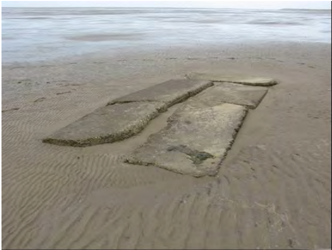
Plate 213 RAF Theddlethorpe, concrete hardstanding, part of beach bombing range in 2009
