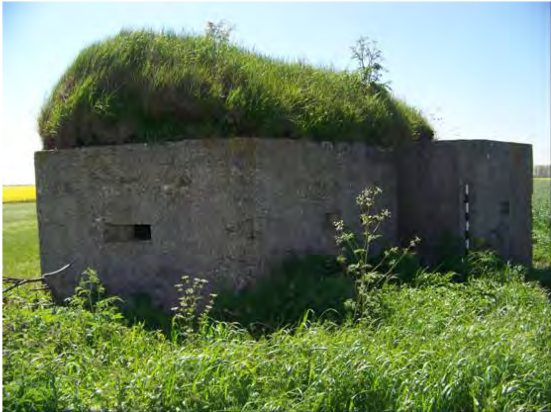
Plate 135 Second World War lozenge pillbox BA104, showing east and north walls and blast wall with embrasure (1m scale)
