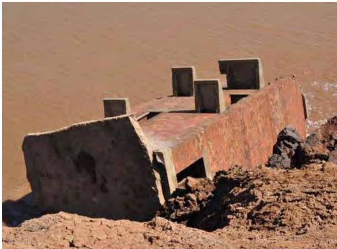
Plate 172 Second World War Ringbrough Battery, Aldbrough (AL55), collapsed Battery Observation Post, looking east from cliff
