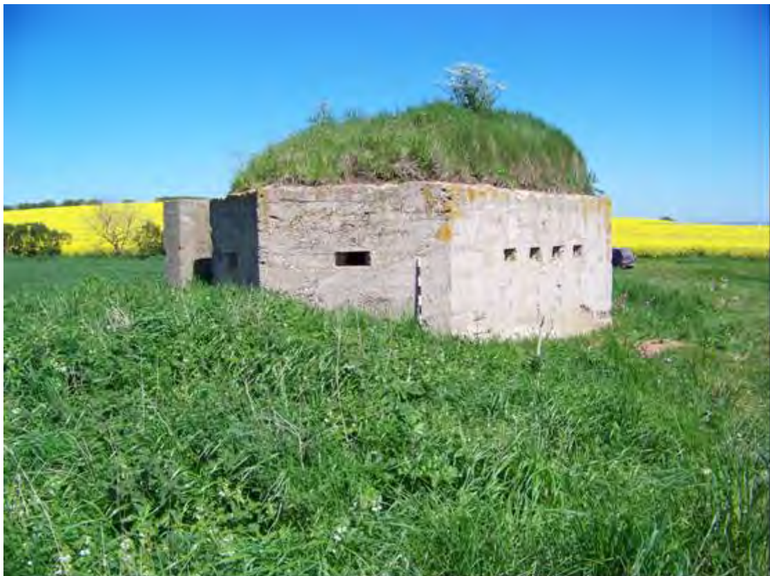
Plate 136 Second World War lozenge pillbox BA104, showing light machine-gun embrasures in end walls, looking north-west (1m scale)
