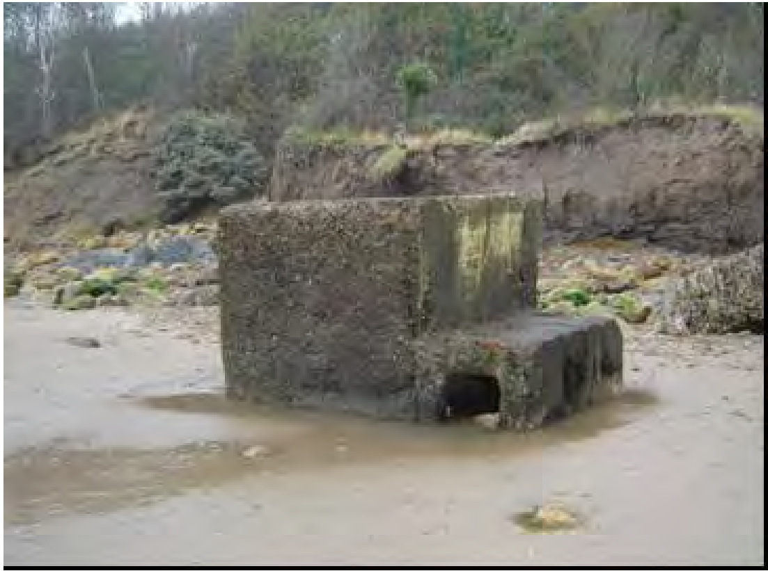
Plate 115 Second World War command/communications post OS10, general view, looking south-west
