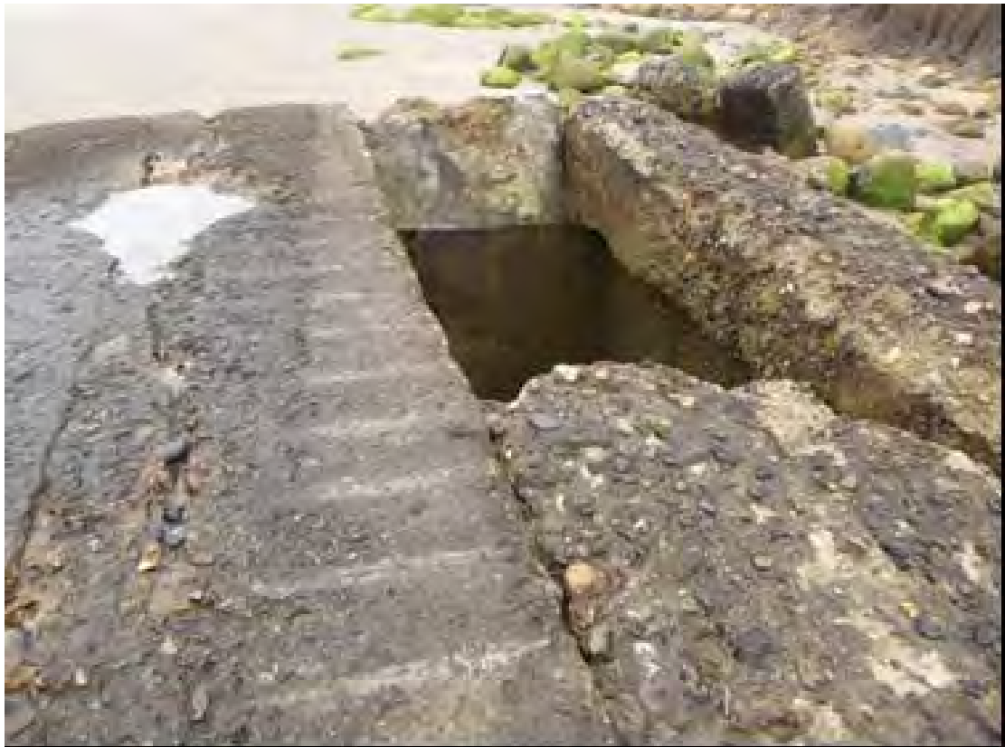
Plate 116 Second World War command/communications post OS10, opening on present upper face, looking south-west
