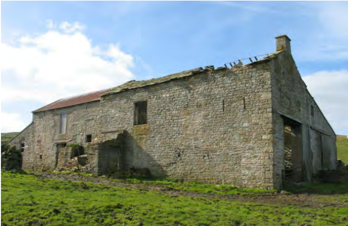
Figure 28. Holymire barn viewed from the south-east. The original bastle forms the south-western end of the building (to the left of the photograph) where the blocked first floor entrance can still be seen.
