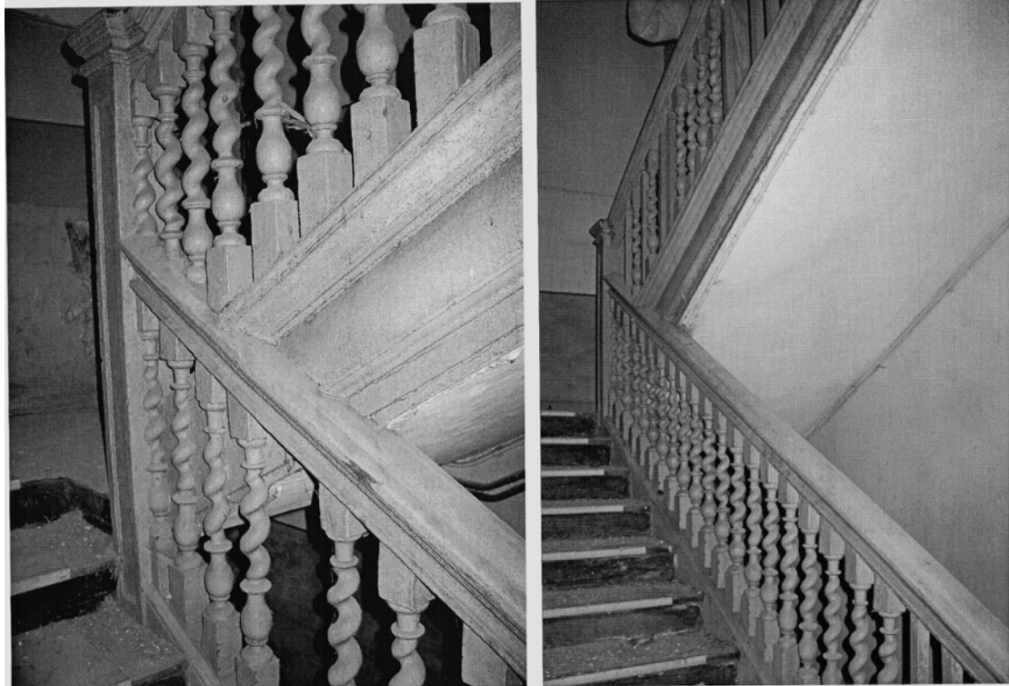
Fig. 28. Sherwin House, Pilchergate. The staircase. Pete Smith 2005.
