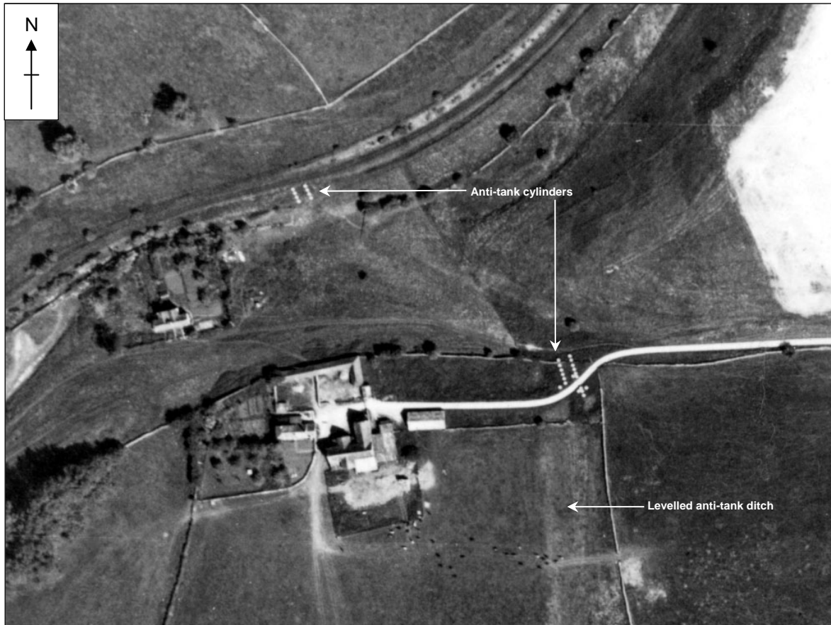
Figure 8.6: Two groups of anti tank cylinders at Little Larkhill Farm, Tetbury with the levelled anti-tank ditch just visible extending south to north. NMR RAF/CPE/UK/2110 3078 28-MAY-1947 English Heritage (NMR) RAF Photography
