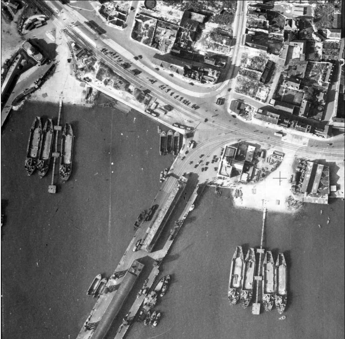
Figure 6.49: D-Day embarkation hards S2 and S3 Lansdowne Hill, Southampton. MKM614 and MKM615. The concrete loading ramps and associated dolphins were used in Operation Neptune, the assault phase of Operation Overlord. Photograph: NMR RAF/106G/UK/650 5291 12th August 1945. English Heritage (NMR) RAF Photography.
