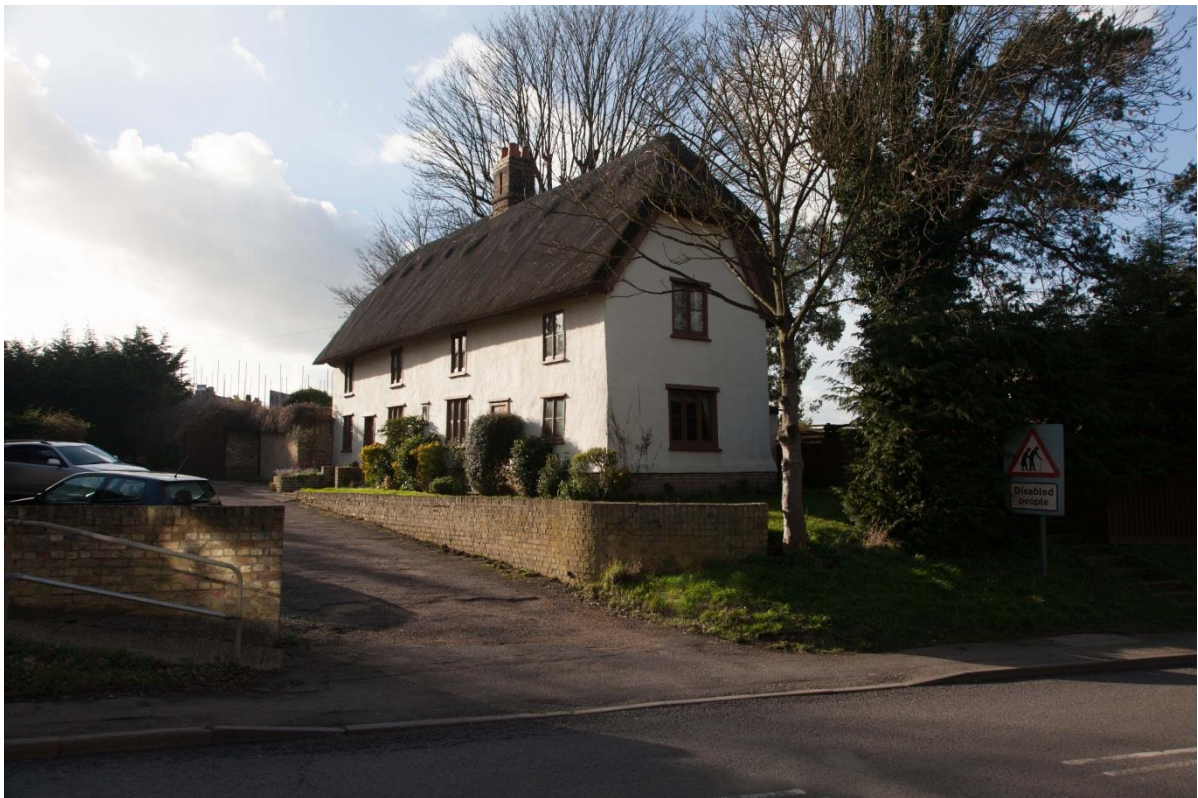
Figure 12.2: Development immediately adjacent to Grade II 18th century thatched cottage off Ermine Street
