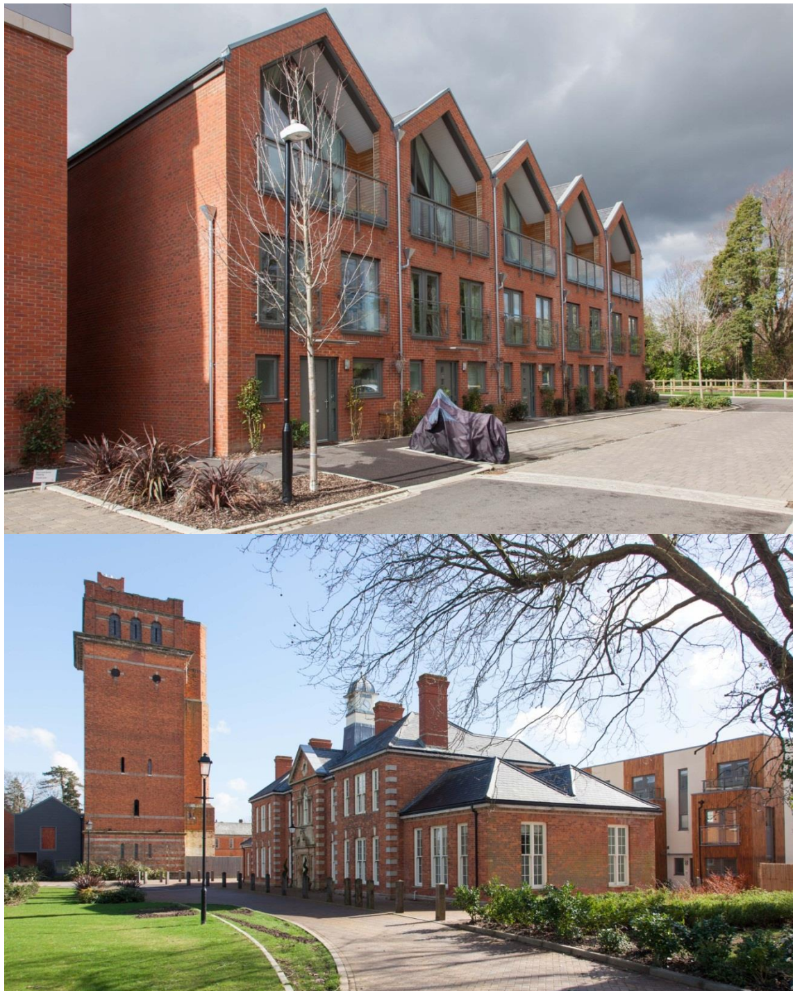
Figure 7.2: New build townhouse (top); extension to administration building (bottom)
