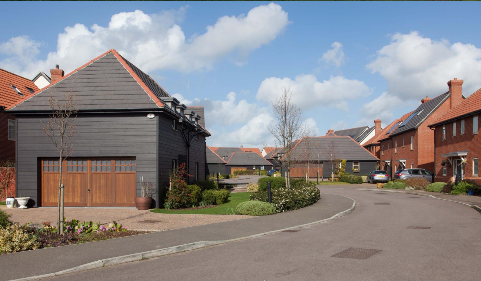
Bellrope Meadow. 'Work at home' units in black weatherboard.
