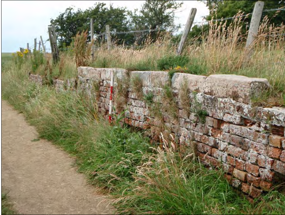
Figure 2.6 Handmade brick retaining wall with sandstone copings (scale = 1m).
