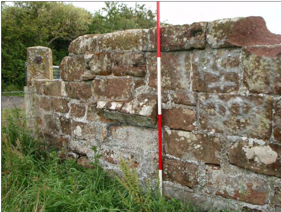
Figure 2.5 Springing line of an arch, possibly showing the location of a former water channel (scale = 2m).
