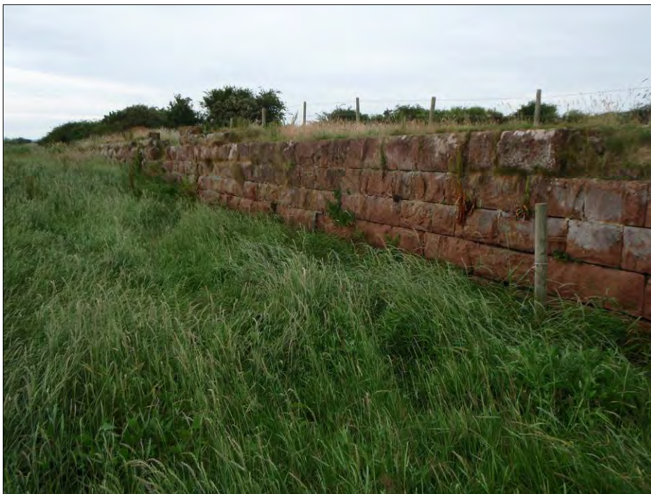
Figure 2.3 Neston Old Quay: Red Sandstone seawall surviving to c.1.8m in height.
