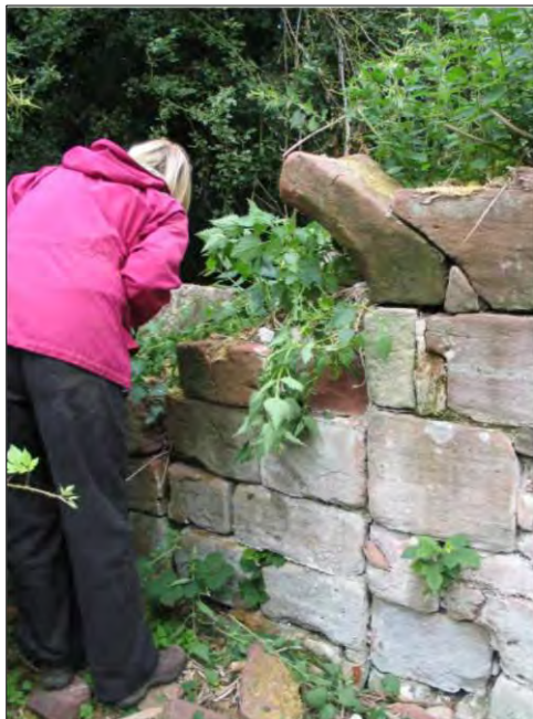
Figure 2.15 In-situ medieval doorway (Ainsworth 2010, © English Heritage)
