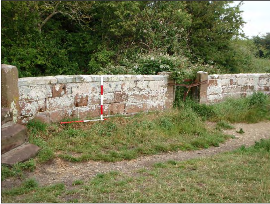
Figure 2.4 Remains of Red Sandstone walling, possibly associated with Neston Old Quay, remodelled and incorporated into garden walls. (scale = 1m x 2m).
