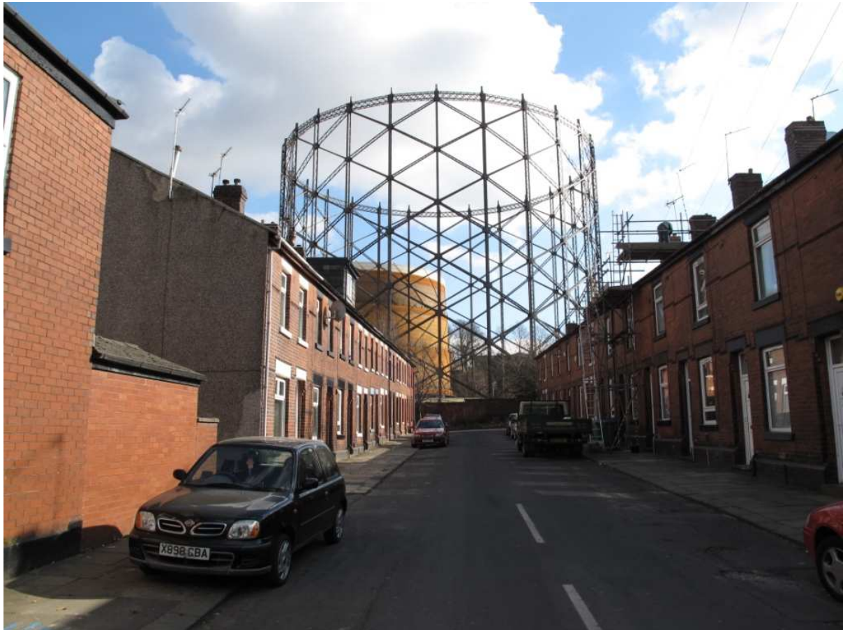
Figure 11h View along Briar Street, Rochdale, dominated by a gas holder
