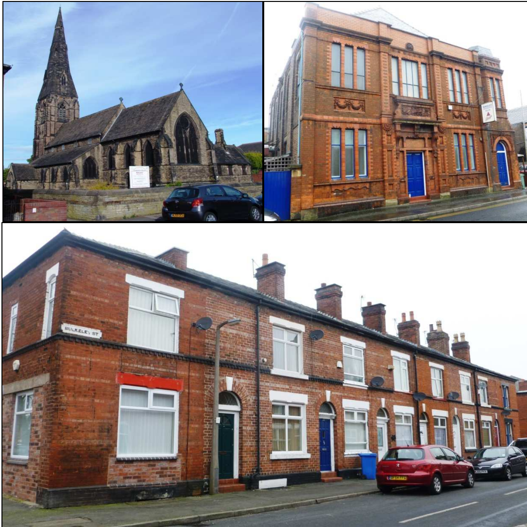
Figure 14f Predominant character of Edgeley with communal buildings and terraces associated with 19 th century industrial activity. Above (starting at top left): St Matthews Church, Edgeley Conservative Club and a row of houses on Bulkeley Street. The church and club are locally listed buildings
