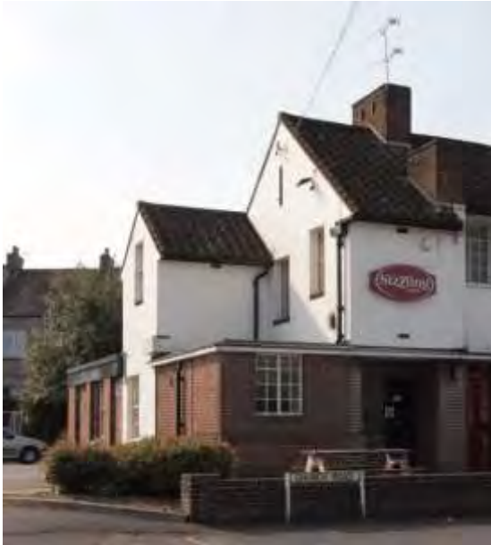
The remains of the corner 'Off Licence' at the Star, Soundwell Road, Soundwell, Architects: R. C. James and H. E. Meredith for The Bristol Brewery Georges and Co., Ltd. Fiona Fisher and Rebecca Preston, 2014
