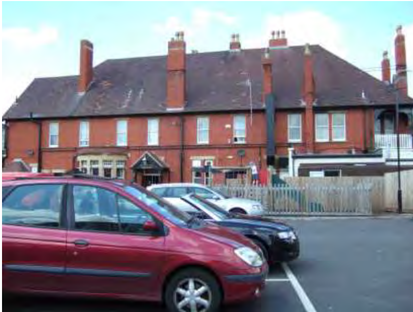
The rear of the Brunel (formerly the Engineers Arms), St John's Lane, Bedminster, Fiona Fisher and Rebecca Preston, June 2014
