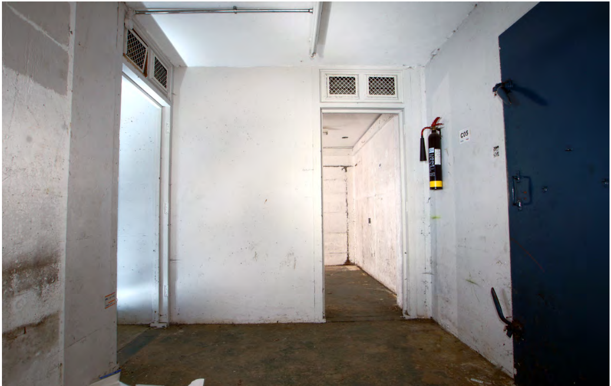
Plate 33: Exit air-lock with splinter-proof steel door and two door frames with exhaust vents above
