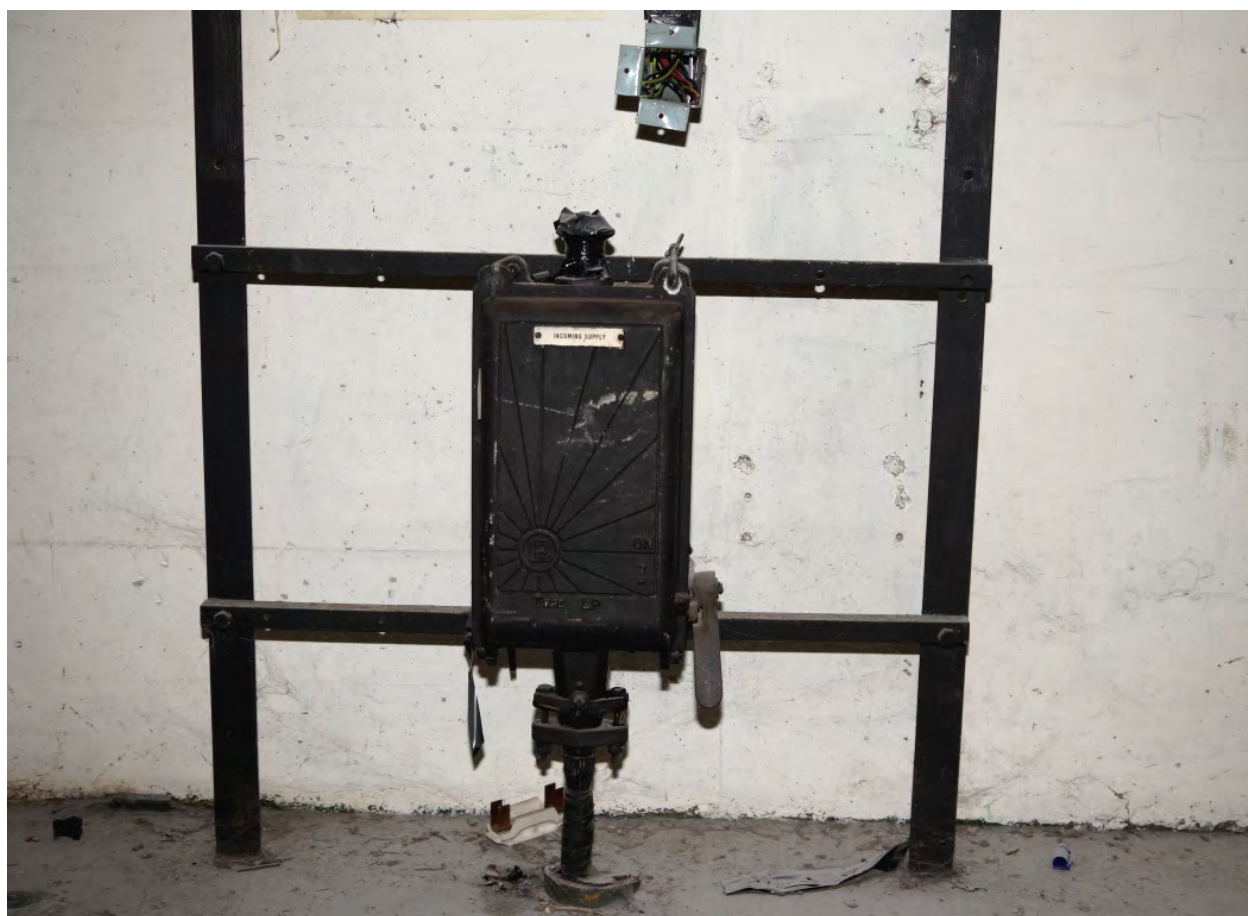
Plate 30: Auxiliary room 1 – incoming electrical mains
