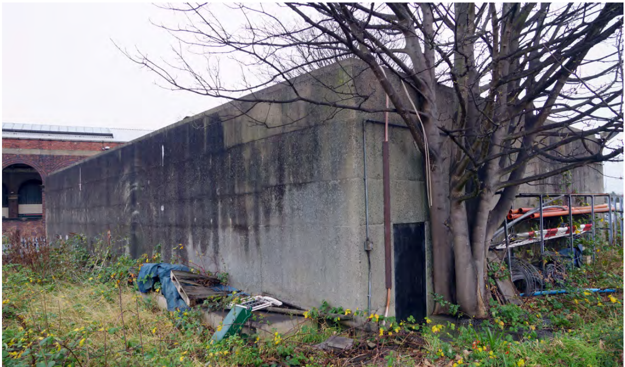
Plate 23: View looking north with exit in end wall It just possible to make out the curb on the roof which is set back from the wall perimeter. Marks made by the shuttering process of laying the concrete can clearly be seen.
