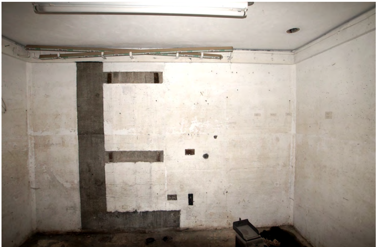
Plate 32: Auxiliary room 3 – phone and switch room Note the timber coving with steel brackets
