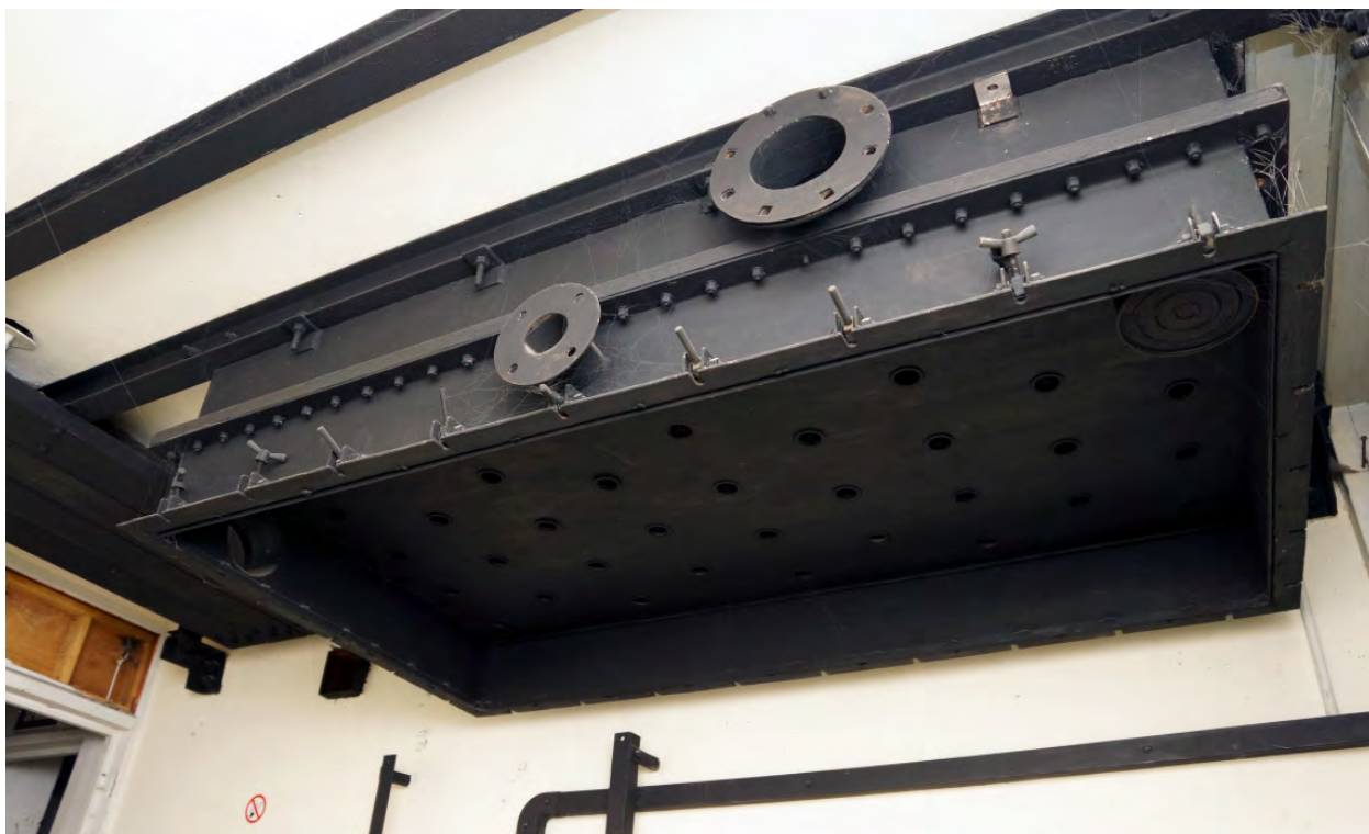
Plate 43: Post-war ceiling mounted ventilation filter
