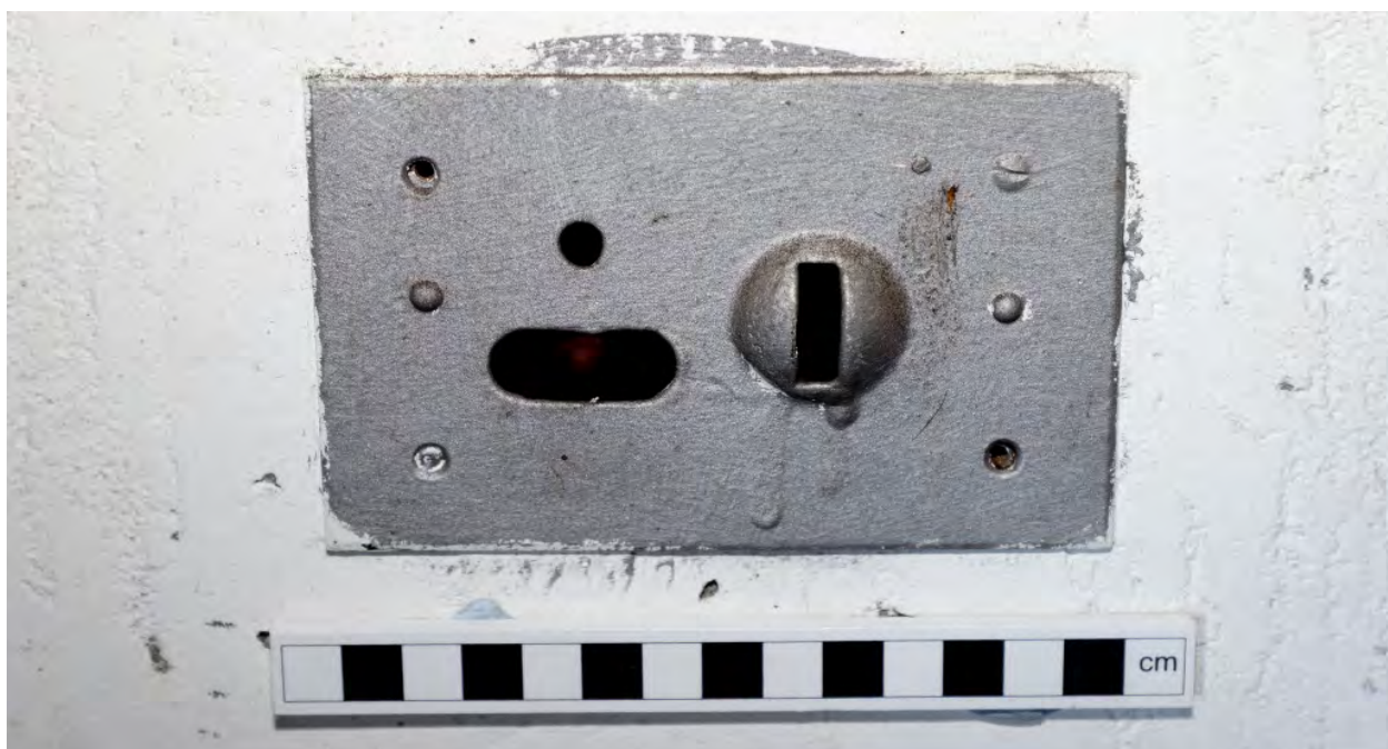
Plate 38: Wall mounted electrical switched socket plate of a type found in various rooms
