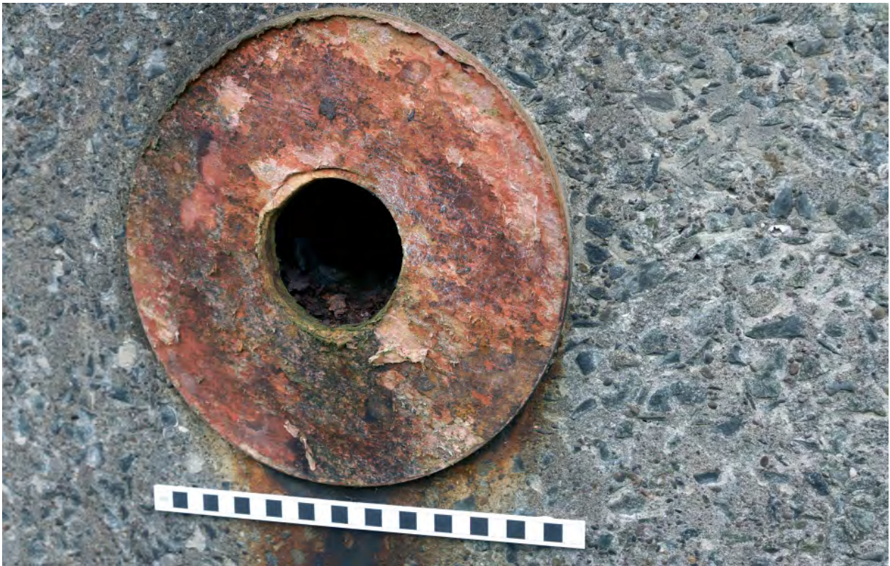
Plate 42: Exterior wall steel flange of what is believed to be a clean air vent - If this is the case then the vent would have risen vertically to take air from above a possible gas cloud. -
