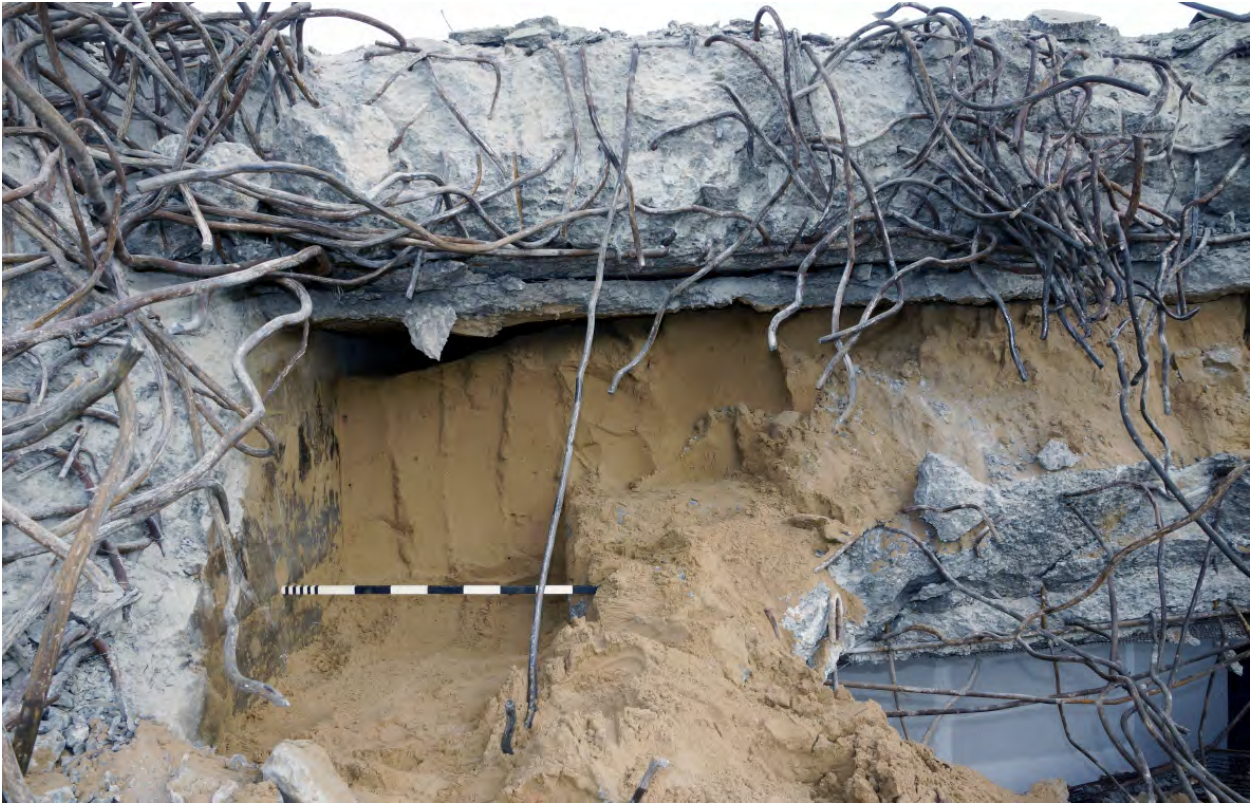
Plate 51: The wall and roof burster layer voids over the emergency exit air-lock
