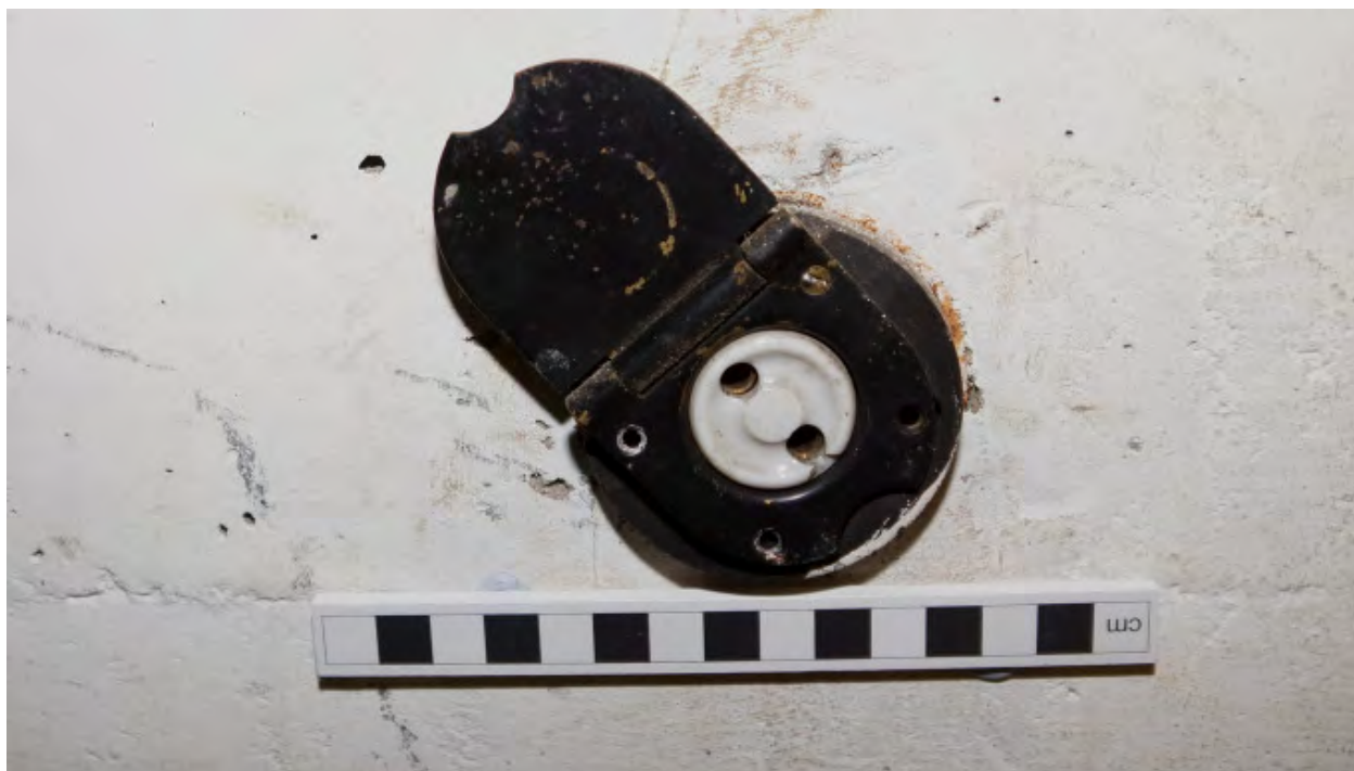
Plate 37: LMS communications wall socket inside rooms 2 and 3 -
