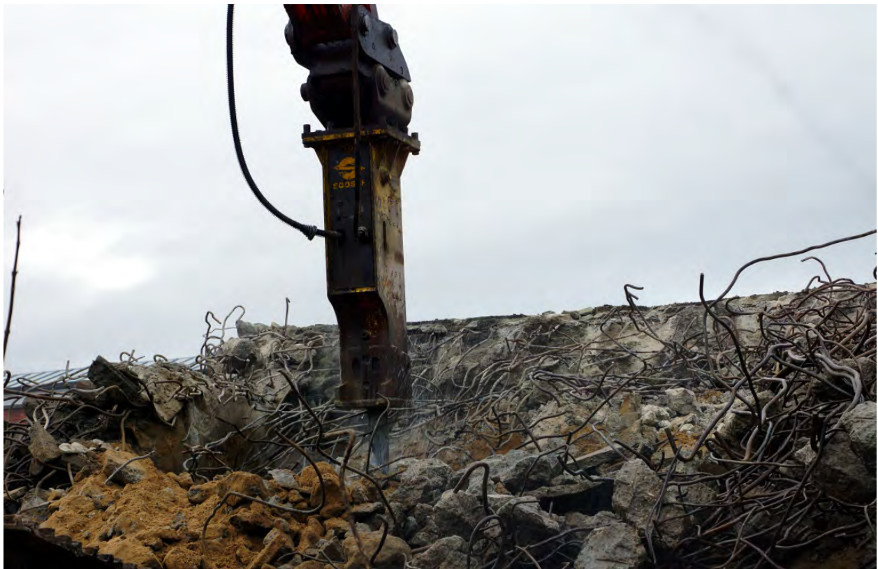
Plate 58: Hydraulic hammer in action
