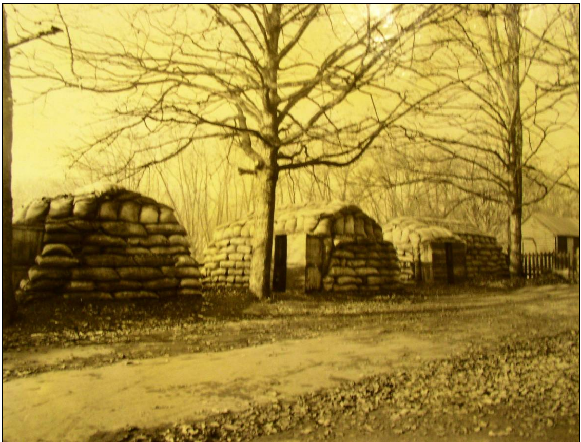
Figure 24: SRN: 514 - Royal Gunpowder Mills air raid shelters near Main Office. Image dated to 14 th November 1918 (RGPM Collection Ref: A.96)
