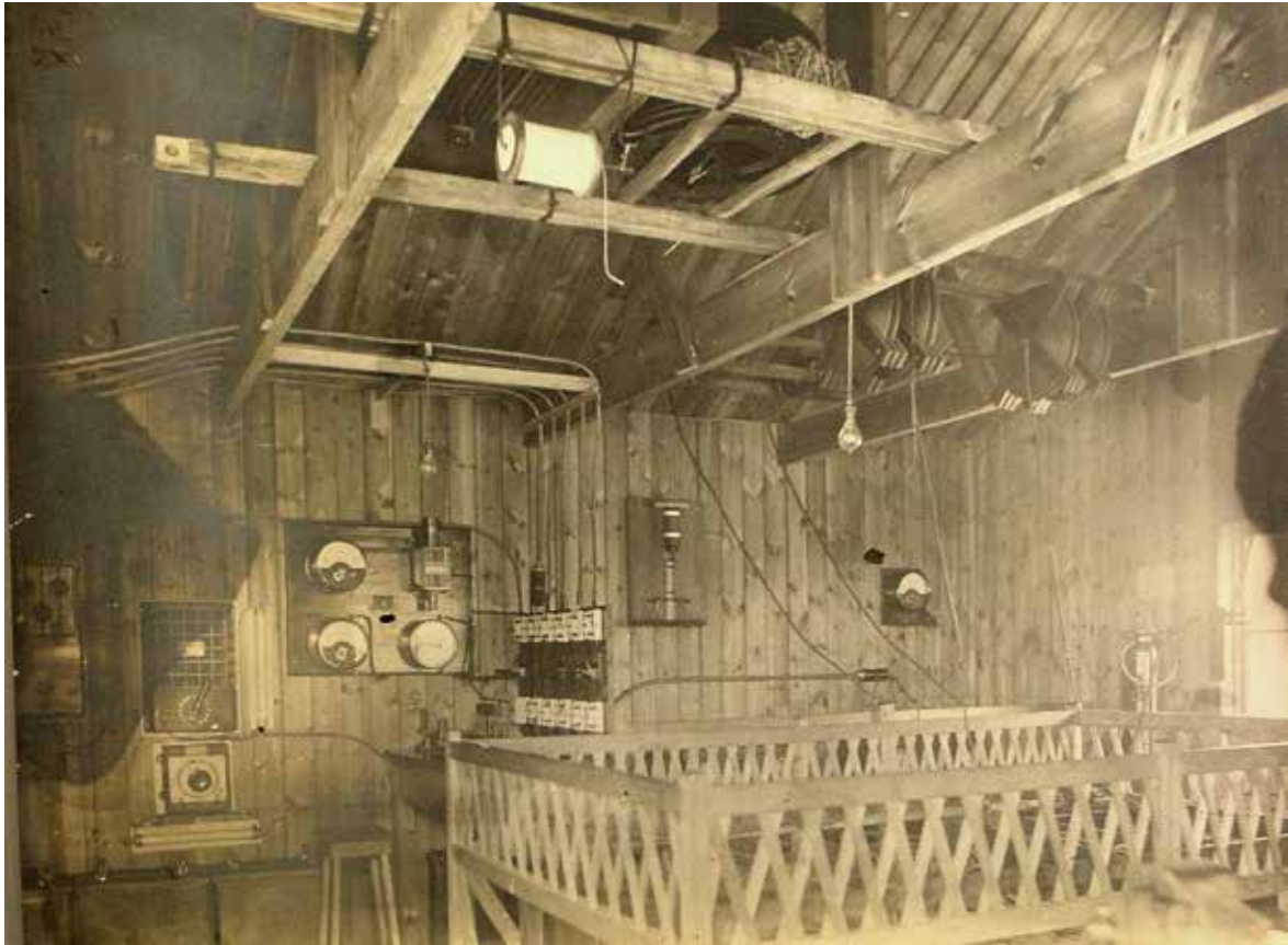
Plate 15: Interior of Marconi Station, Broomfield Road, Chelmsford (MS.Photogr.b.63 (2))
