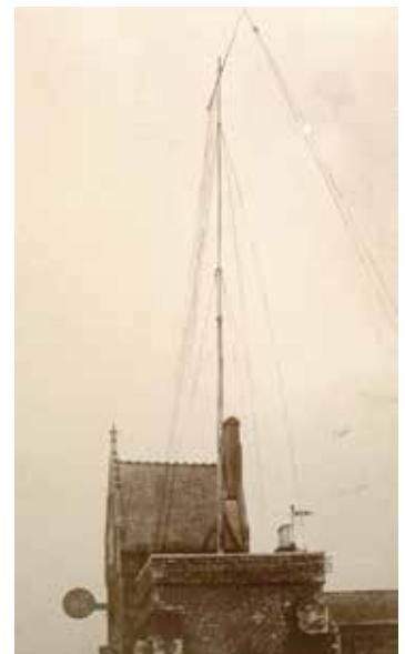
Plate 6: Wireless mast on unidentified building (MS.Marconi.181)
