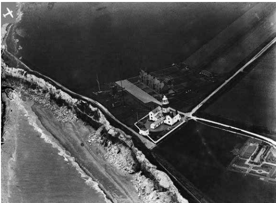
Plate 2: Hunstanton Wireless Station and Lighthouse, June 1920 ( http://www.britainfromabove.org.uk/image/EPW001849 ) © English Heritage
