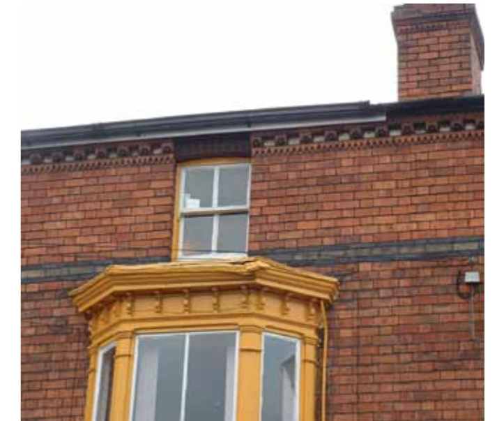
Figure 4 Decorative elements including moulded brickwork at eaves and polychromatic brick string course on terraced buildings along West Parade
