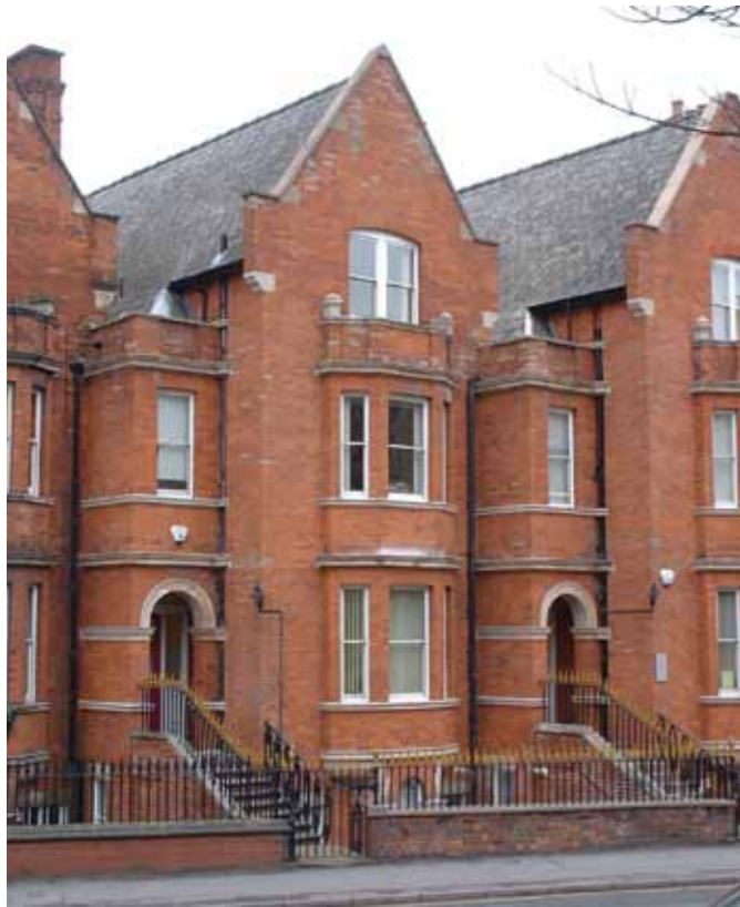
Figure 5 Terraced housing, stepped back around a corner on West Parade, with two storey brick bay windows and moulded decorative stonework
