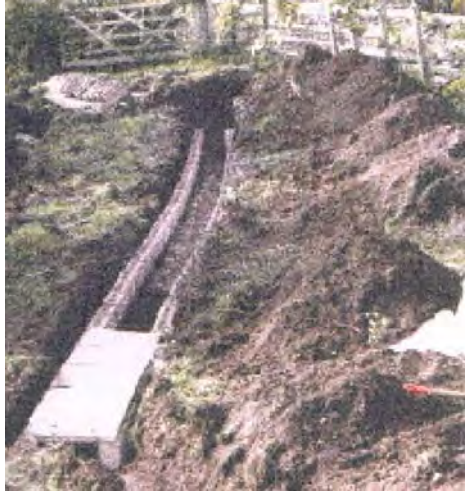
SECTION THROUGH TRENCH ARCH DRAIN
