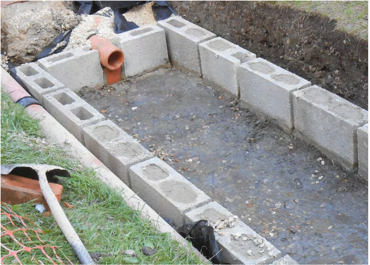
Figure 13: TAD Installation in progress, St. Mary's church, Childrey, Oxford diocese
