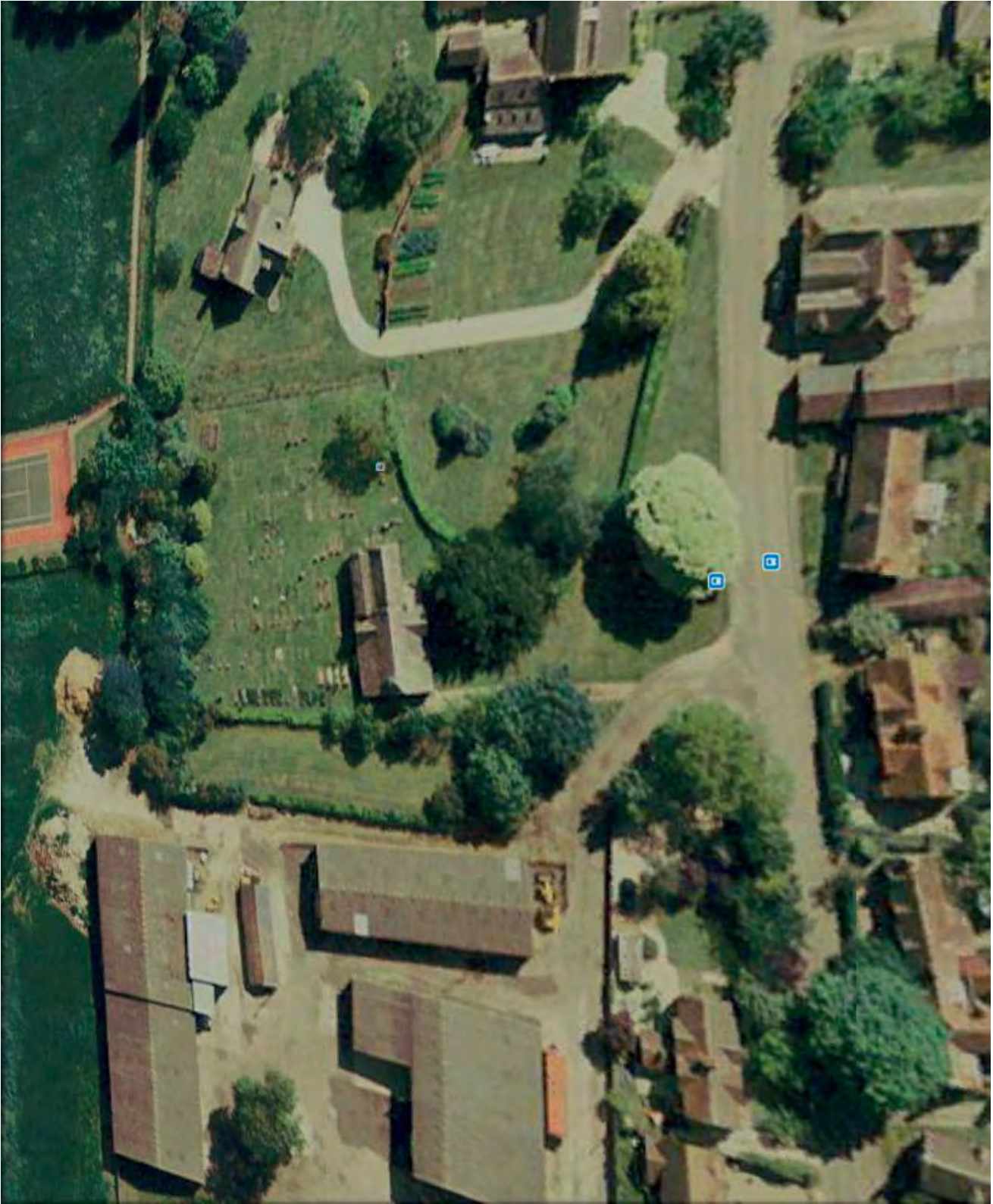
Figure A3.4: St. Katherine's church, Wormington, Gloucestershire (Google Earth, 2015, 52°01'33.72"N, 1°56'40.34"W, elevation 54m. < http://www.google.com/earth/index.html > [Viewed 25 February 2016].
