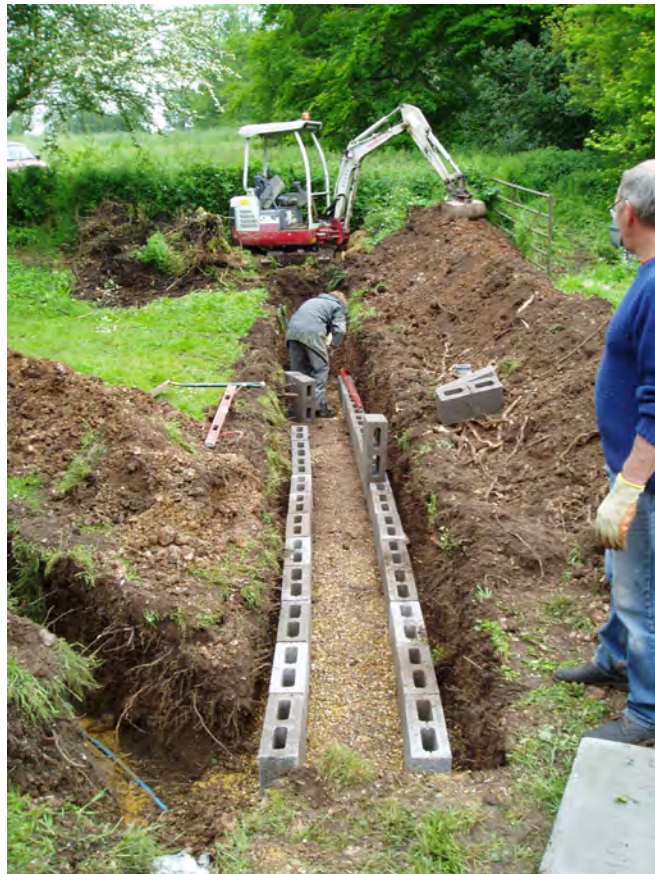
Figure 14: TAD installation working shot, Christ Church, Hatherden, Winchester diocese
