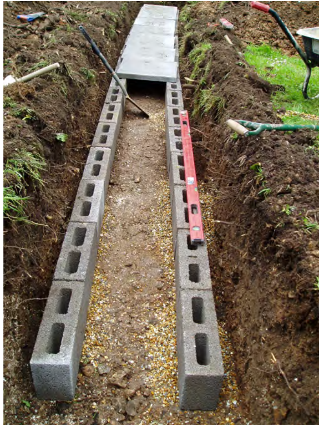
Figure 15: TAD installation in progress, Christ Church, Hatherden, Winchester diocese
