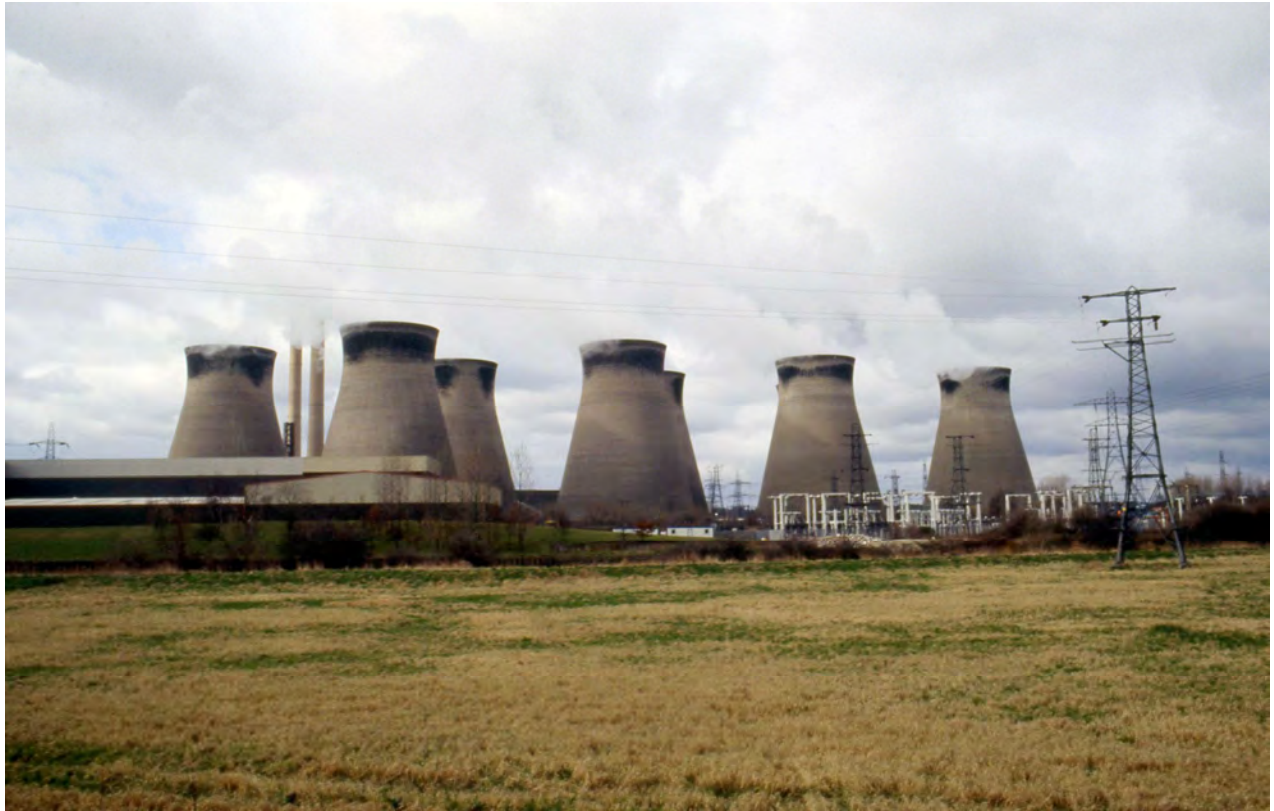
4. Ferrybridge Power Station in 1995 ©Wayne Cocroft
