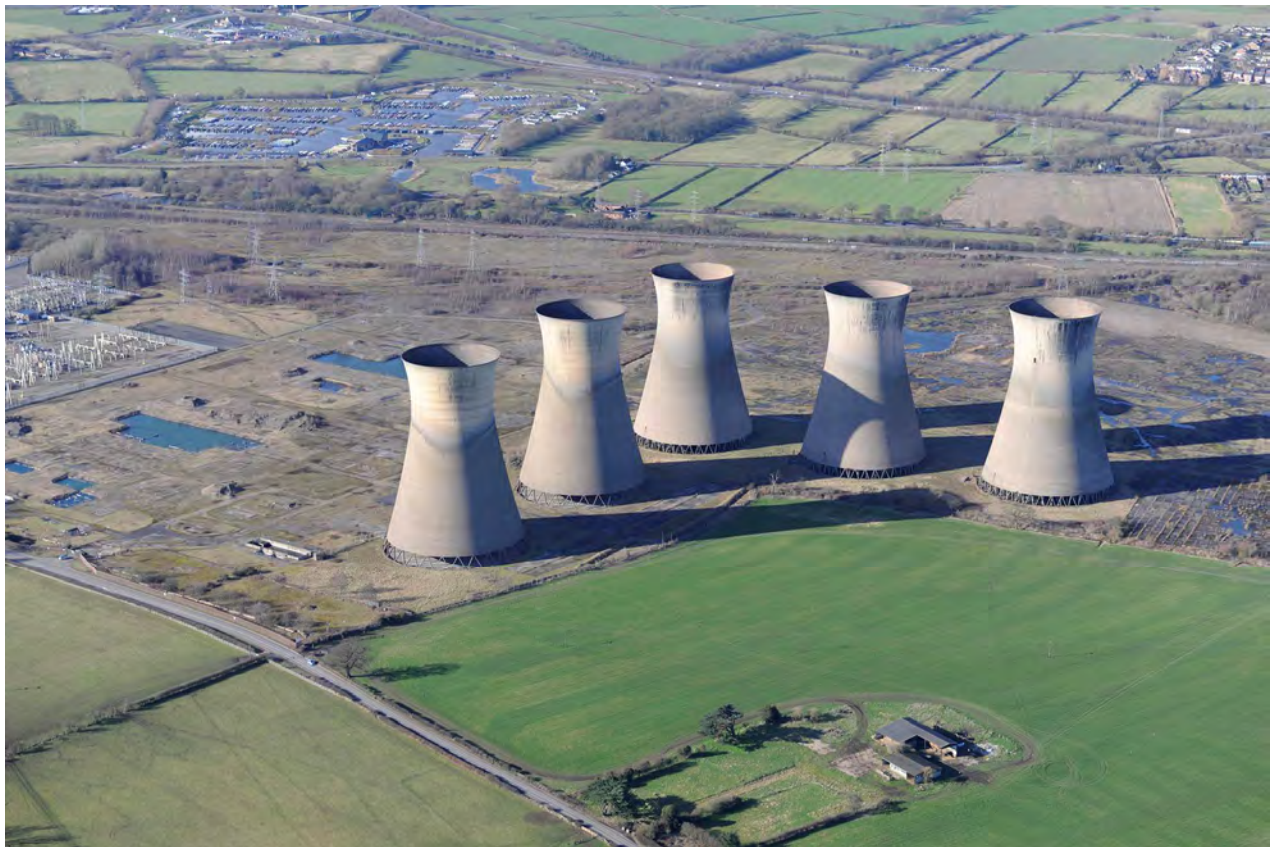
3. Willington power station, Derbyshire (1954-60; only the cooling towers remain) © Historic England 28666/03 -
