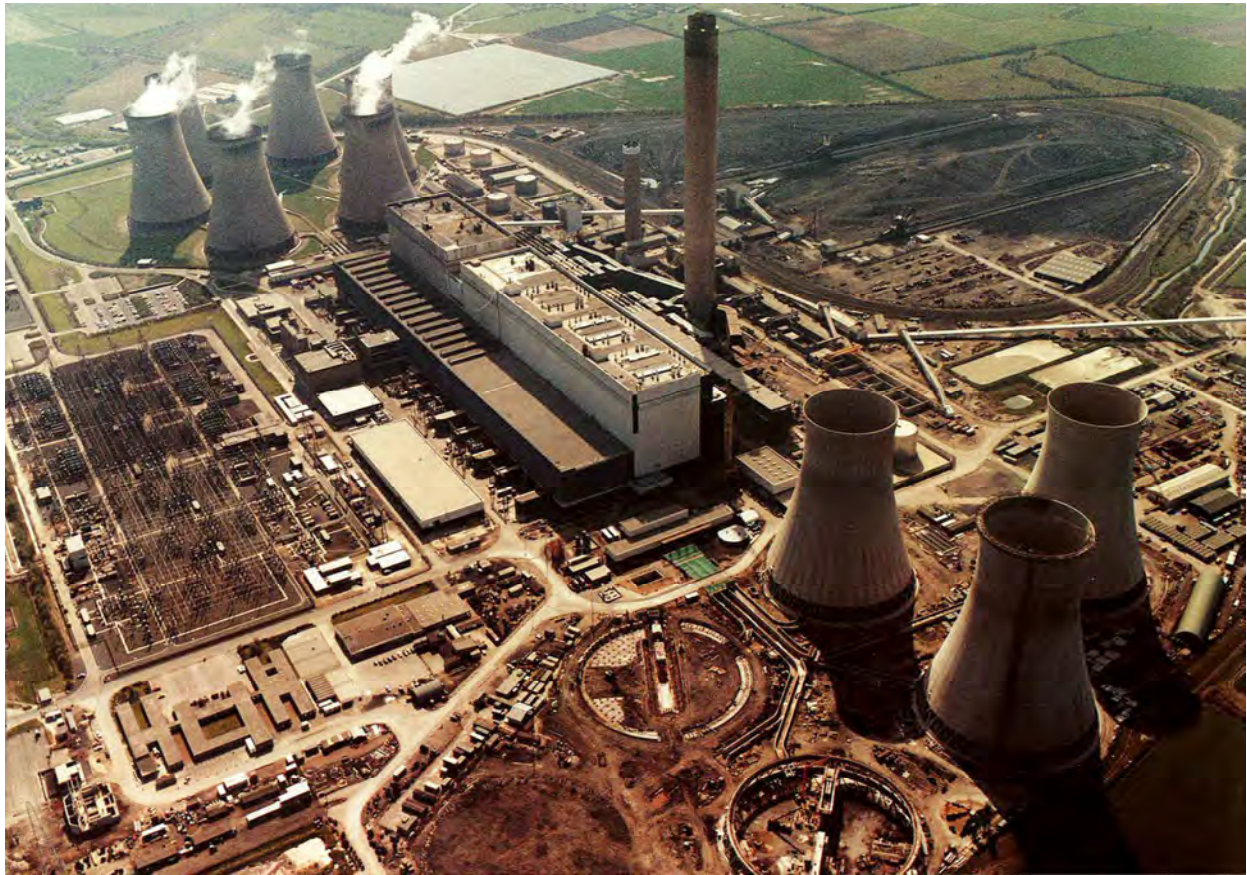
12. Drax, Phase 2, North Yorkshire (1978-86) nearing completion in c.1985. Then largest coal-fired station in Western Europe, its turbine house and boiler house is 433m (1421 ft) long and the entire site is 368 hectares (909 acres)
