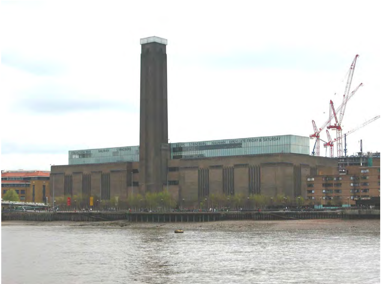
2. British Electricity Authority 1948-1955, Bankside, London, © Wayne Cocroft
