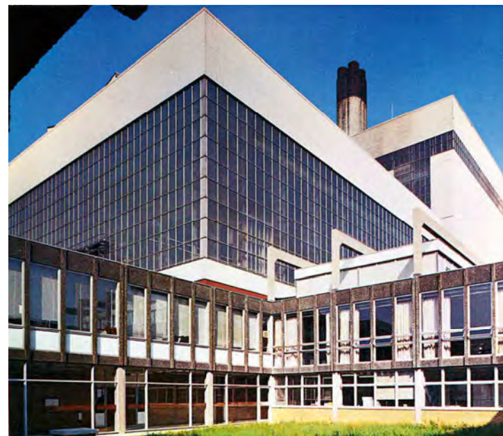
The turbine hall and boiler house tower over the administration block
