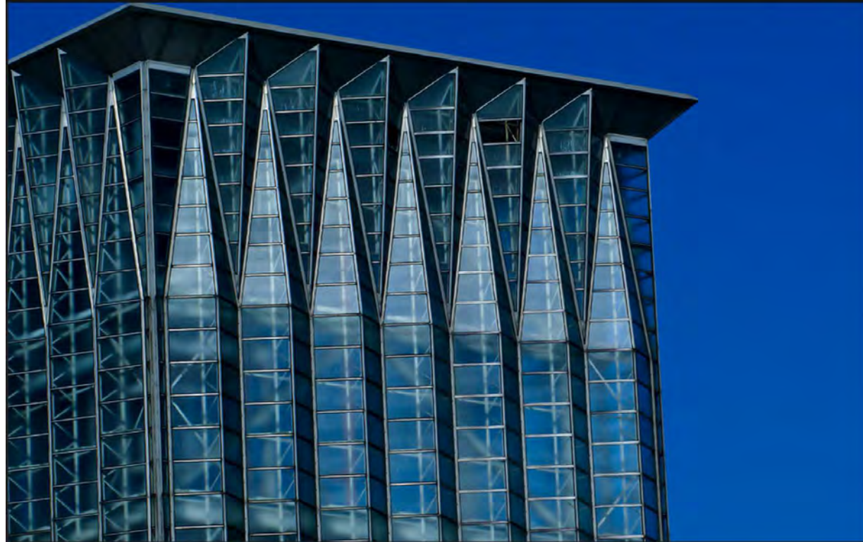
Above: Glazing at Fawley, Hampshire ©Historic England
