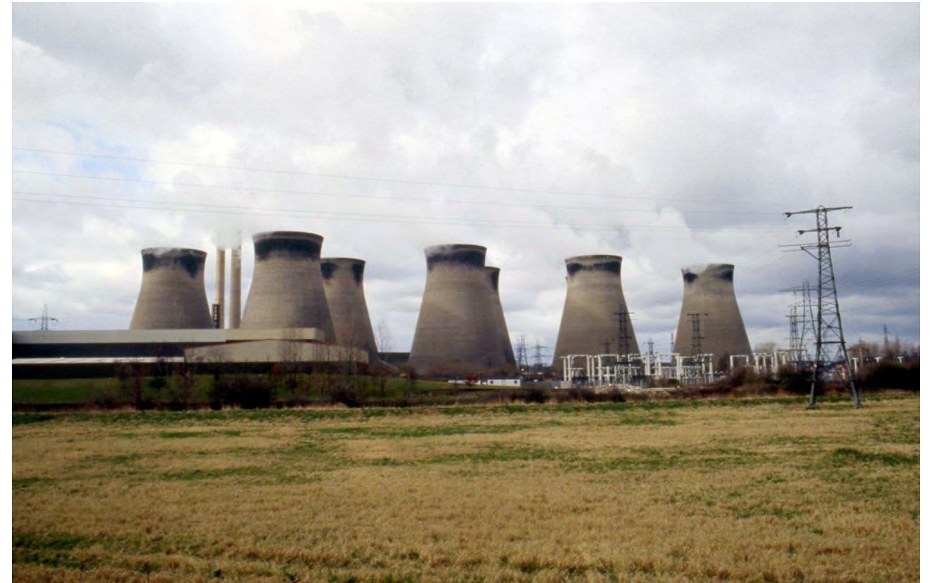
Above: Ferrybridge in 1995 © Wayne Cocroft.
