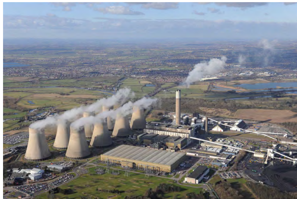
Below: © Historic England 28668_050
