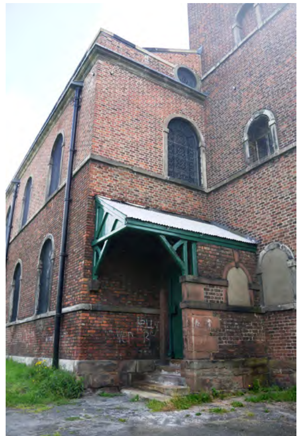
Locked entrance to the church on the north side
