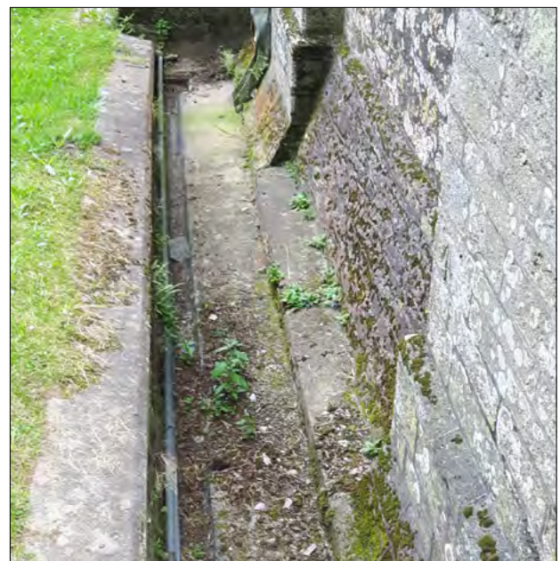
St Germans Priory's surface drainage / gully
