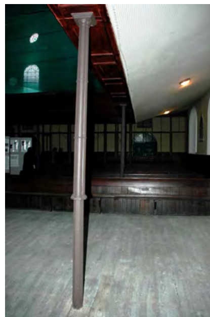
Cast-iron columns within the church © St James' Conservation Management Plan
