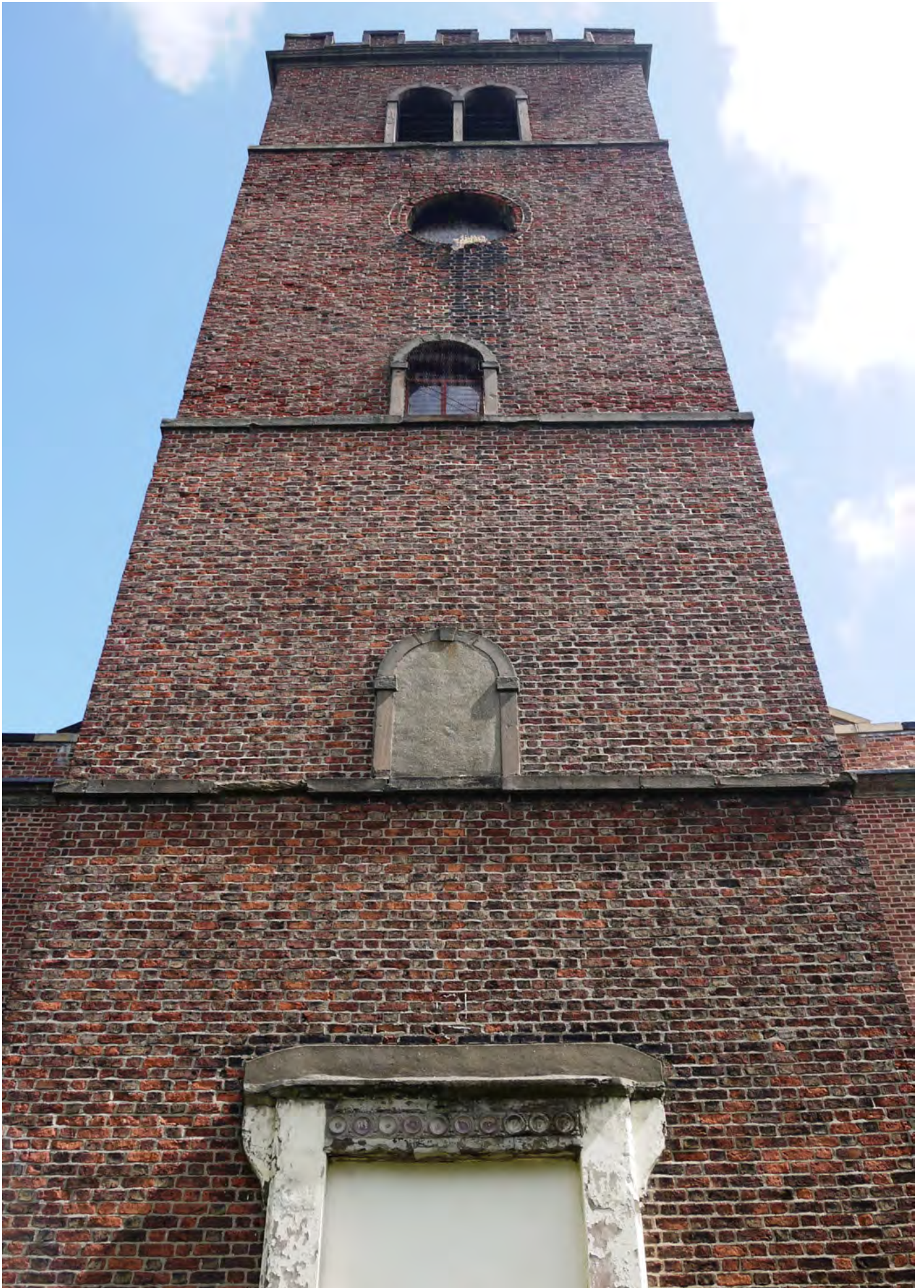
View of the west tower
