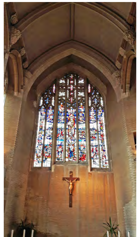
The liturgical east end, showing the differently coloured bricks used in the rebuilding following bomb damage during WWII
