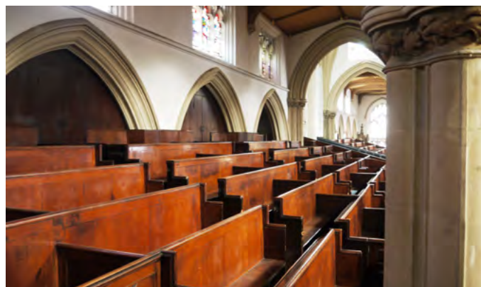
Box pews within the upper gallery
