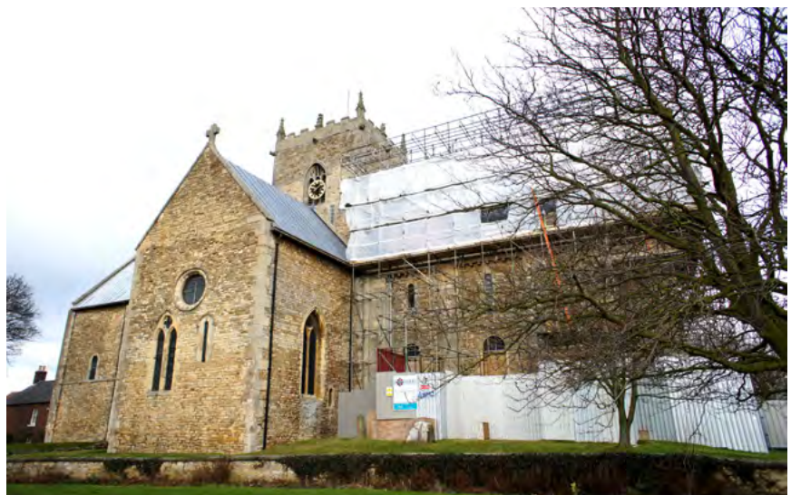
Repair works to the high-level roofs
