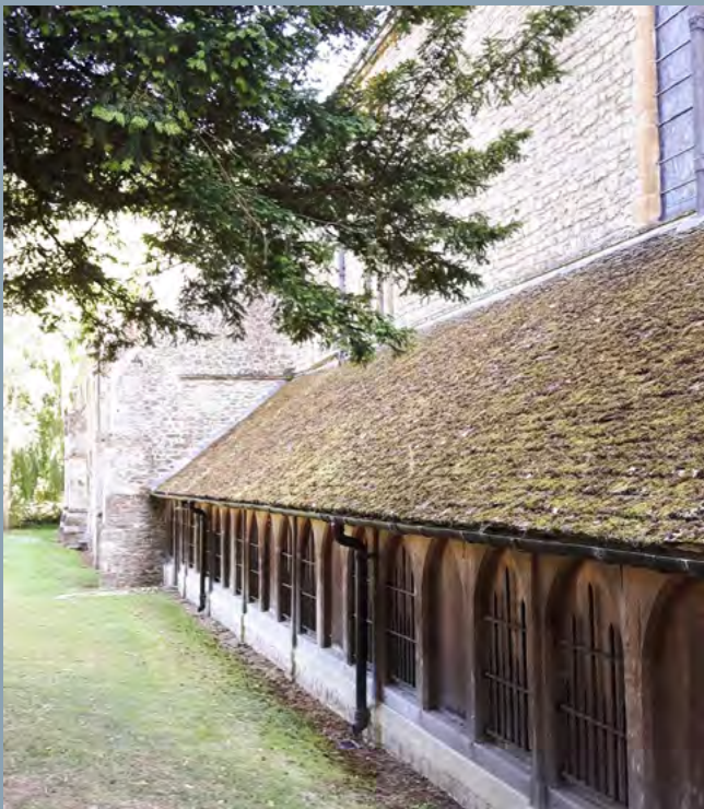
Exterior of the cloister gallery
