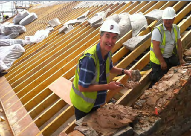
The current incumbent getting involved in the repair works
