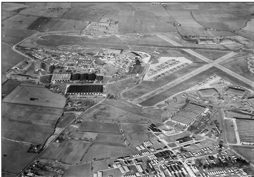
Figure 19. The military airfield of RAF Burtonwood (1390446), north-east of Warrington, showing the main runways, hangars and building complexes, along with the adjoining camps to the south.
