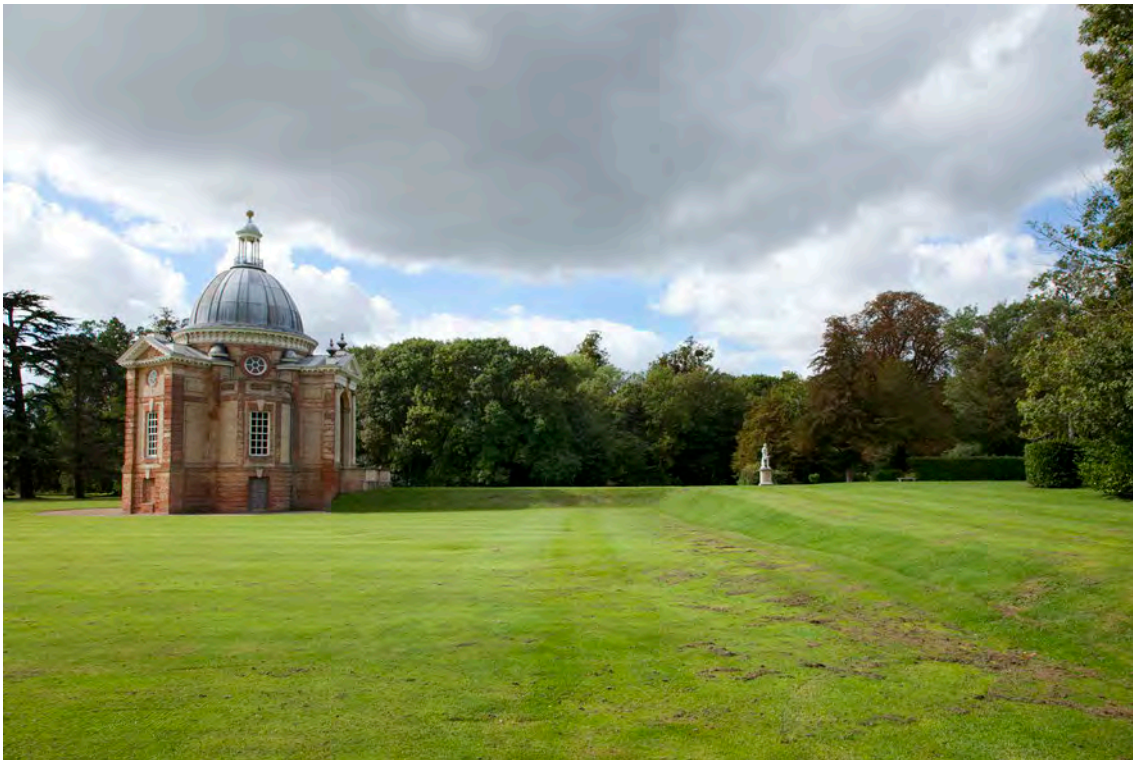
Figure 67 The pavilion, causeway and dam from the east (Patricia Payne © English Heritage DPI41075)
