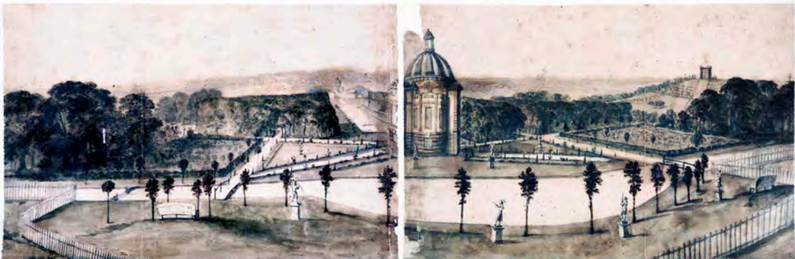
Figure 92 Angelis' view of the gardens from the south (BLARS L33/127 © English Heritage Archive, e850341/6)
