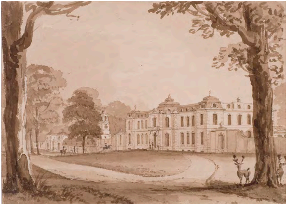
Figure 161 'North front of the new house, looking eastwards!' in pencil beneath (Steve Cole © English Heritage DPI 10100, by permission of a descendant of Thomas, Earl de Grey)
