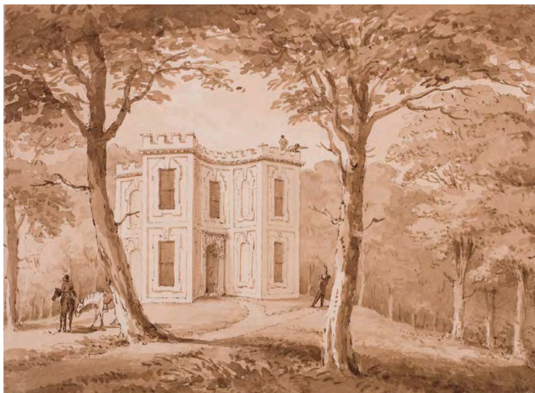
Figure 128 'The Hill-House', in pencil beneath; 'now pulled down' (Steve Cole © English Heritage DPI 10034, by permission of a descendant of Thomas, Earl de Grey)
