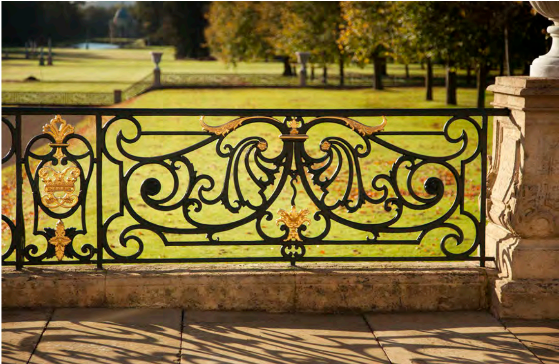
Figure 56 Dividing wall balustrade (Patricia Payne © English Heritage DPI 35910)
