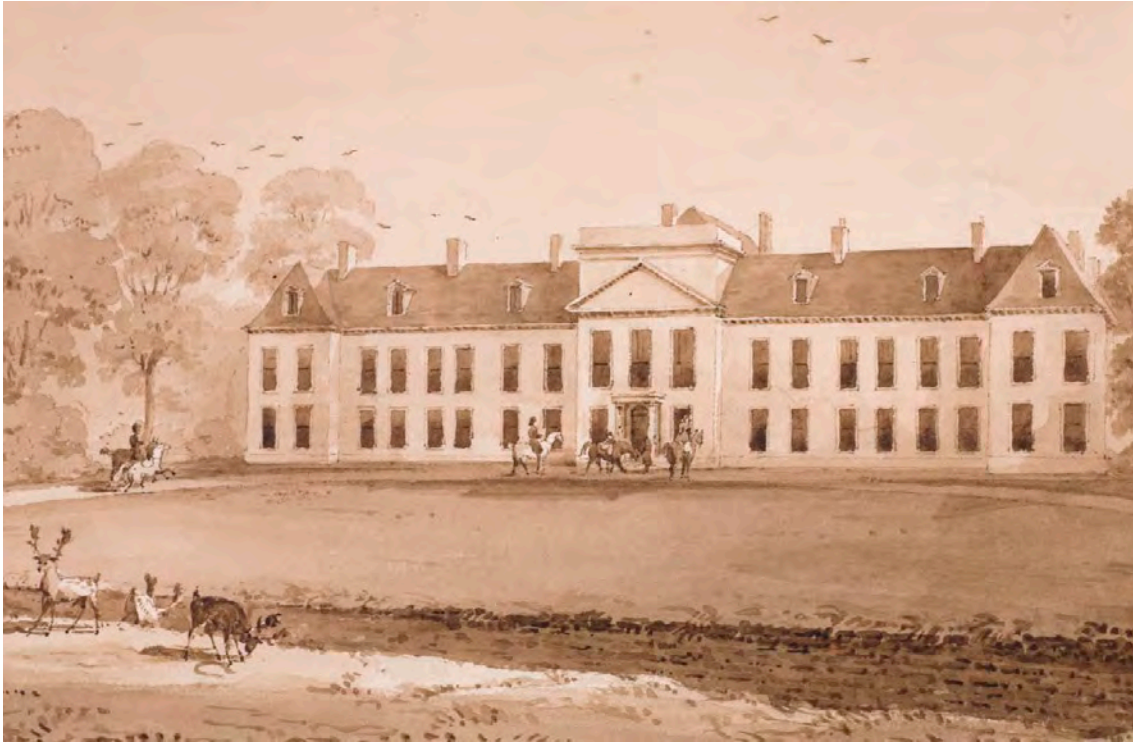
Figure 20 Sketch of the north front of the old house from the 1831 sketchbook (Steve Cole © English Heritage DPI 10020, by permission of a descendant of Thomas, Earl de Grey).
