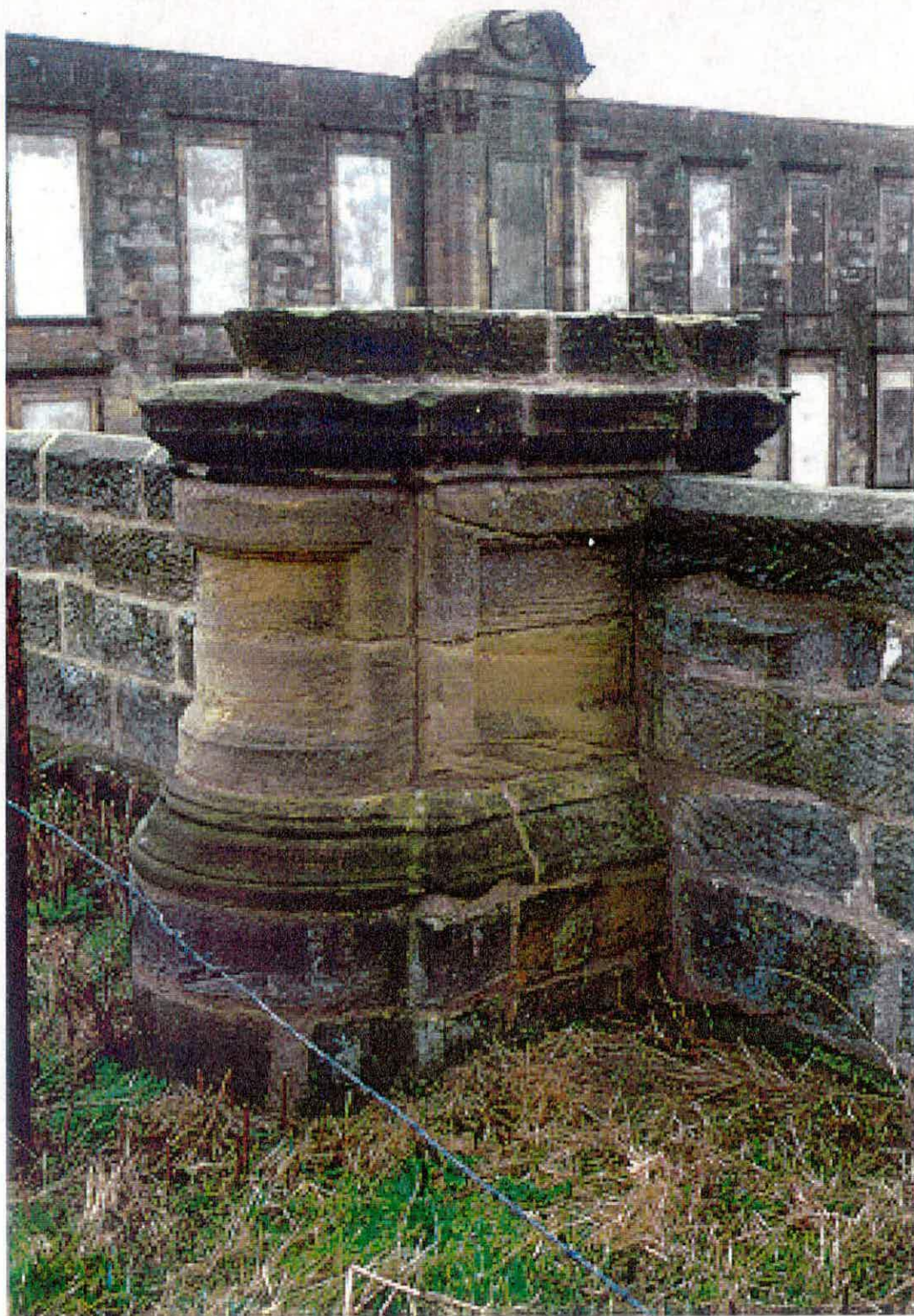
Fig. 16, a photograph of the pedestal in the east wall overlooking the court.
