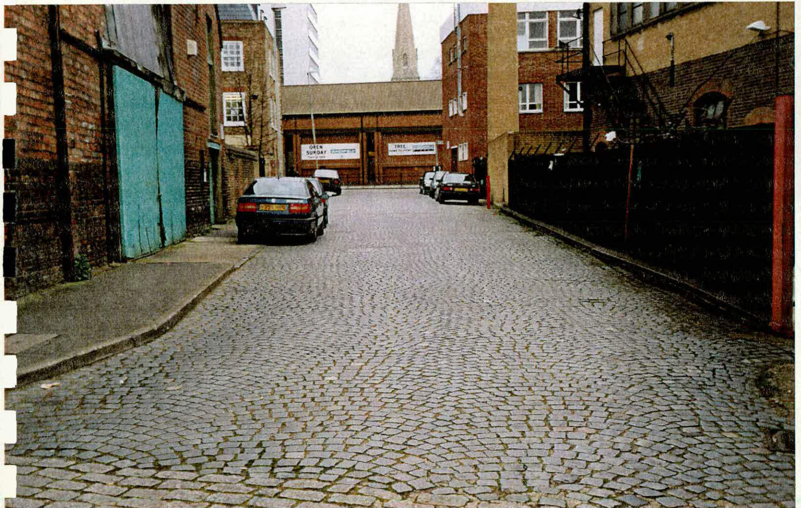
Underwood's hay and straw warehouse Dock Road, 1881, and below: Dock Road, cut through in 1859, with setts in a fan-shaped pattern.
