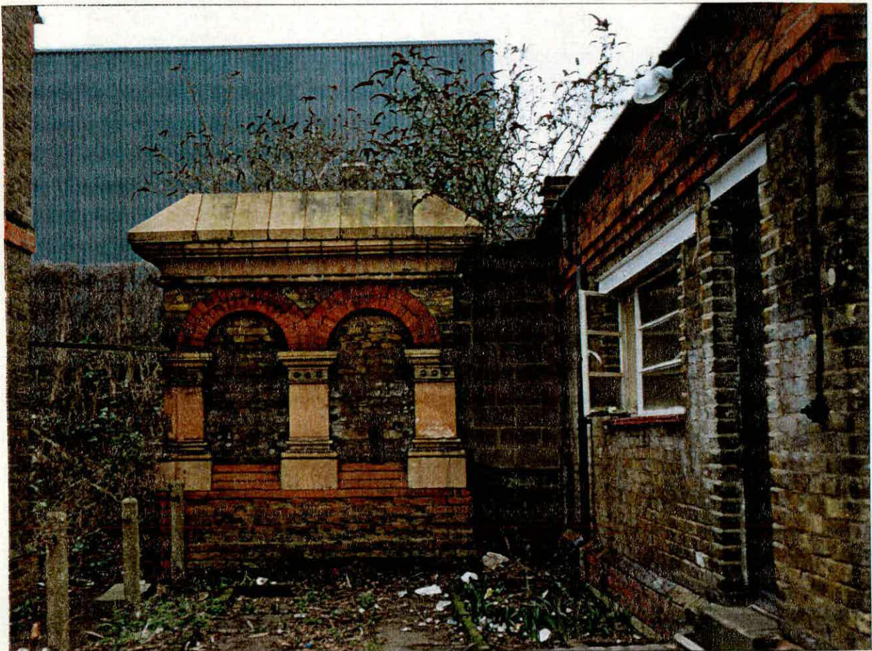
Pumping station: engineer's cottage and base of chimney, F.W. Lacey, 1883.
