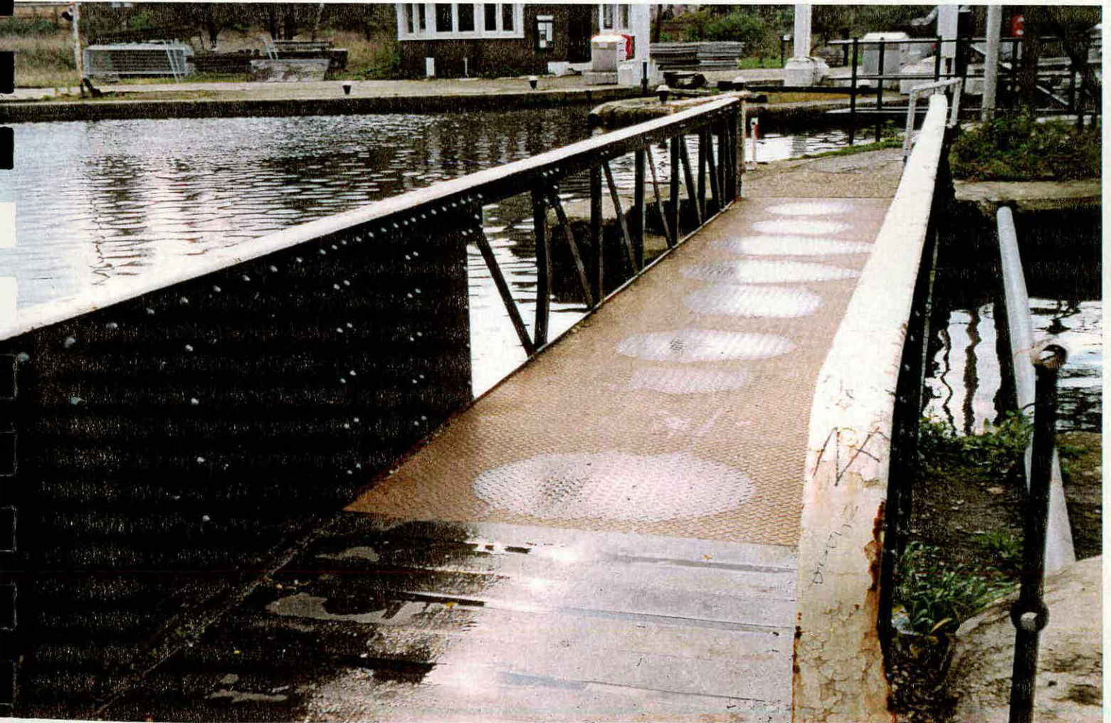
Brentford Lock Toll house, 1912 Swing bridge, c.1870
