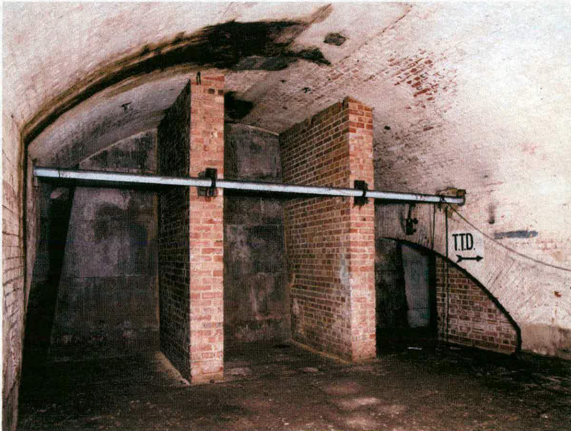
Figure 1 - the ashlar-faced pump platform wall of 1770, as seen from the north end of vault 3 (English Heritage, AA042381).
