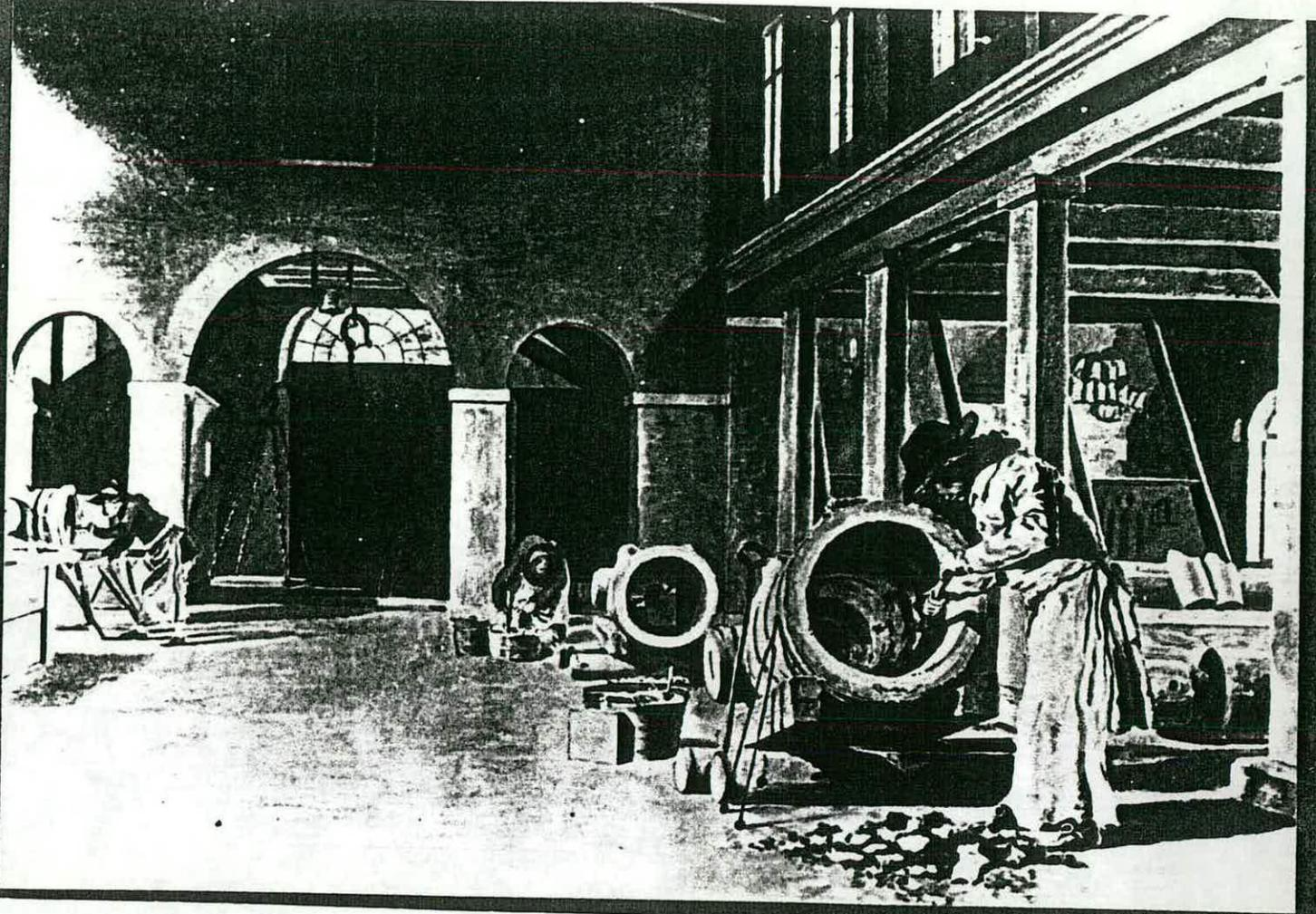
15. The final stage of clearing the pattern from the mould - the clay is being removed.
