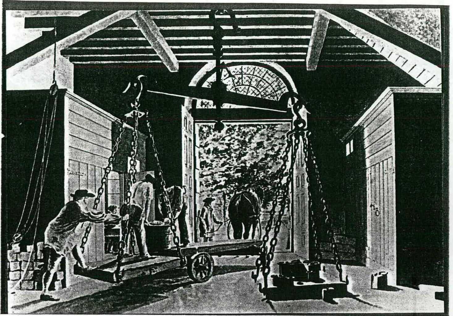
1. View from the vestibule of the Royal Foundry looking north-east towards the Thames. Note the large beam scale which was an essential piece of equipment, not only to measure the ingredients of the melt, but also to weigh the finished ordnance and to determine its Centre of Gravity.
