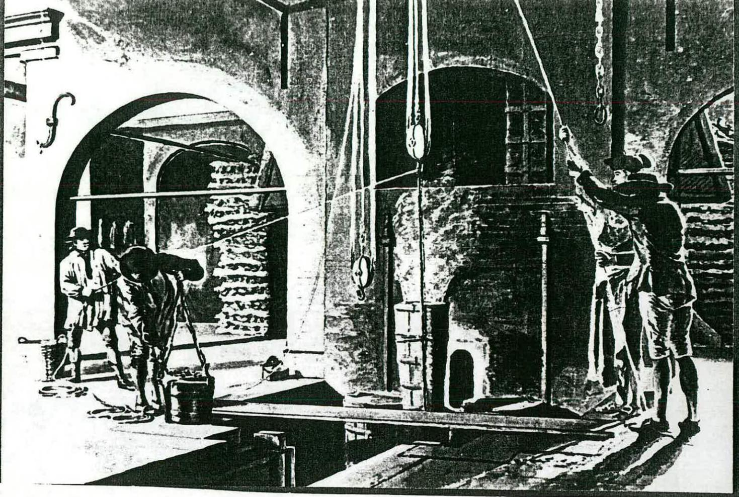
30. The worker on the left is rigging iron strapping above the cascabel mould of a small-calibre gun.
