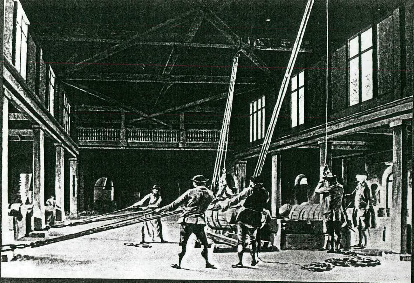
11. A completed mould is being lifted off its turning frame for removal of the pattern.
