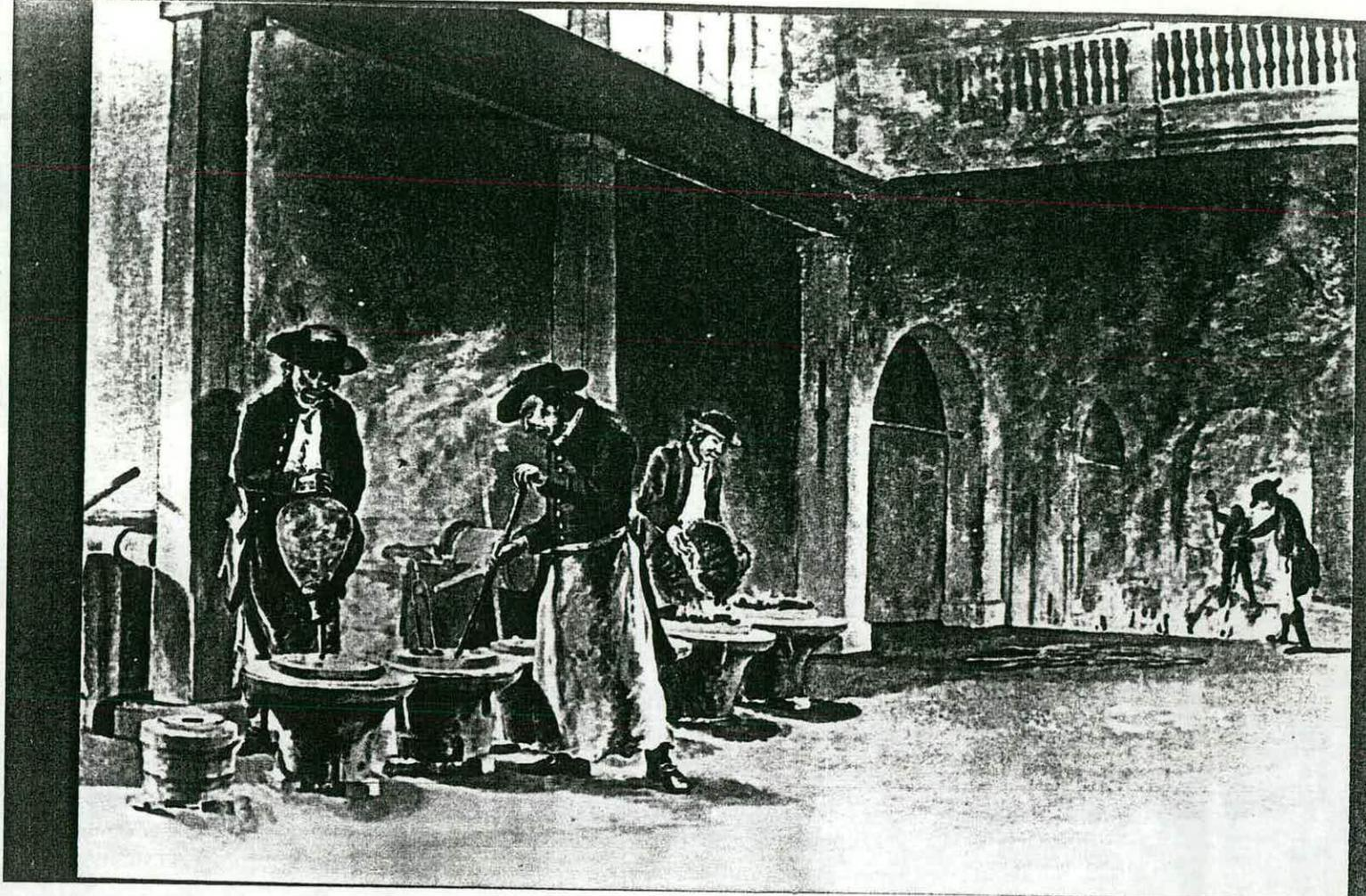
27. Seven cascabel moulds are being baked on the left. A charcoal fire burns within as well as under the moulds.
