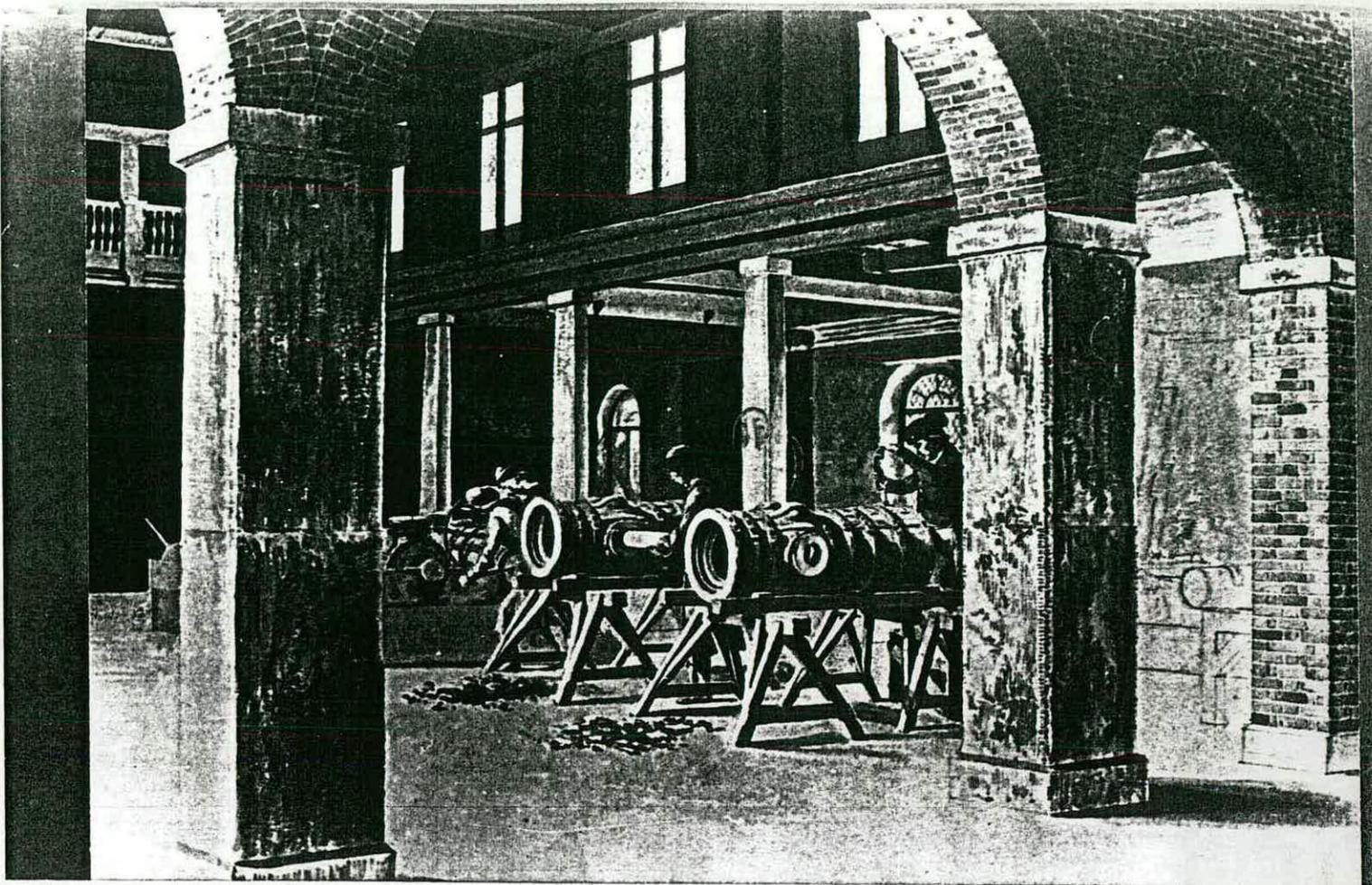
16. Two small howitzers are shown that have been cleared of their patterns. The worker in the middle is smoothing and gauging the trunnion holes whilst the man on the right is drilling a Sprue hole, eg a vent for the air to escape when molten metal is poured in and so reduce the risk of blow holes.
