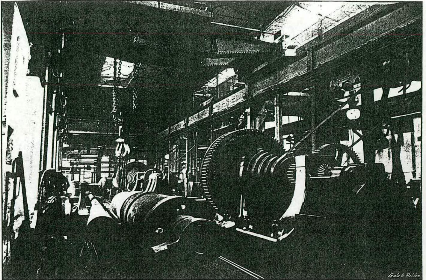
HEAVY TURNERY DEPARTMENT ROYAL GUN FACTORY, SHEWING A 12-in. OR 50-TON GUN BEING HOISTED IN A LATHE, PREPARATORY TO BEING TURNED.
