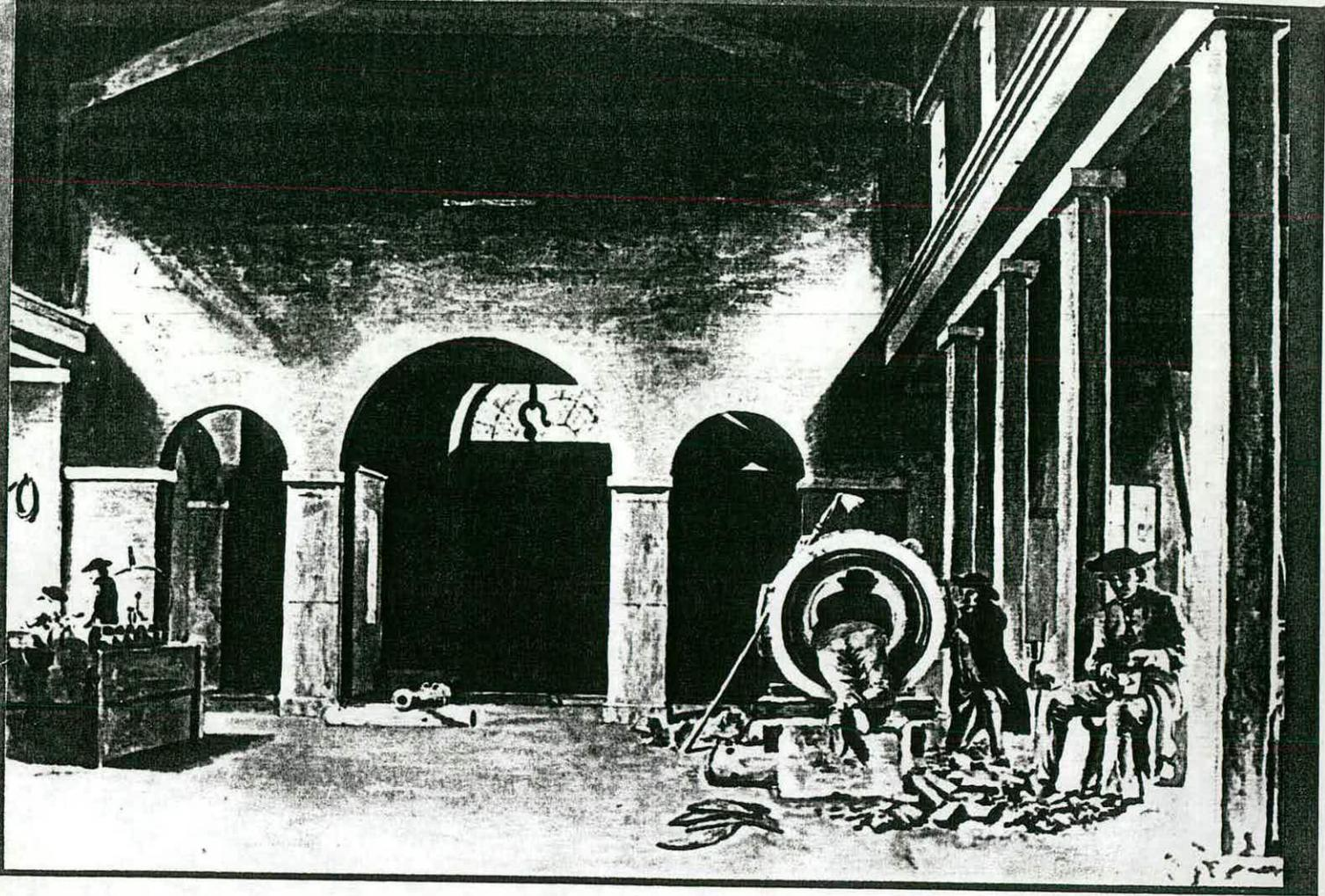
23. The mould being cleared of its brick armature and clay model. Bore and trunnion holes are being examined for flaws by the light of a candle.
