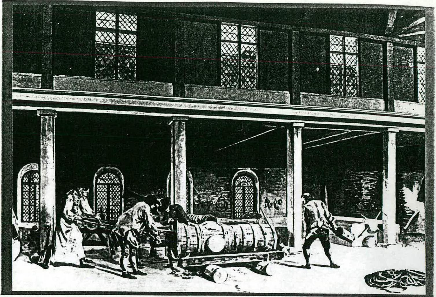
12. The clay model is ready to be disengaged from the mould. The worker has clouted the greased tapered wooden spindle, freeing it. The workers on the left are carefully withdrawing it.
