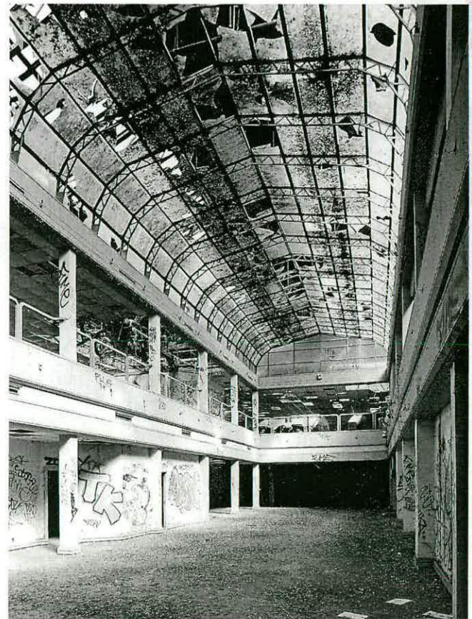
Fig 8 - Atrium inserted within the original structure of the former 'Liberal Arts Palace'.
