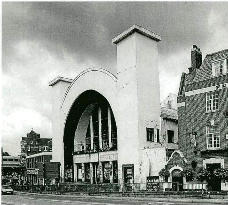
Fig 5 - The White City Arch as it looked in 2001, from the southeast.
