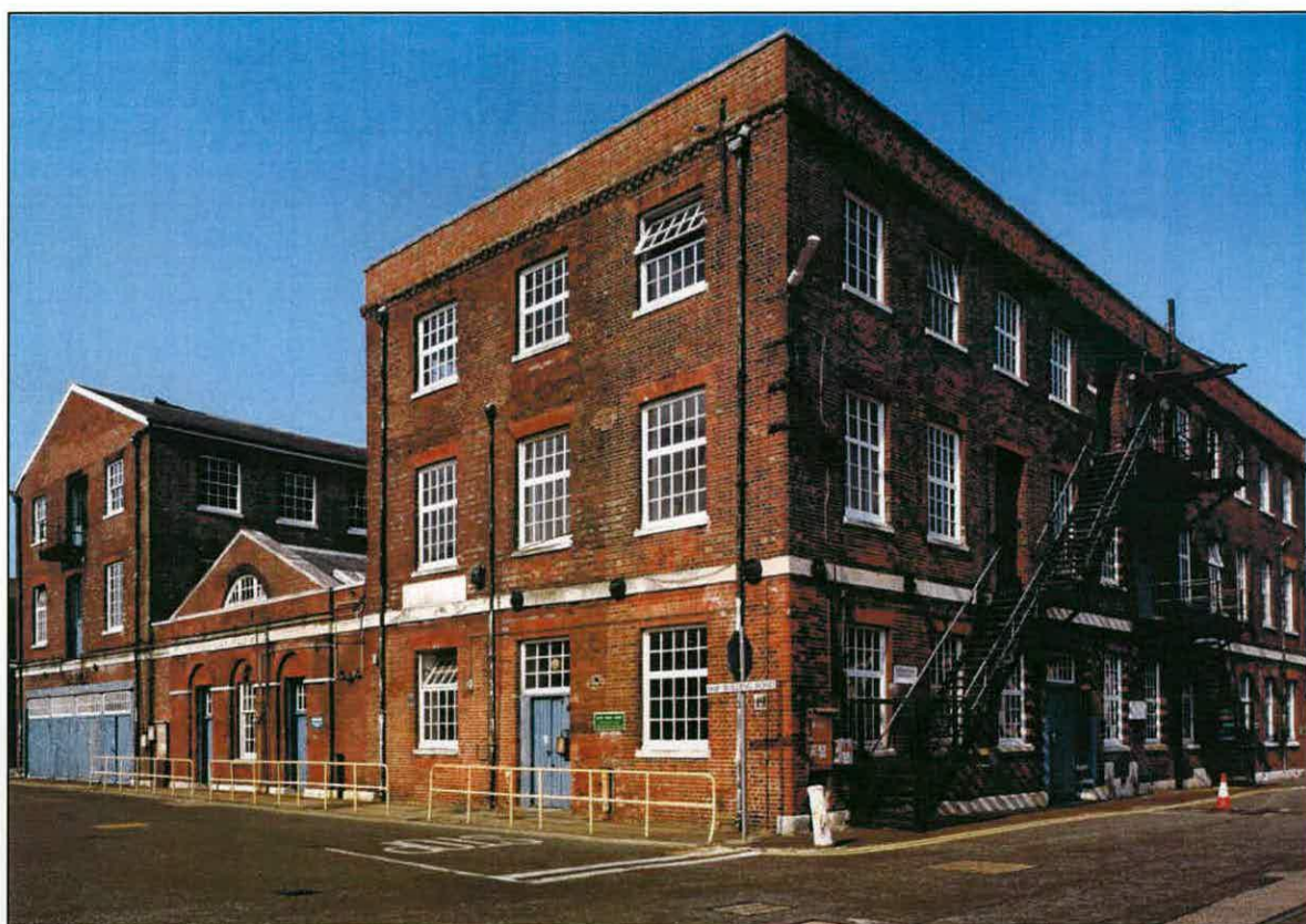
Figure 1. The Block Mills from the south west, 2003. [AA042456]
