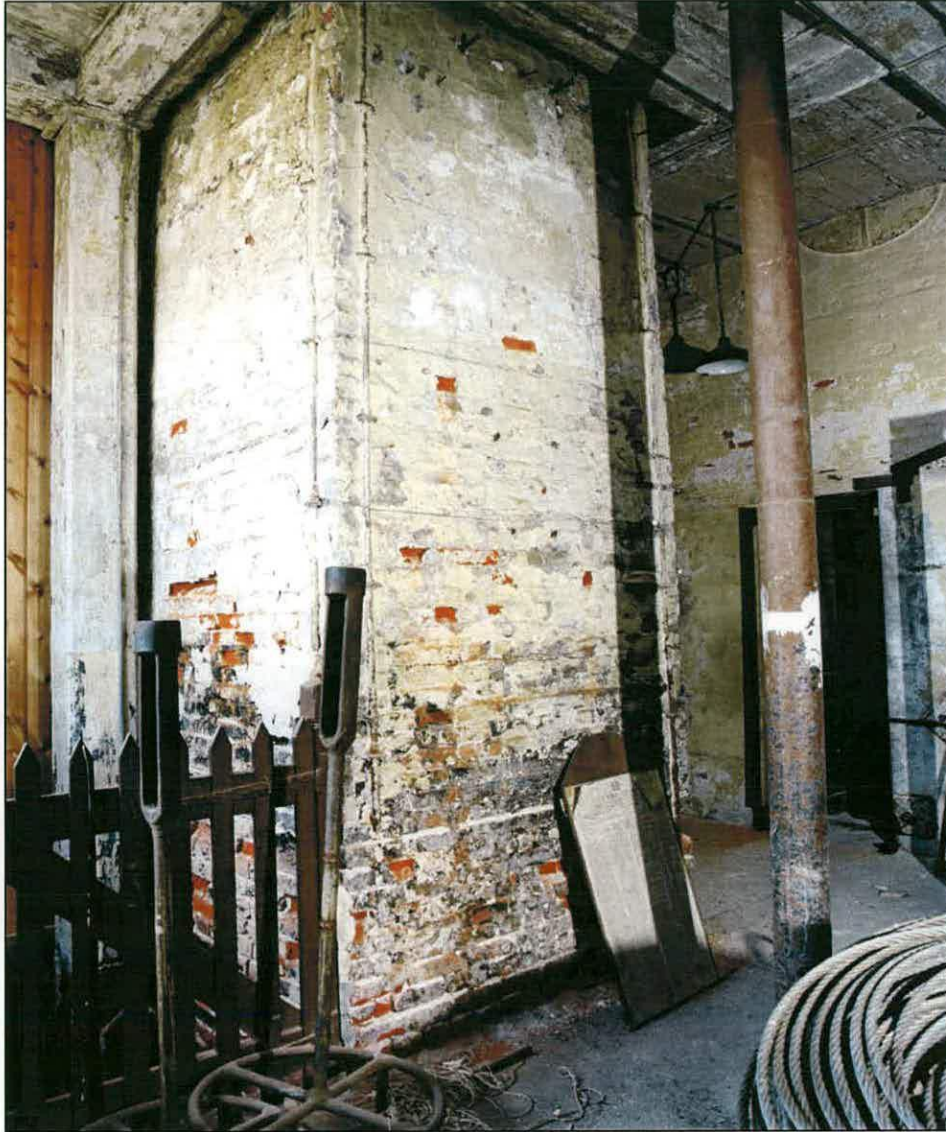
Figure 6. The base of the surviving chimney of the western boiler house in the south range of the wood mills. A photograph taken in 2003. [AA042389]
