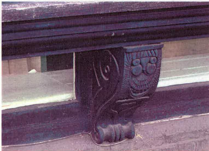
Figure 6 Carved timber bracket supporting projecting front ground floor window of north cross wing of main house.
