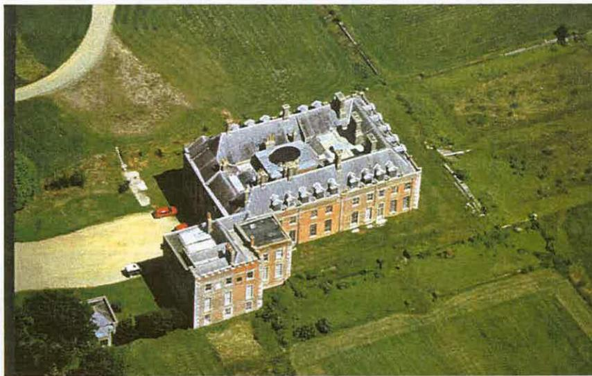
**Figure 27. View of the house from the south west. Note the flat roofs over the Stone Hall and, to the east of that, the Great Stair**
