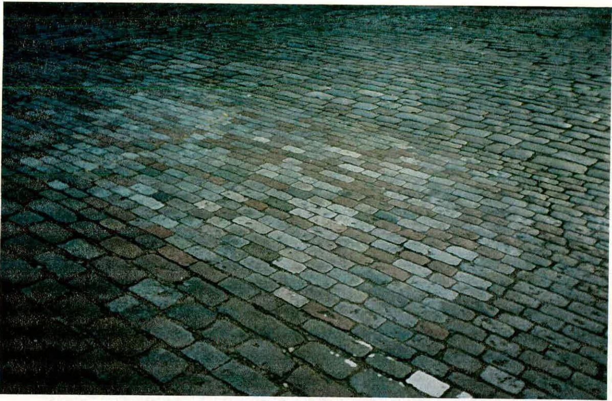
17 Charterhouse Square. North-west corner, showing crossing 2000
